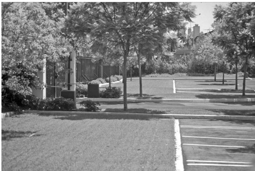
FIGURE 8.15 Grassroad overflow parking spaces at California JPIA in La Palma, California.
