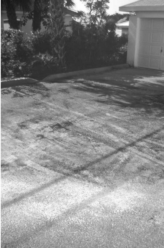
FIGURE 2.23 Sediment on a porous concrete parking area surrounded by raised curbs at an office building in Hobe Sound, Florida.
