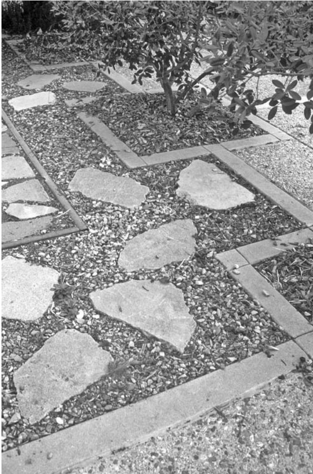
FIGURE 9.30 Plaza of recycled concrete rubble at the Lyle Center for Regenerative Studies in Pomona, California.
