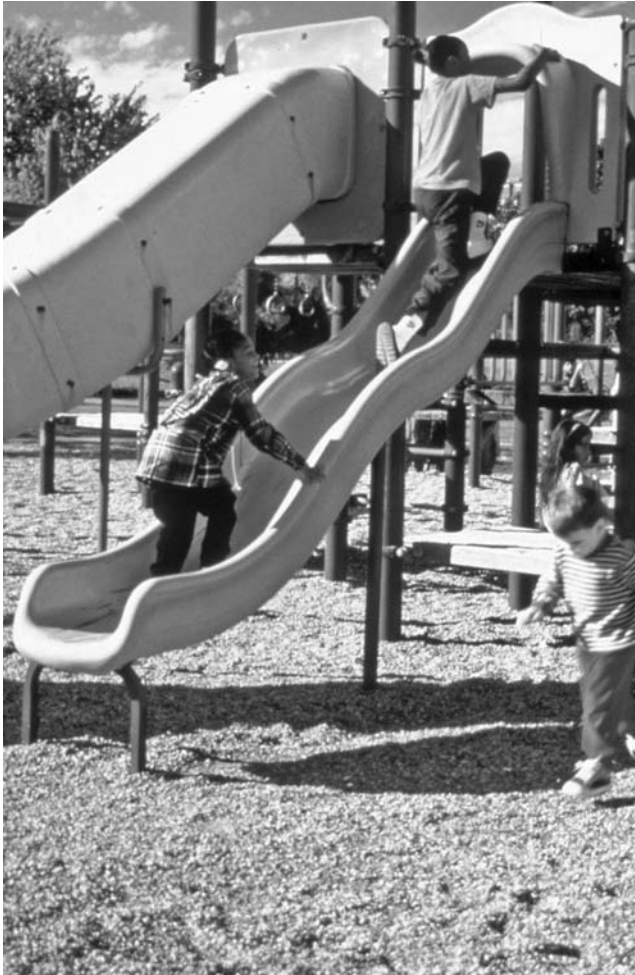
FIGURE 6.19 Playground surface of rounded aggregate in Vandergrift Park, Arlington, Texas.
