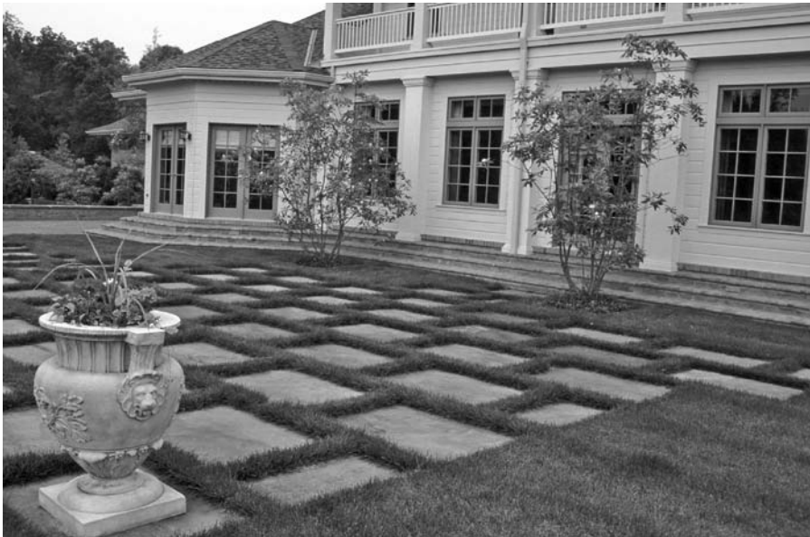
FIGURE 9.29 Widely spaced concrete slabs with turf joints at a residence in St. Clairsville, Ohio.
