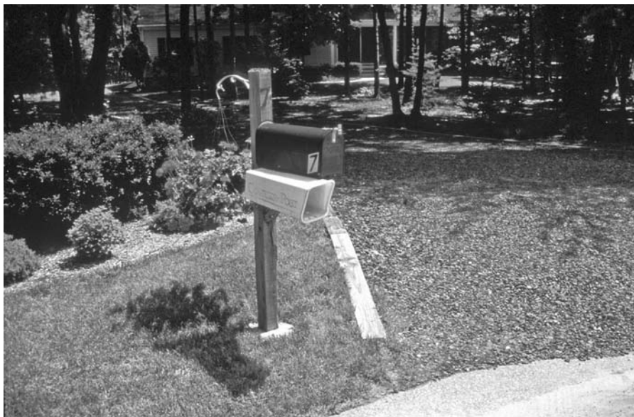
FIGURE 6.10 Aggregate driveway at a residence in Medford Township, New Jersey, about four years after installation.
