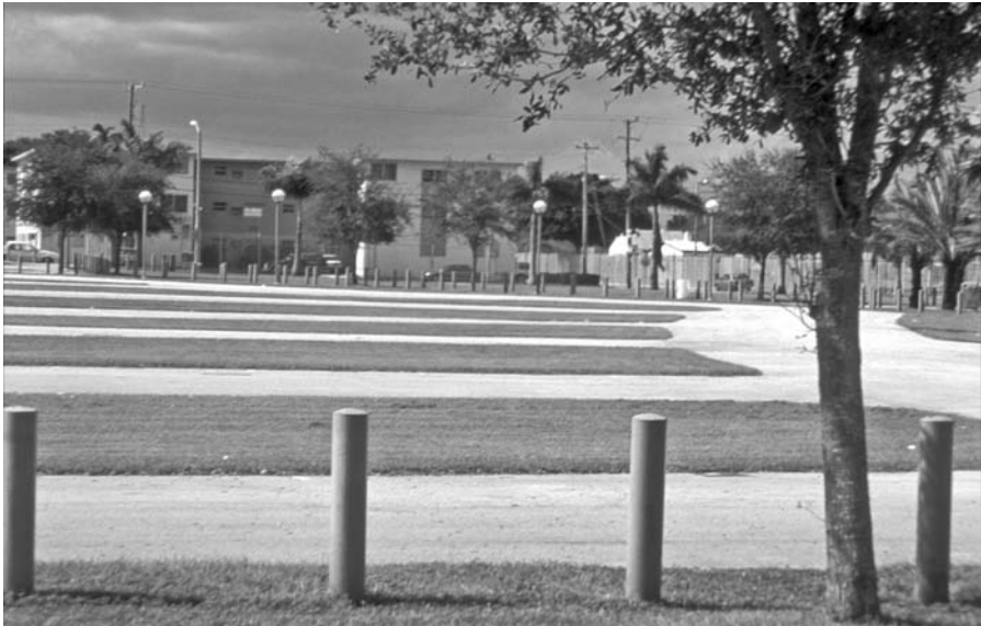
FIGURE 8.8 Grasspave 2 parking at the Orange Bowl, six years after installation and five days after heavy use during a college football game.
