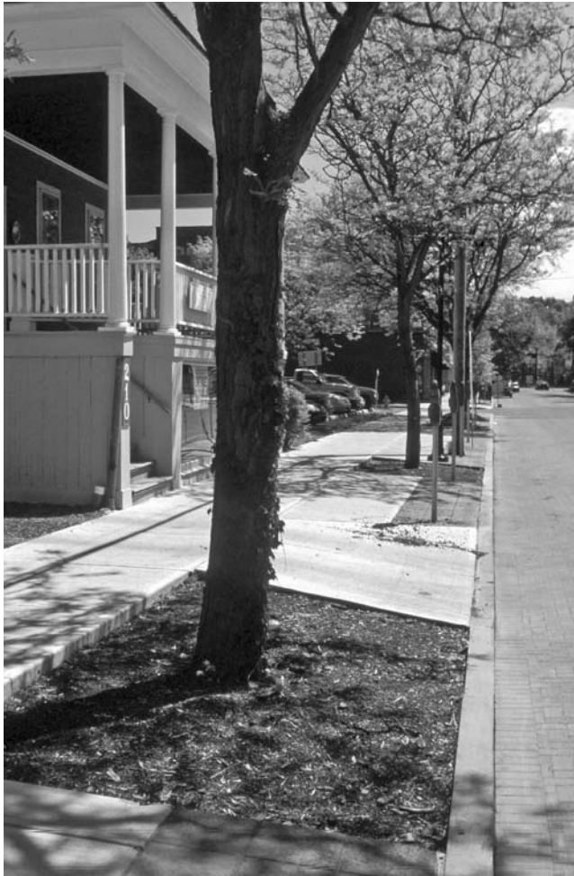
FIGURE 5.4 Trees rooted in Cornell structural soil on State Street in Ithaca, New York.
