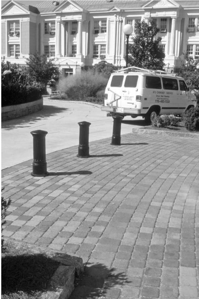
FIGURE 3.29 Metal bollards confining vehicles to a concrete pavement and away from a pedestrian block pavement.
