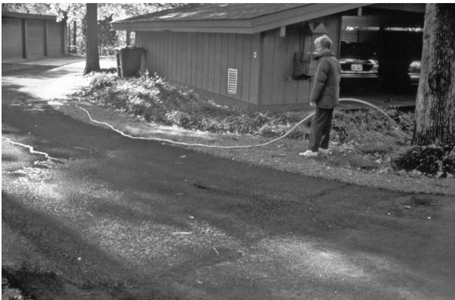
FIGURE 12.1 A porous asphalt residential driveway near Macon, Georgia, in 1996.
