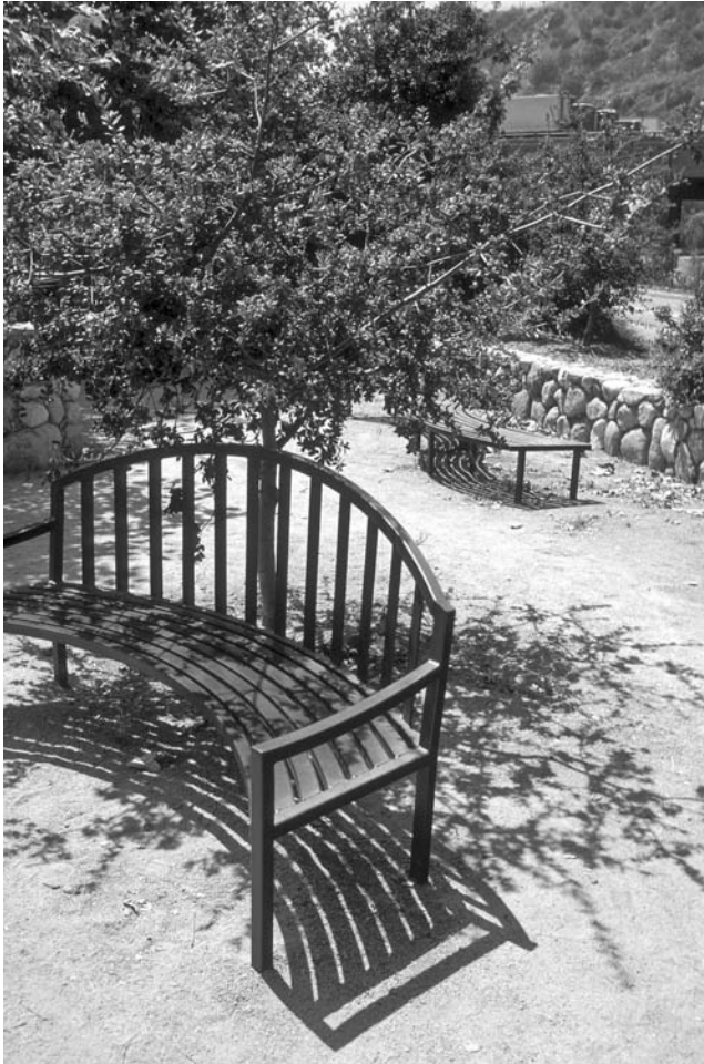
FIGURE 6.9 Pedestrian area of decomposed granite partly stabilized with Stabilizer, Steelhead Park, Los Angeles, about one year after installation.
