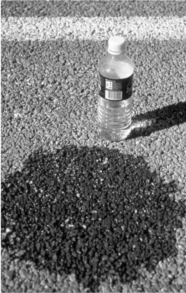
FIGURE 1.9 Infiltration into the surface of the porous concrete parking lot at the Florida Aquarium in Tampa, Florida.
