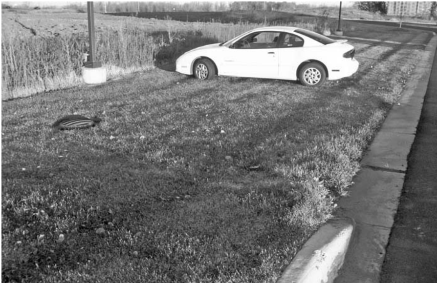
FIGURE 7.14 Mesh-reinforced turf parking at Lino Lakes State Bank in Lino Lakes, Minnesota, in November 2002.
