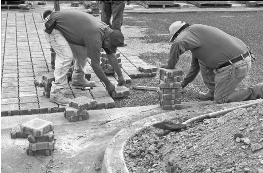
FIGURE 9.26 SF-Rima being laid on a bedding layer of No. 8 aggregate.
