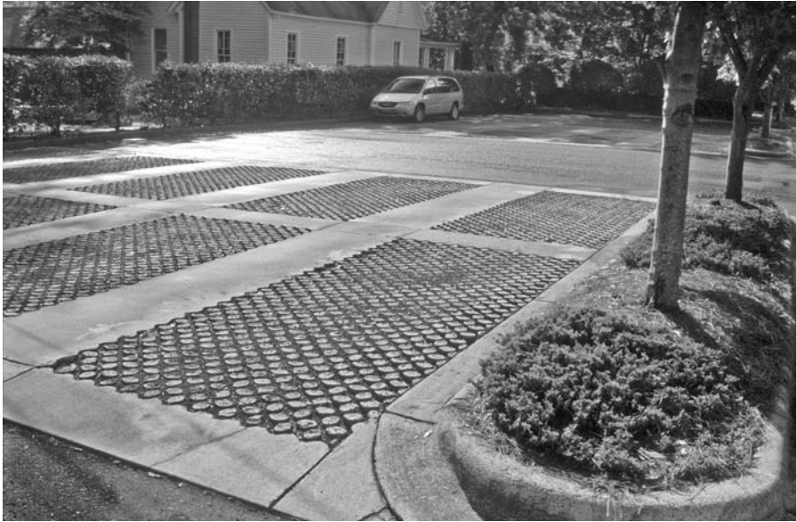
FIGURE 10.11 Parking spaces of Grasscrete with crushed-brick aggregate at the office of David Furman Architecture in Charlotte, North Carolina.
