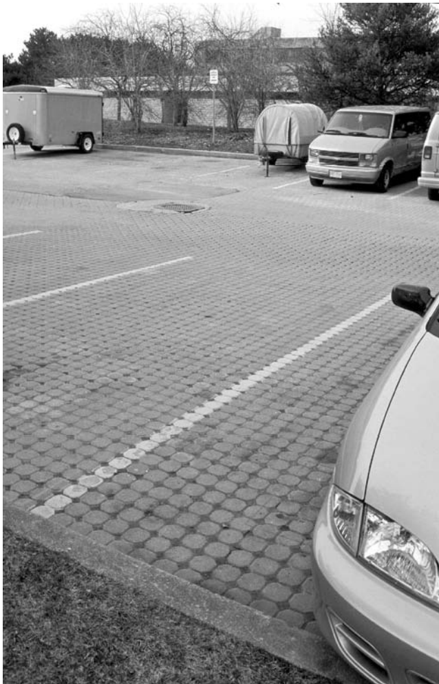
FIGURE 3.17 Porous pavement of open-jointed Eco-Stone blocks at the Thornbrough Building at the University of Guelph, Guelph, Ontario.
