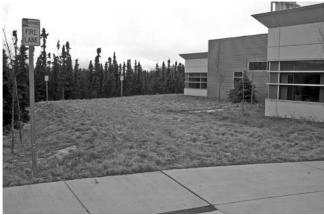
FIGURE 8.3 Geoblock emergency access lane at the Alaska Department of Health and Social Services Public Health Laboratory, Anchorage, in 2003.
