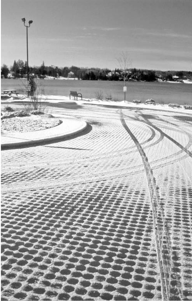
FIGURE 3.18 Porous pavement of open-jointed Eco-Stone blocks at Sunset Beach Park, Richmond Hill, Ontario.
