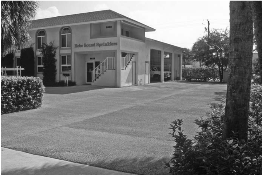
FIGURE 11.12 Porous concrete parking lot at Hobe Sound Sprinklers in Hobe Sound, Florida.
