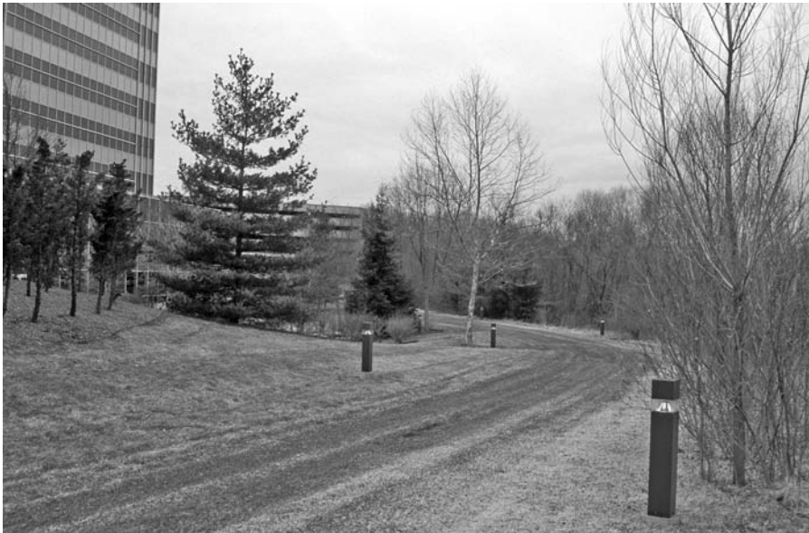
FIGURE 8.12 Grasspave 2 emergency access lane at Blue Cross Blue Shield of Michigan, Southfield, Michigan.
