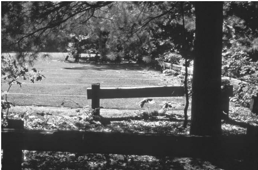
FIGURE 12.19 Porous asphalt parking lot at Walden Pond State Reservation, Massachusetts, in 1999.
