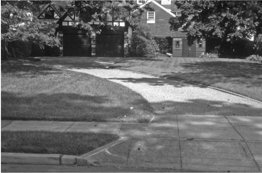
FIGURE 6.11 A residential driveway in Garden City, New York.
