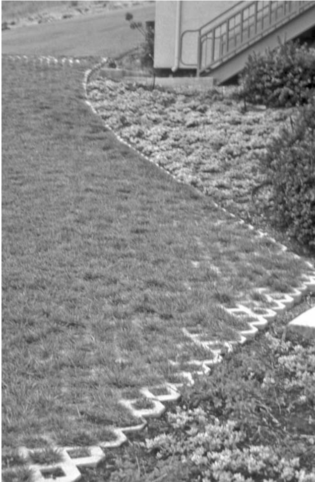
FIGURE 10.19 Turfstone emergency access lane at the San Luis Bay Inn in Avila Beach, California.
