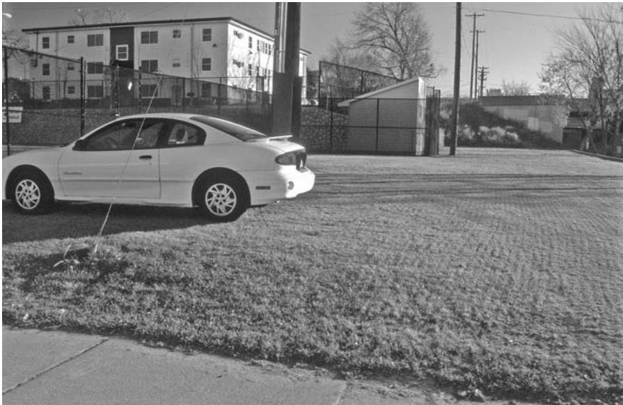
FIGURE 7.16 Mesh-reinforced turf parking at the Urban Ventures soccer field in Minneapolis, in November 2002.
