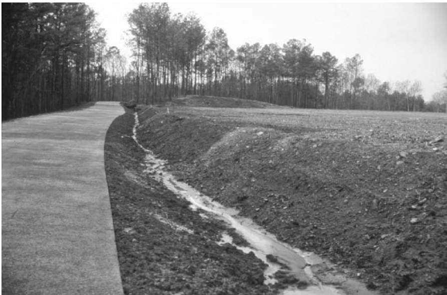
FIGURE 2.22 Edge of a porous concrete road in Webb Bridge Park, Alpharetta, Georgia, in 1998.
