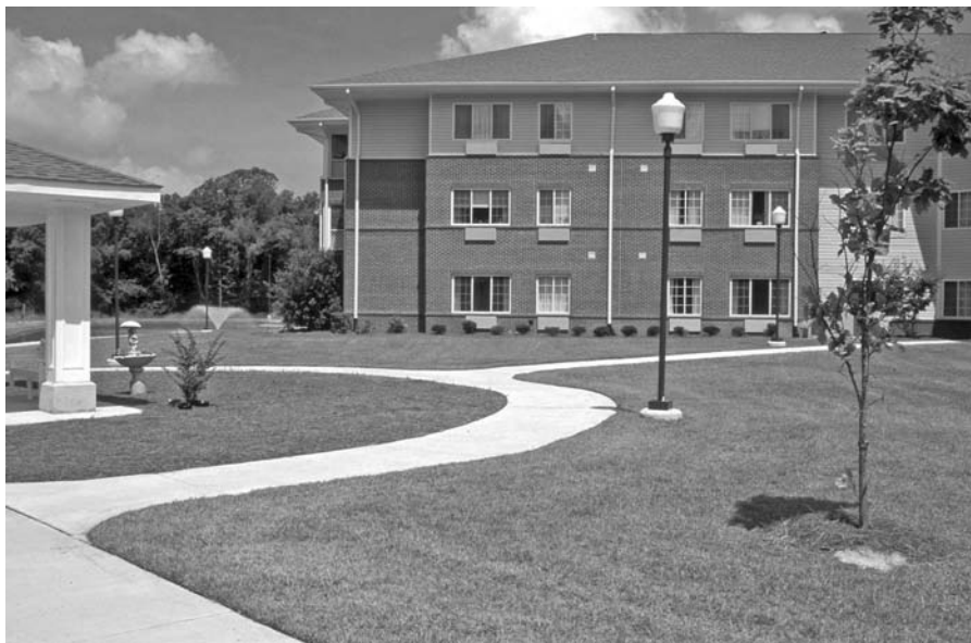
FIGURE 8.11 Emergency access lane at Trace Pointe Retirement Community, Clinton, Mississippi.
