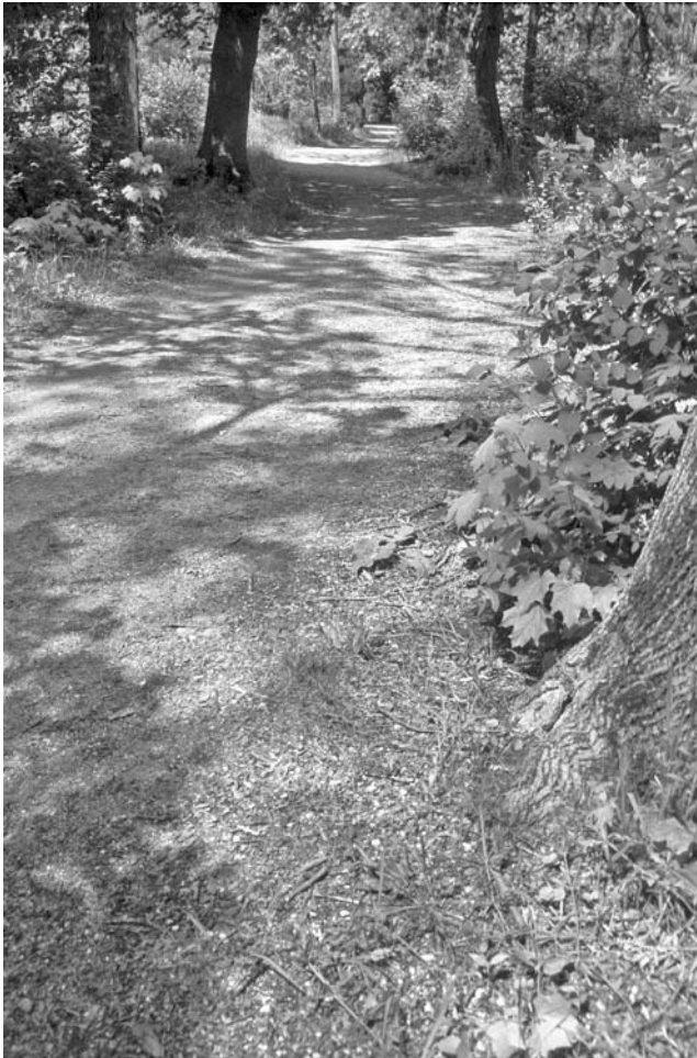
FIGURE 6.6 Stabilized aggregate trail in Minuteman National Park, Concord, Massachusetts.
