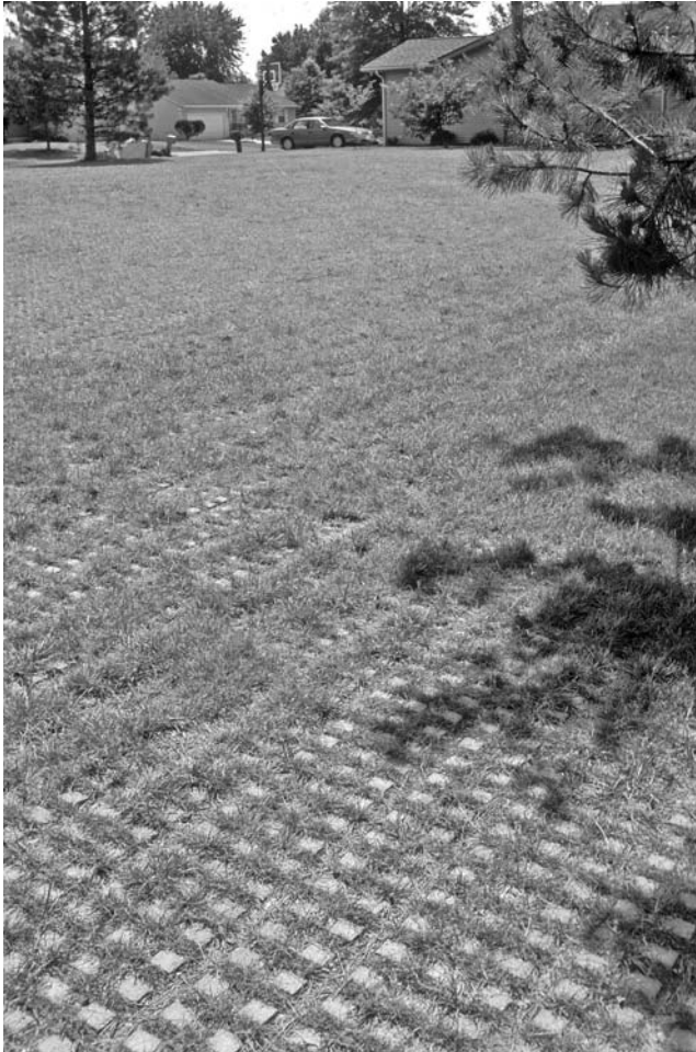
FIGURE 10.15 Monoslab area for weekly parking at the Christian Meeting Room, Gahanna, Ohio.
