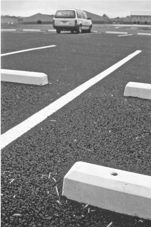
FIGURE 12.11 The porous asphalt parking lot in Roswell, Georgia's Sweet Apple Park.
