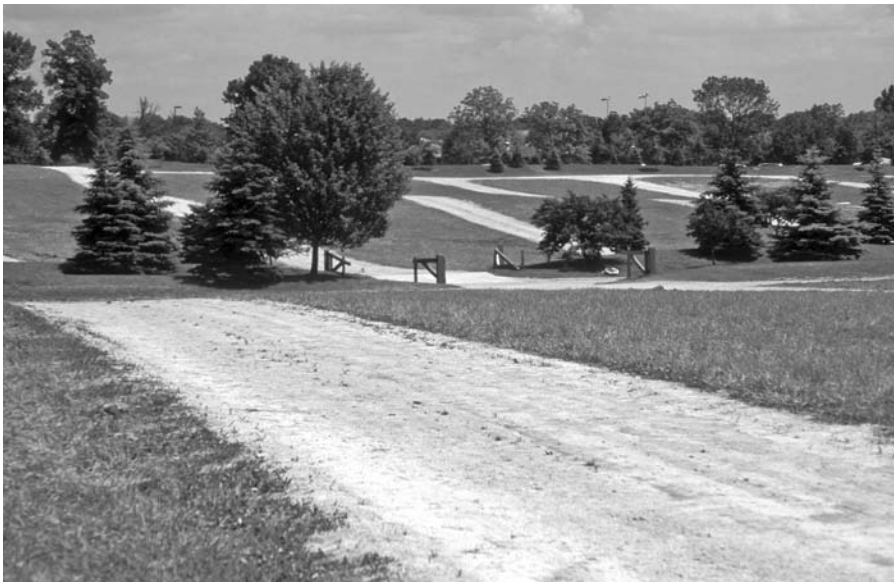
FIGURE 7.12 Parking field at Muirfield Village in Dublin, Ohio.
