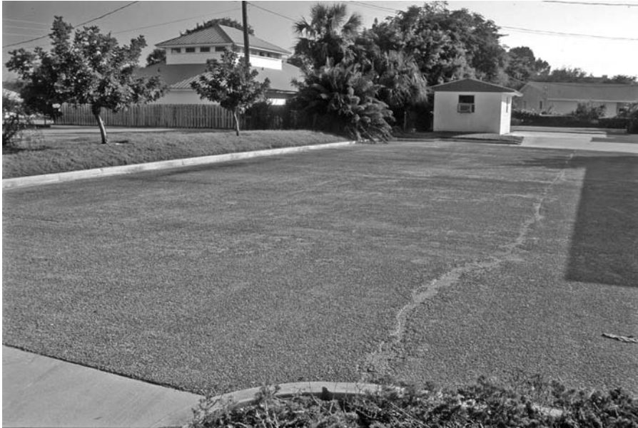
FIGURE 11.11 Porous concrete parking lot at another medical office in Stuart, Florida.
