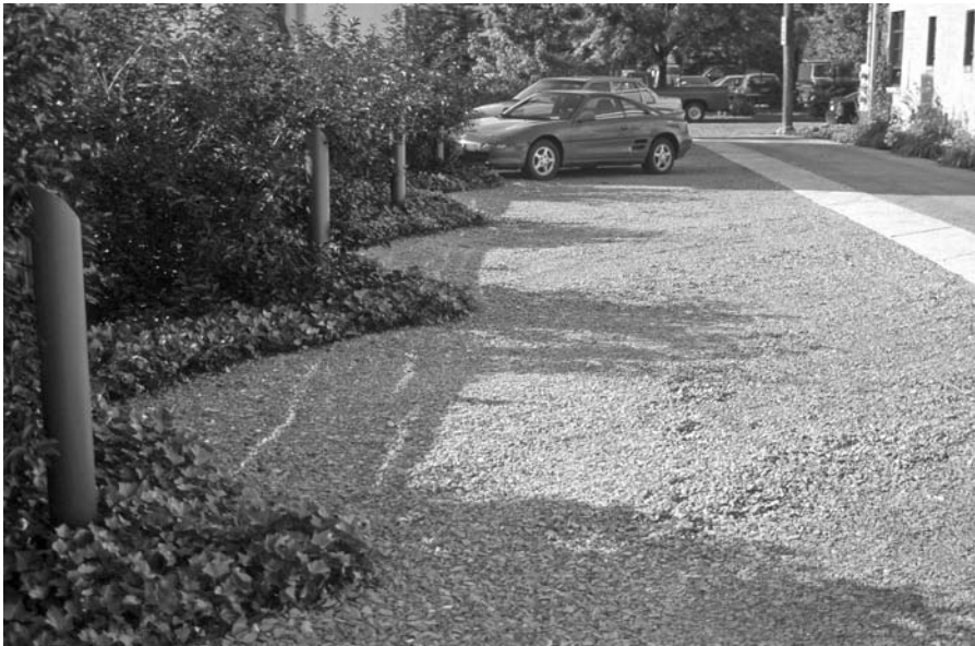
FIGURE 6.13 Parking stalls of crushed vitrified clay at Lincoln Street Studio, Columbus, Ohio.
