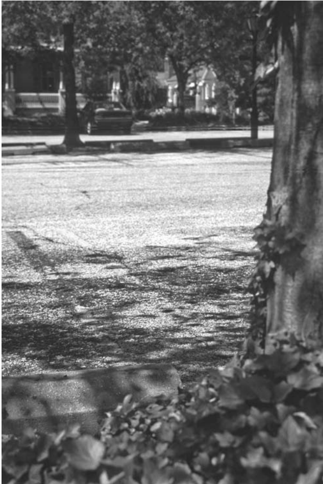
FIGURE 12.3 The University of Delaware porous asphalt parking lot in 1996.
