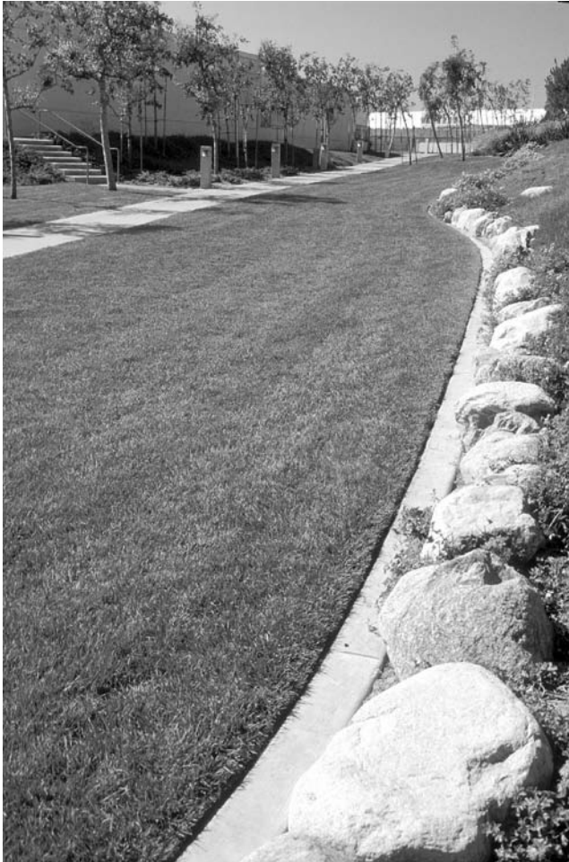
FIGURE 1.22 Emergency access lane of grass reinforced by concrete grids at the Saddleback Church in Lake Forest, California.
