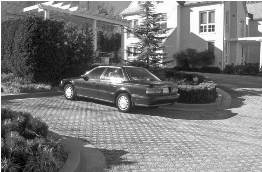
FIGURE 10.23 Turfstone with gravel fill at the Blue Heron residential community in Annapolis, Maryland.
