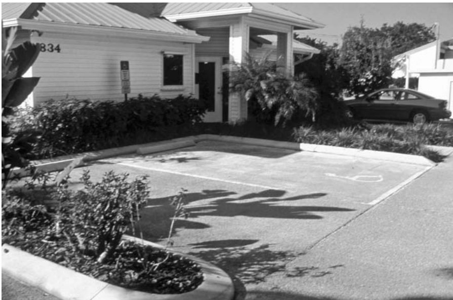
FIGURE 11.10 Porous concrete parking lot at a medical office in Stuart, Florida.
