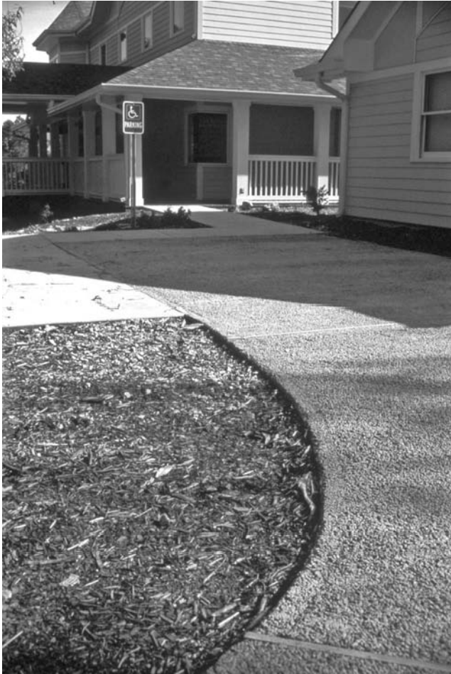
FIGURE 11.15 Porous concrete driveway at the Southface Institute in Atlanta, Georgia.
