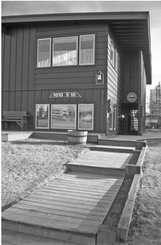
FIGURE 14.4 On-grade boardwalk in Anchorage, Alaska.
