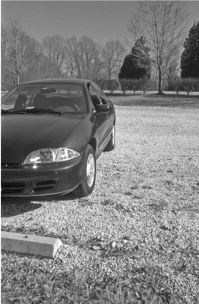
FIGURE 6.12 Aggregate parking lot in Quiet Waters Park, Annapolis, Maryland, ten years after installation.
