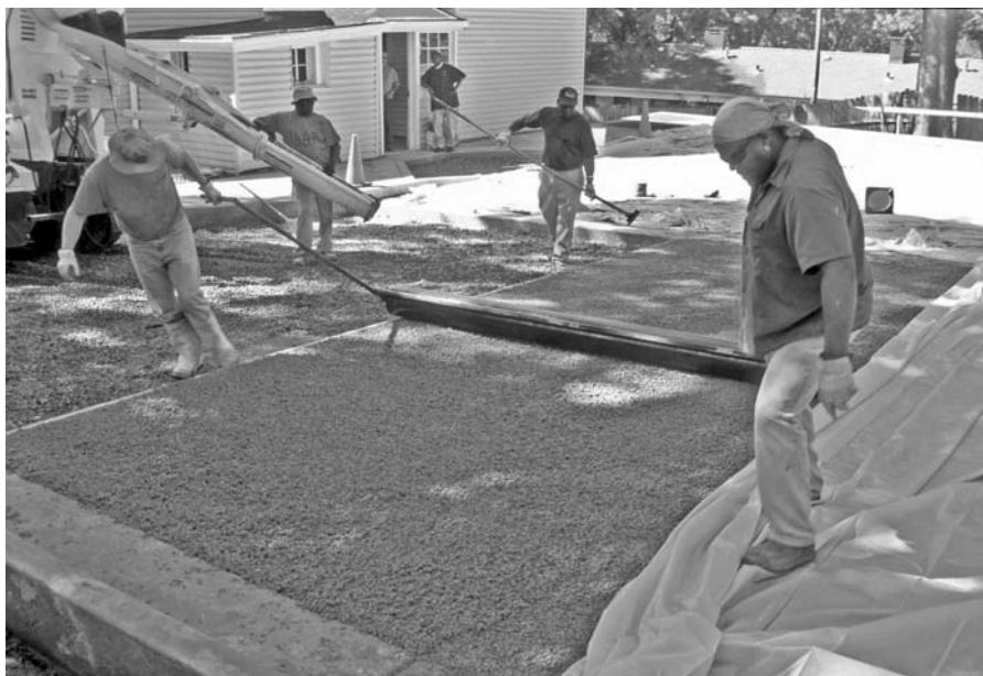
FIGURE 11.9 Rolling porous concrete to level.
