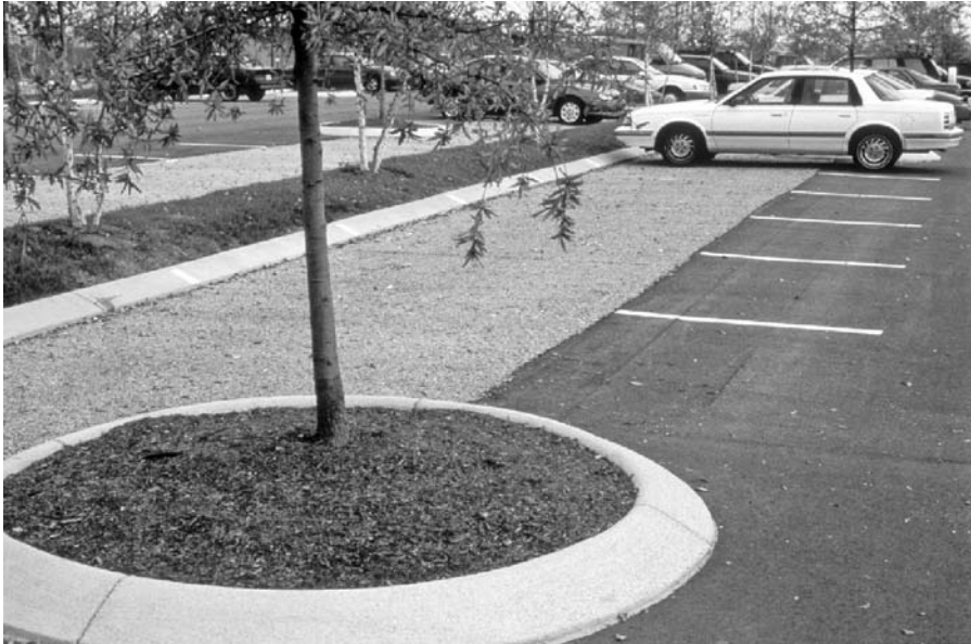
FIGURE 2.13 Porous concrete parking stalls at Finley Stadium in Chattanooga, Tennessee.
