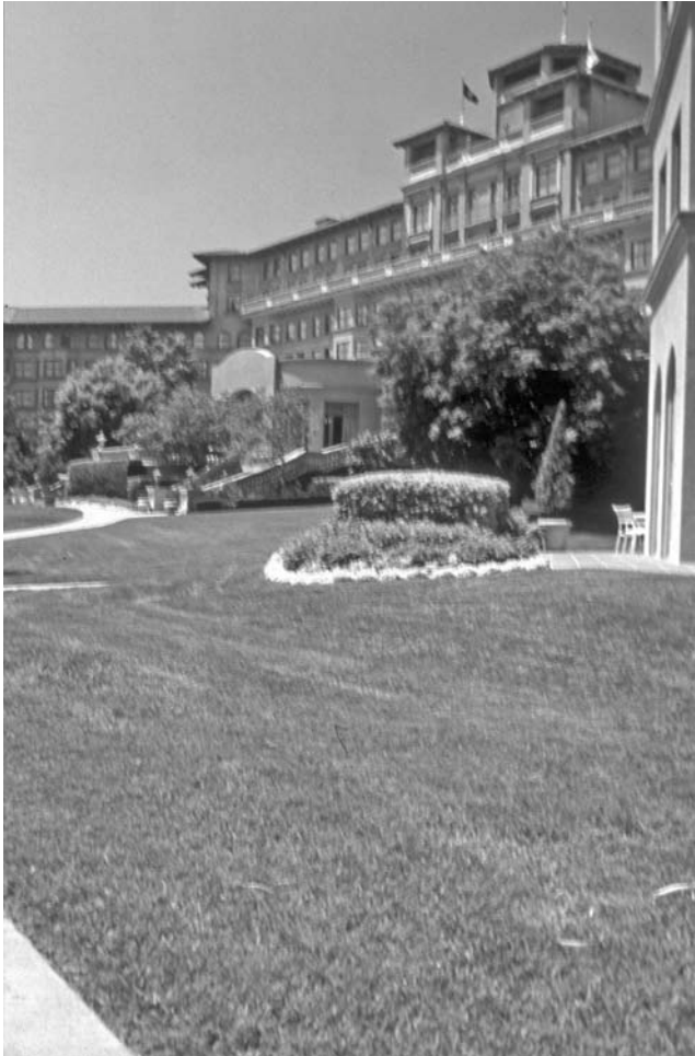
FIGURE 8.2 Geoblock emergency access lane at the Ritz-Carlton Huntington Hotel in Pasadena, California.
