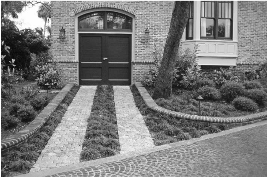
FIGURE 1.5 A residential driveway reduced to two wheel tracks.
