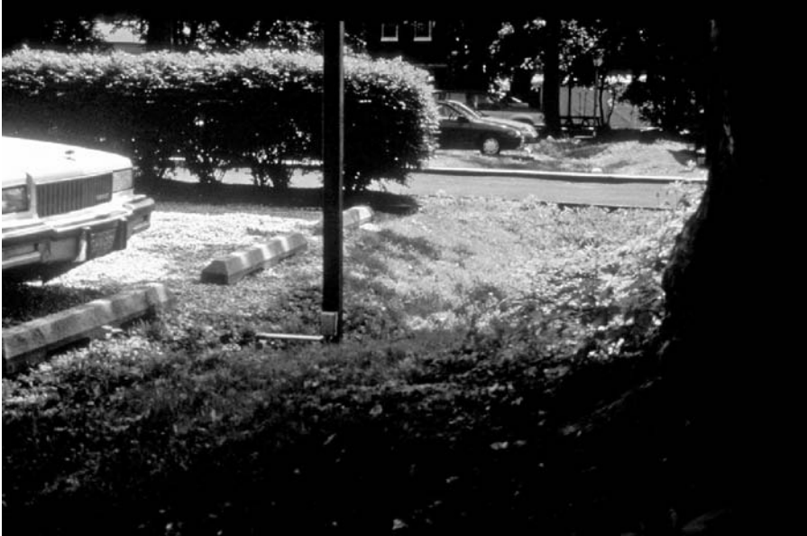
FIGURE 2.18 A vegetated swale draining aggregate parking stalls in Medford Village, New Jersey.
