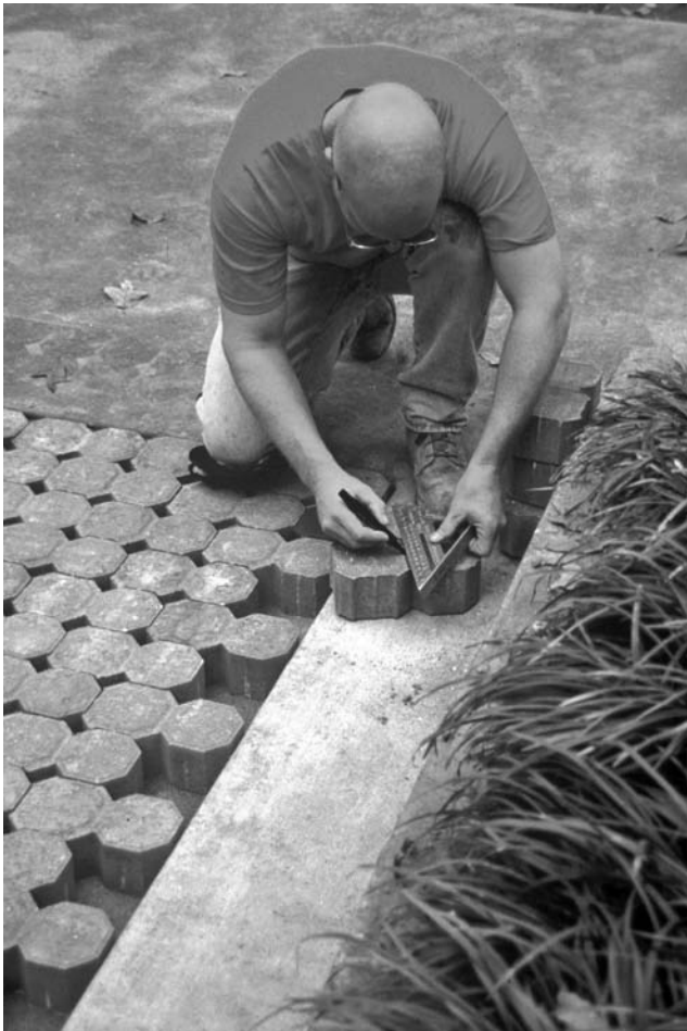
FIGURE 9.19 Eco-Stone being placed in a parking bay.
