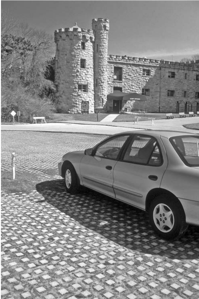
FIGURE 10.8 Checkerblock parking field at the Sands Point Museum on Long Island, New York.
