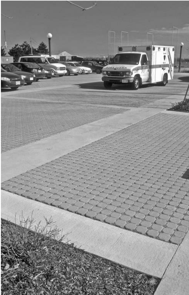
FIGURE 9.23 Eco-Stone drive at Harbourfront Fire Station, Toronto.
