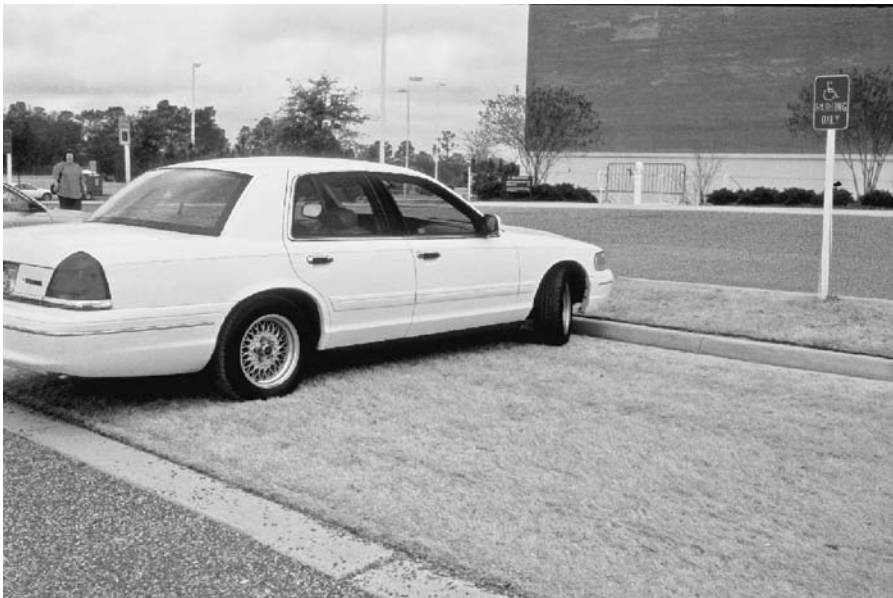
FIGURE 2.21 Parking bay of turf reinforced with plastic geocells at Mitchell Center Arena, University of South Alabama, Mobile, Alabama.
