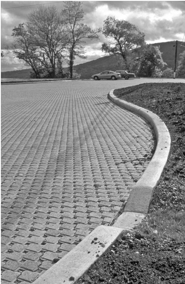
FIGURE 9.15 Ecoloc parking lot at Annsville Creek Paddlesports Center, Cortland, New York.
