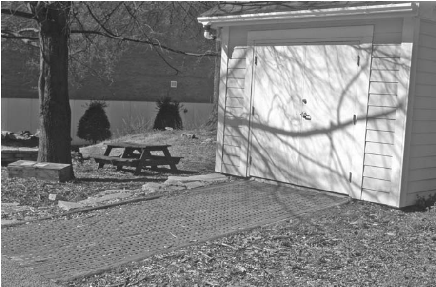
FIGURE 10.24 Cored brick used as an open-celled paving grid at the Southface Institute, Atlanta, Georgia ( www.southface.org ).
