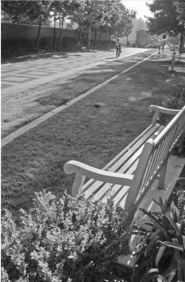
FIGURE 10.10 Grasscrete emergency access lane at the Anderson School of Management, University of California, Los Angeles.
