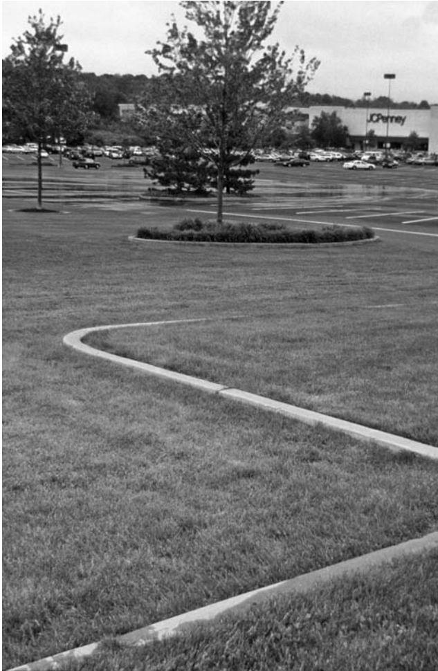
FIGURE 8.9 Grasspave 2 overflow parking at Westfarms Mall in Farmington, Connecticut, in 2002.
