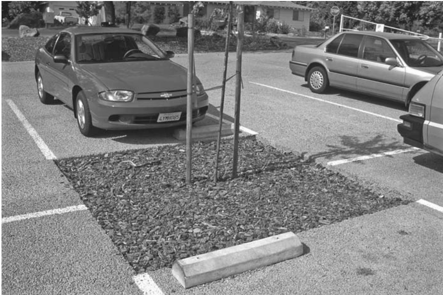
FIGURE 11.17 Porous concrete parking lot at Bannister Park in Fair Oaks, California.
