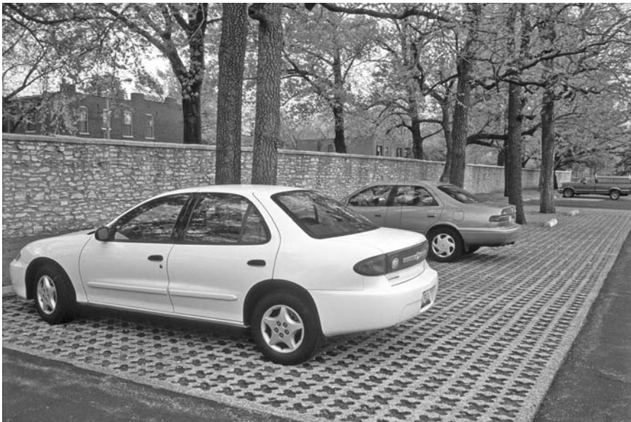
FIGURE 10.12 Grasscrete (old configuration) parking bays over the rooting zones of persimmon trees at the Missouri Botanical Garden, Saint Louis.
