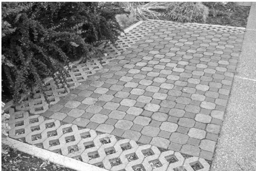
FIGURE 2.12 Concrete open-celled grid draining the edge of a courtyard pavement at Olympia City Hall in Olympia, Washington.
