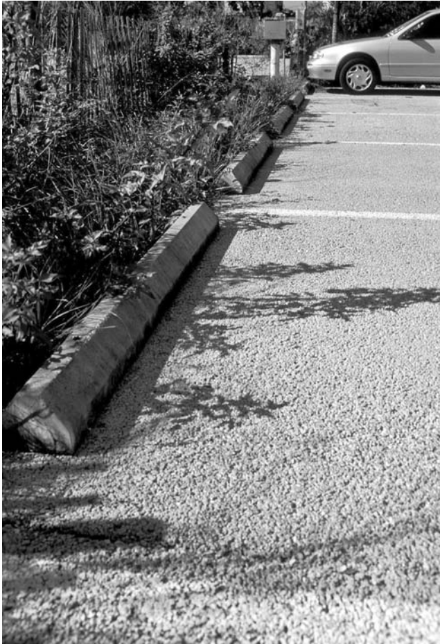
FIGURE 11.1 Porous concrete parking stalls and vegetated swale at the Florida Aquarium in Tampa, Florida.
