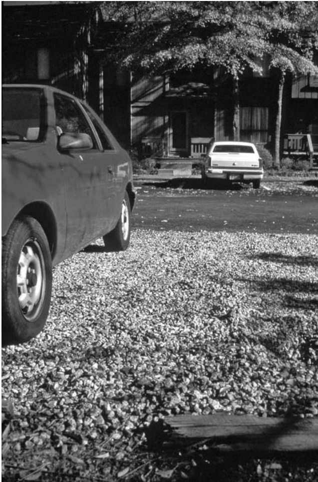
FIGURE 6.14 A retrofit parking expansion of unbound aggregate in the Riverbend East residential condominium in Athens, Georgia.
