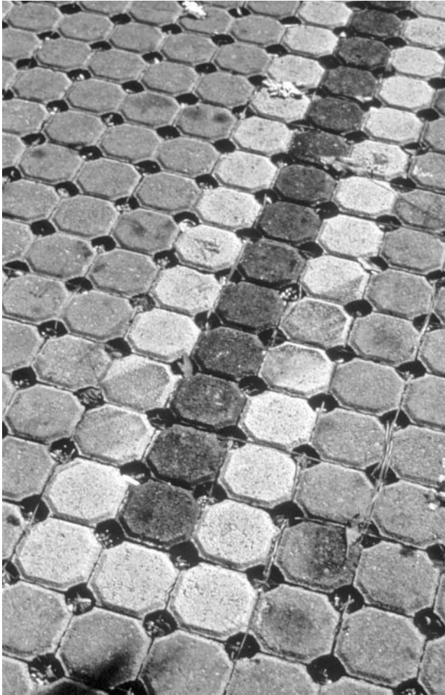
FIGURE 9.11 Painted dividing lines aligned with Drainstone paving blocks at English Park, Atlanta, Georgia.
