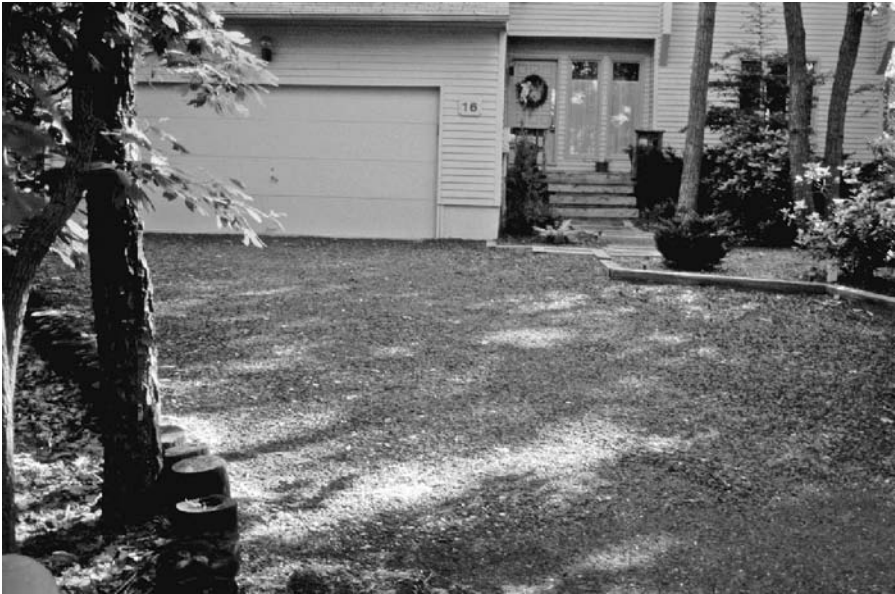
FIGURE 2.19 Porous aggregate driveway in the Cardinal Ridge residential community in Medford, New Jersey.
