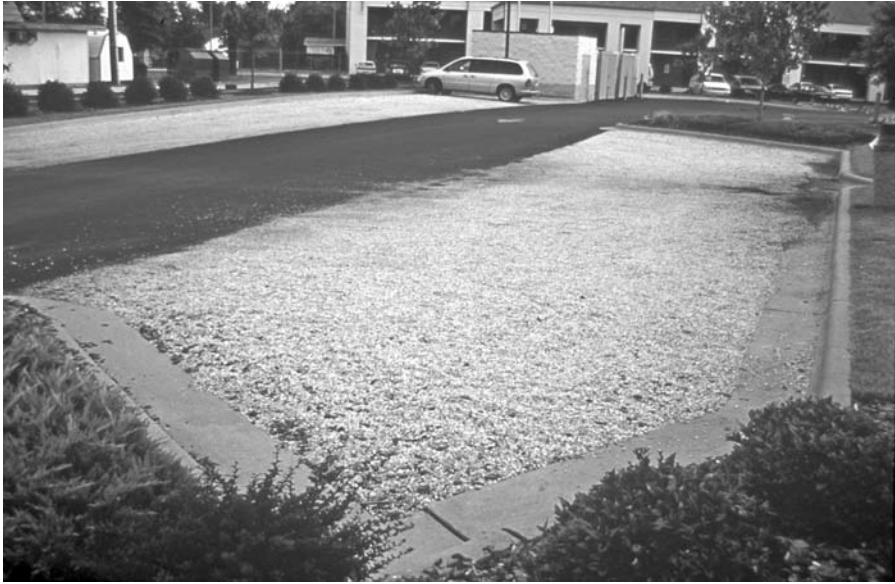
FIGURE 8.18 Gravelpave 2 parking at a Burger King restaurant in Henderson, North Carolina.
