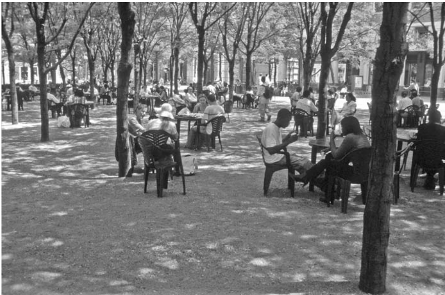
FIGURE 1.12 Large, healthy honey locust trees rooted in "structural soil" beneath a porous aggregate pavement in the Metrotech Business Improvement District in Brooklyn, New York, 14 years after installation.
