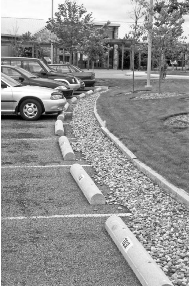
FIGURE 2.14 Porous asphalt parking lot at the Centre County-Penn State Visitor Center in State College, Pennsylvania.
