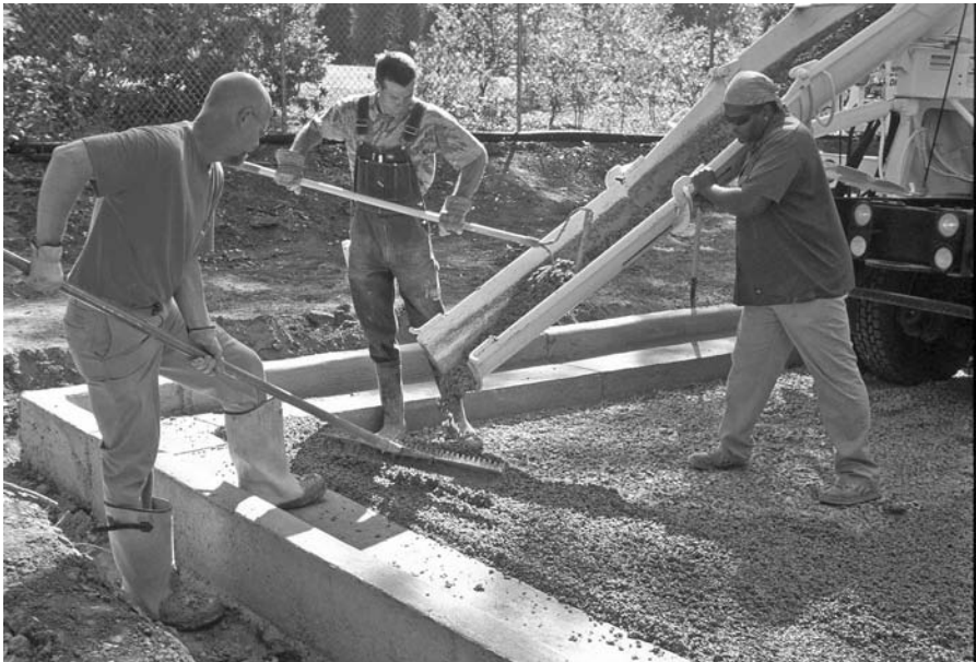
FIGURE 11.8 Placing wet porous concrete.
