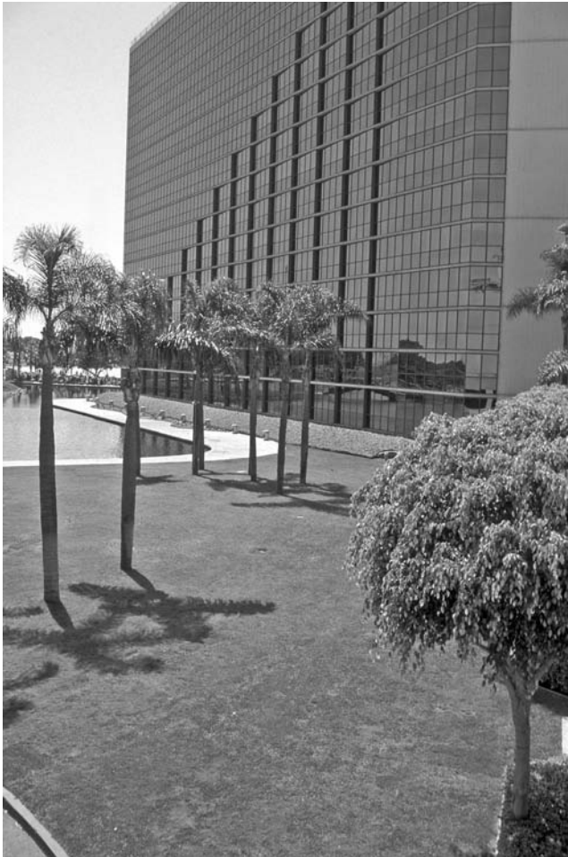
FIGURE 8.14 Grassroad emergency access lane at the Hyatt Regency Hotel in Long Beach, California.
