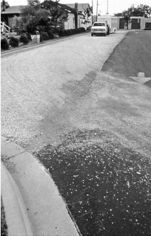
FIGURE 8.19 Displacement of rounded gravel by moving vehicles at the Henderson Burger King.
