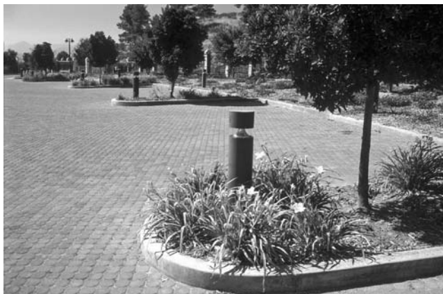
FIGURE 9.22 Eco-Stone parking lot at the Castaic Lake Water Conservatory in Santa Clarita, California.
