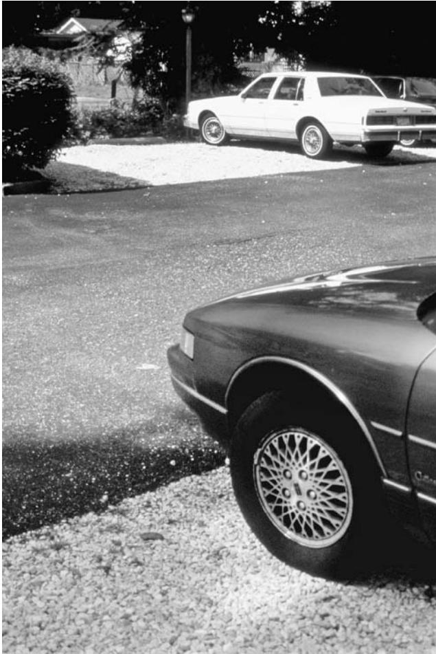
FIGURE 2.17 A parking lot for a small office in Medford Village, New Jersey, selectively combining dense asphalt and porous aggregate.
