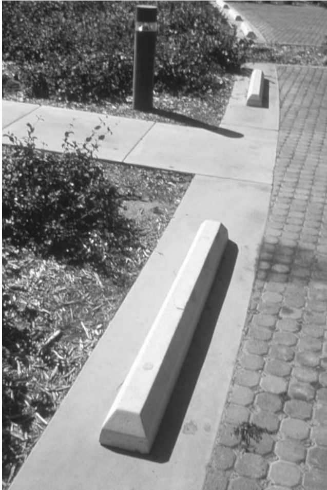
FIGURE 3.27 Concrete wheel stops at the Castaic Lake Water Conservatory in Santa Clarita, California, held by metal pins to a cast-in-place concrete edge; the parking lot pavement is Eco-Stone open-jointed block.
