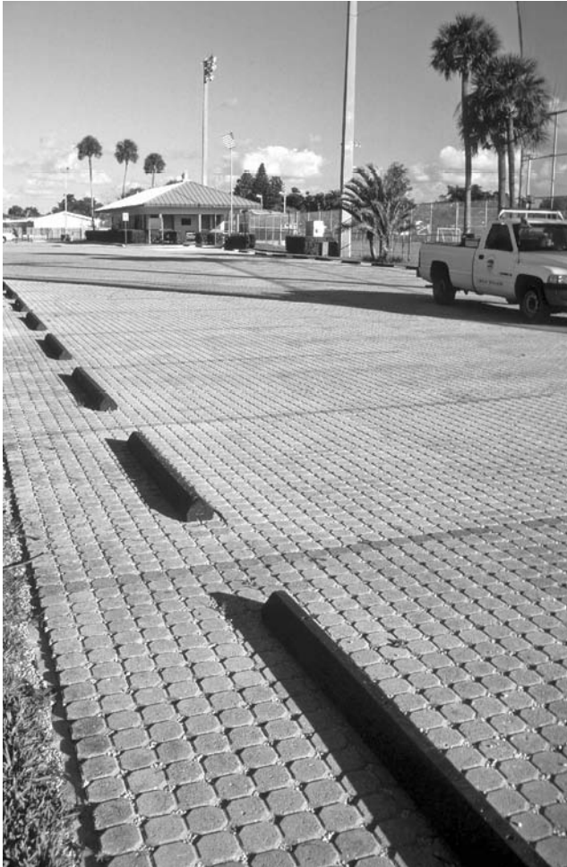
FIGURE 9.20 Eco-Stone parking lot at Mickel Field, Wilton Manors, Florida.
