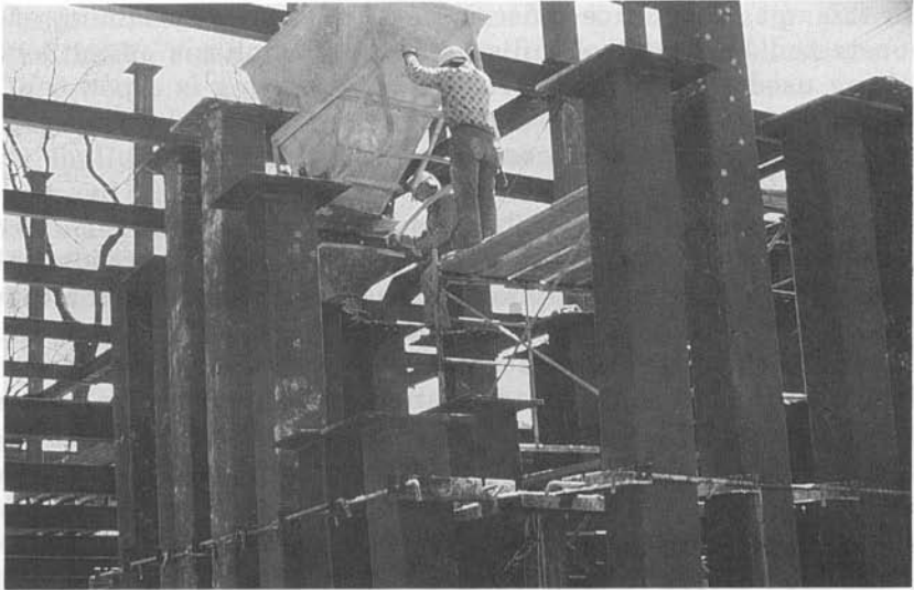
(a) Filling HSS columns with concrete on site, Hamilton, Ontario
