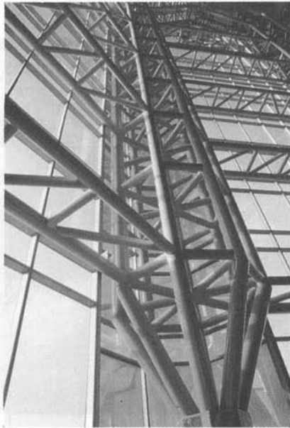
(c) Atrium of Markham Suites Hotel, Ontario
