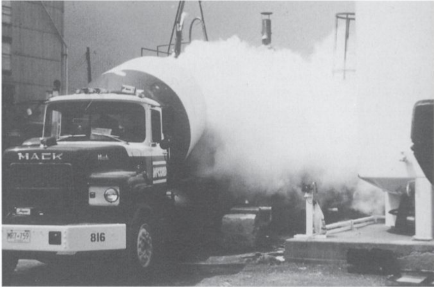
Fig. 9.2 Liquid nitrogen cooling of the high-performance concrete used to build Scotia Plaza in Toronto.
