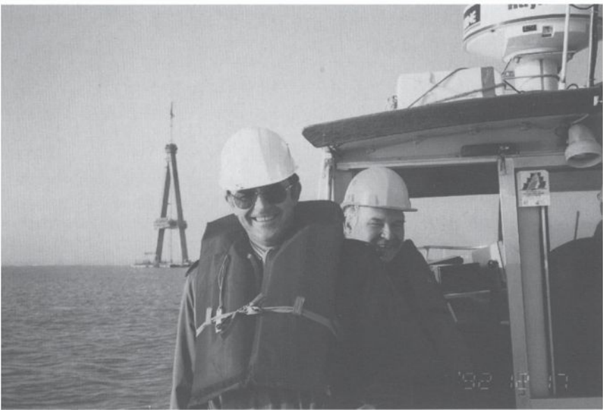
Fig. 4.15 'Pont de Normandie' under construction. One of the two pylons in construction during a visit of the author (pale hat) in December 1992 with Jean-François de Champs (darker hat) of Campenon Bernard Company.
