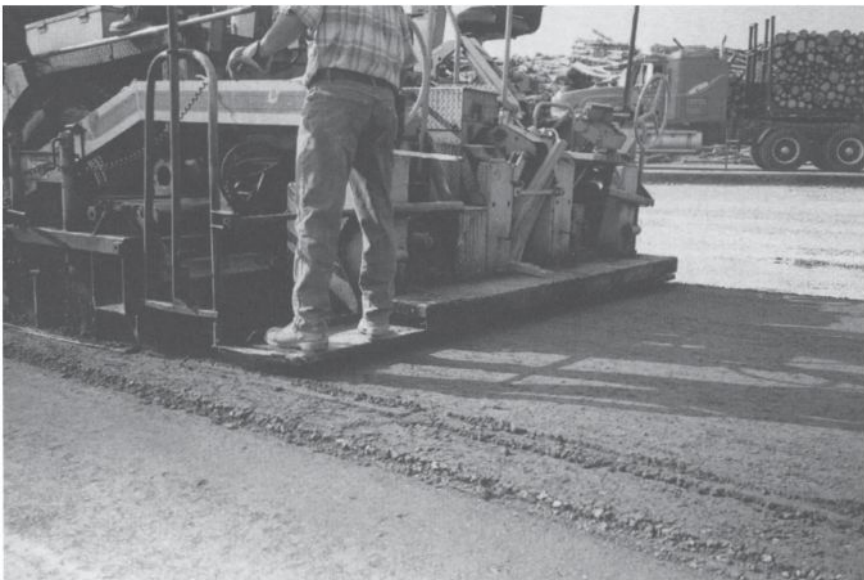
Fig. 18.12 The surface of the roller-compacted high-performance concrete just after the placing by the asphalt paver.
