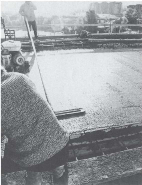
Fig. 11.3 Finishing of the Jacques-Cartier bridge deck in Sherbrooke.
