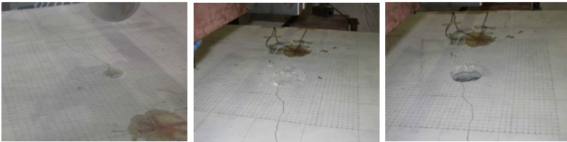
Fig. 4. Damage development in RC100 panel on impact face at 1 st impact (left), 2 nd impact (middle), and 3 rd impact (right)
