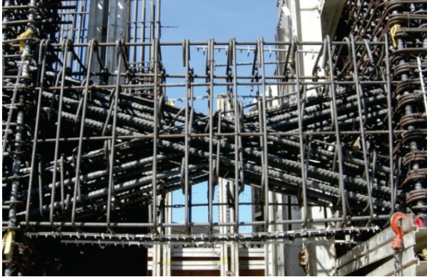
Fig. 1. Reinforcement detailing in diagonally reinforced coupling beam
