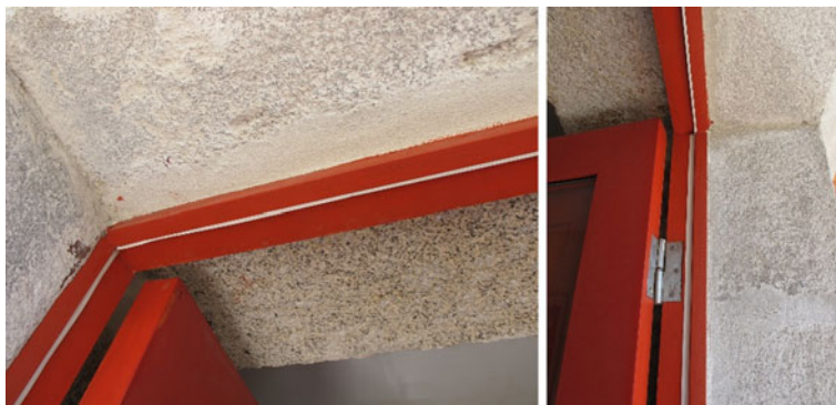
Fig. 6 Introduction of sealants in the window of the main façade
