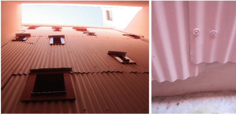
Fig. 4 Rear façade: coating made from galvanised sheet steel painted
