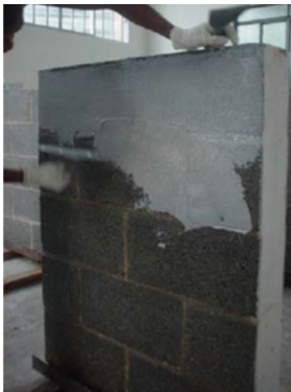
Fig. 4 Putty application. Source Chagas (2005)
