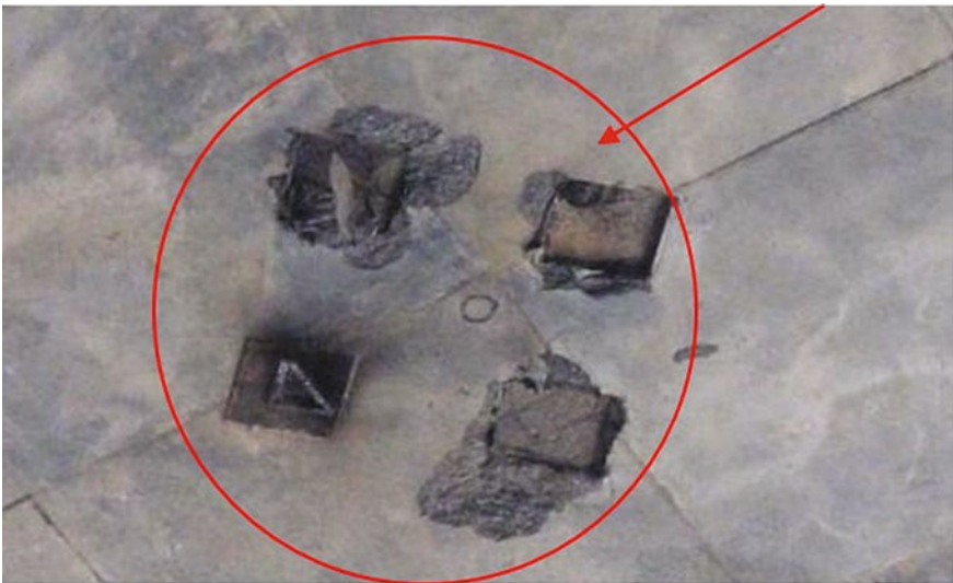
Fig. 2 Marks on the slabs of the methodology towers
