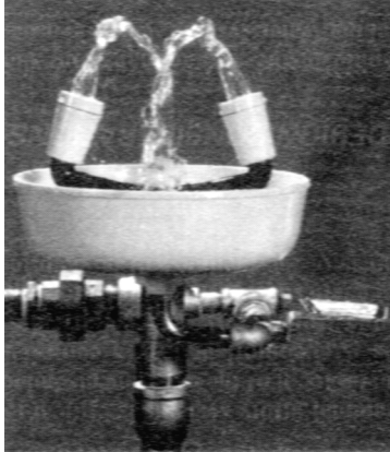
FIGURE 17.3 Stream from typical eyewash.
