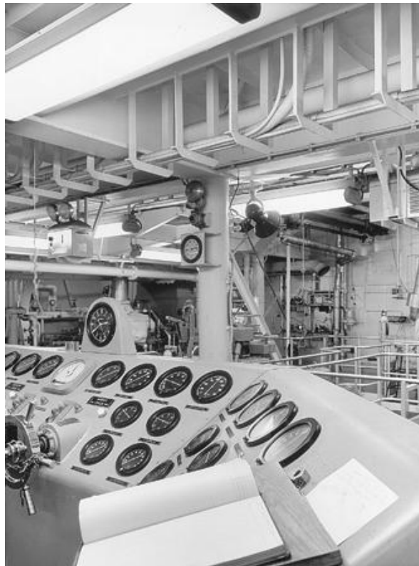
Figure 23-27. Lighting for the engineering control console is provided by fluorescent luminaires. Care should be taken to avoid glare and veiling reflections.
