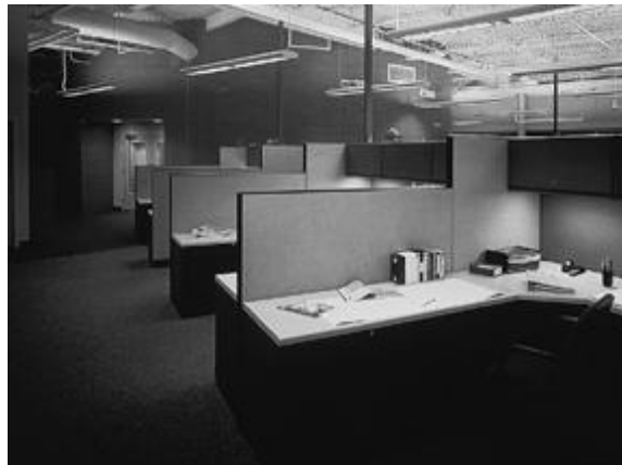
Figure 11-13. An open-plan office with direct-indirect fluorescent luminaires in a regular pattern, providing ambient light for the workstations beneath.
