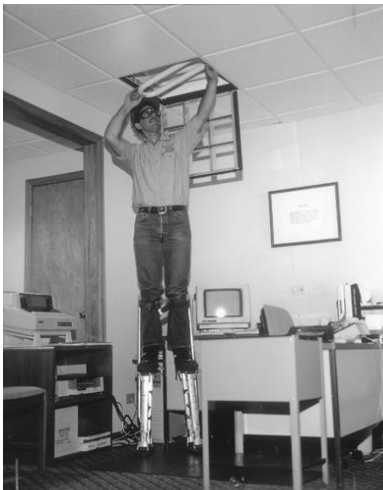
Figure 28-4. Stilts used for maintenance in spaces with low ceiling heights.
