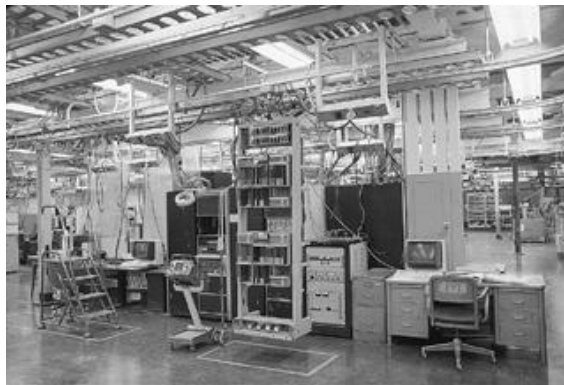
Figure 19-1. VDTs are now commonplace in manufacturing facilities, and proper placement of luminaires improves the visibility of information on the screen. Note the luminaires reflected in the screens of the VDTs in this photo. Consideration should be given to luminaire locations to reduce this effect.
