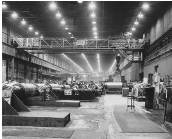
Figure 19-25. High bay roll storage area lighted with deep reflector, direct luminaires with high efficacy HID lamps having suitable color rendering characteristics. The luminaire row located close to the wall improves luminance on the wall surface.
