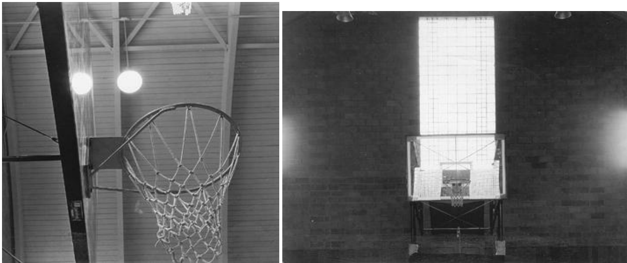
Figure 20-5. Luminaires directly over the basket (a) or windows behind the basketball board (b) produce direct glare to players.
