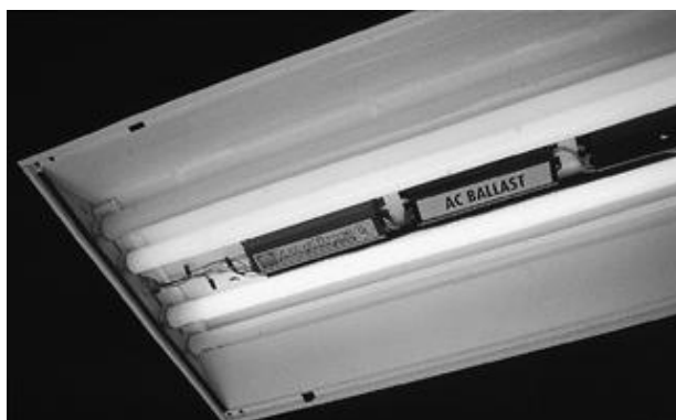
Figure 29-9. An example of a battery-inverter unit mounted in a suspended fluorescent luminaire adjacent to the ballast.
