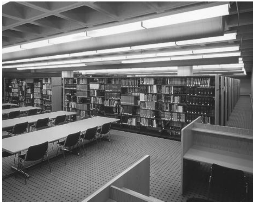
Figure 12-6. Open-access stacks are lighted with rows of fluorescent luminaires parallel to the stacks.
