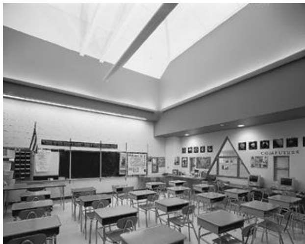
Figure 12-3. Uplighting is used to light a vaulted-ceiling classroom. A suspended uplight luminaire is
