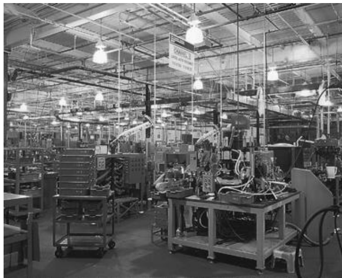
Figure 19-3. Uniform lighting for areas with similar seeing tasks provides a good visual environment and a flexible operation that allows for relocating the task without changing the lighting.
