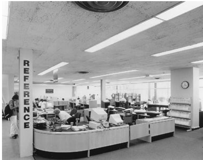
Figure 12-7. Direct lighting in a library using fluorescent luminaires for general illumination and for highlighting the circulation desk.
