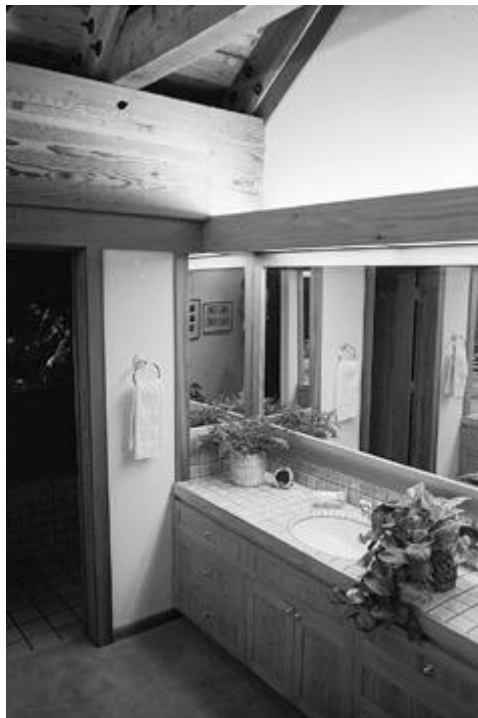
Figure 18-6. This bath features a simple soffit with overlapping up/down 4 ft T-12 fluorescent striplights that provide an even wash of light. The luminaires are outfitted with wooden egg-crate louvers.
