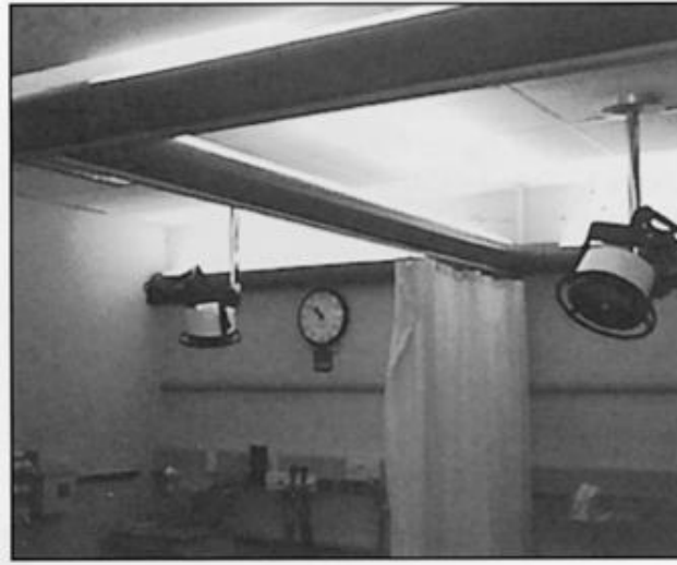
Figure 16-9. This post-anesthesia recovery room has indirect lighting that restricts glare to awakening patients.
