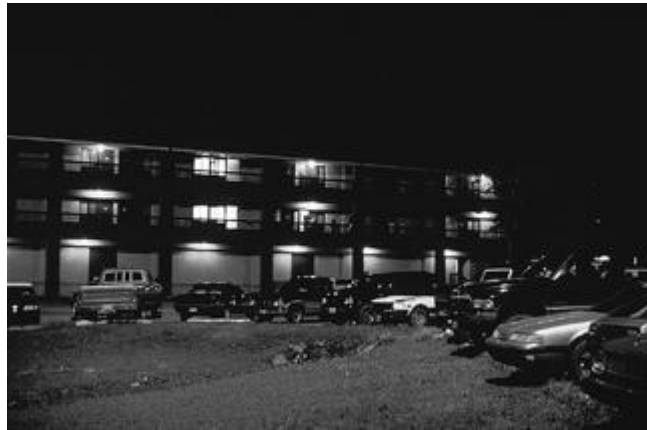
Figure 21-10. The wall-pack lighting causes light trespass into the building's windows.
