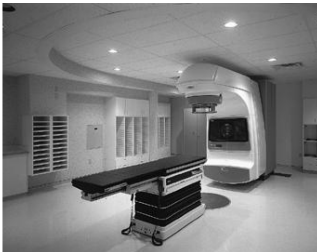
Figure 16-13. Dimmable incandescent downlights are used in this MRI scanning room.
