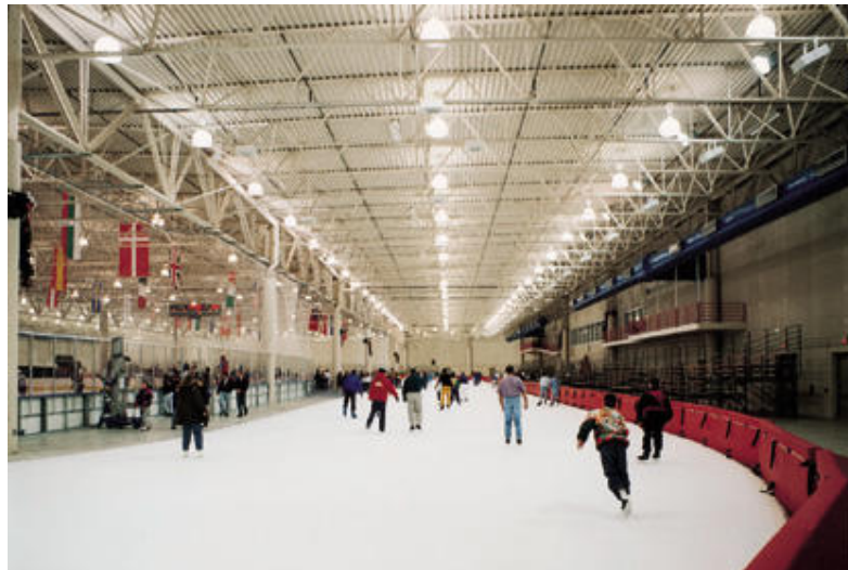
Plate 9. Metal halide lighting in industrial luminaires installed over this skating rink provides good general illumination for skaters and a glare-free ice surface. The upright contribution creates a feeling of spaciousness and pleasantness in the space.
