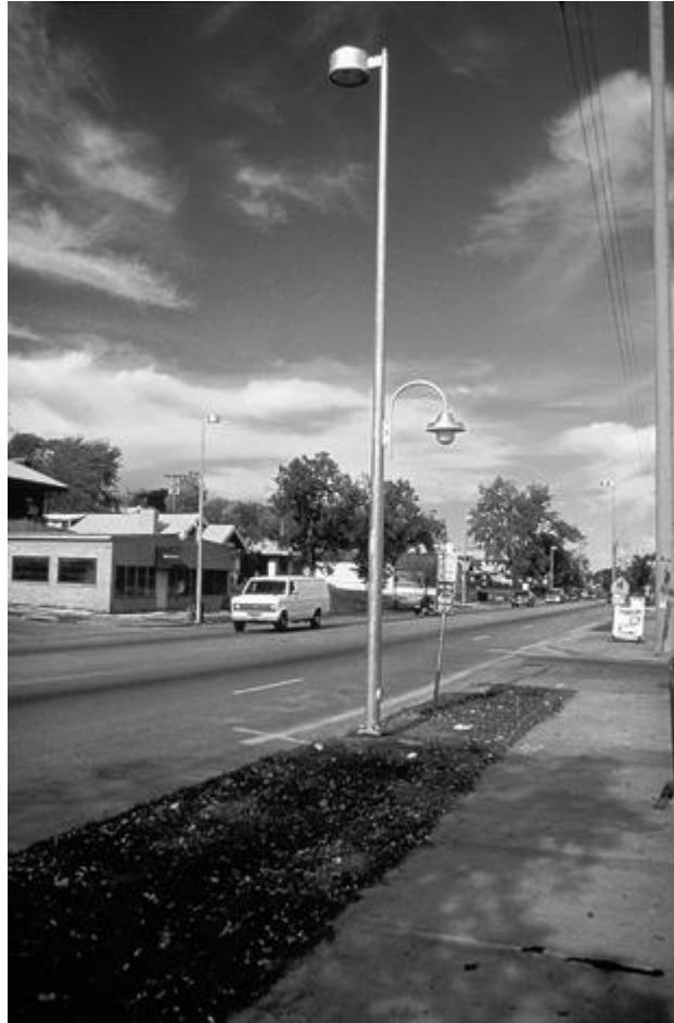
Figure 21-3. The height and location of poles contributes to the hierarchy of exterior lighting equipment along this street.
