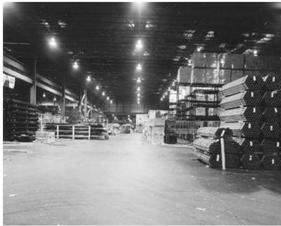
Figure 19-31. General lighting systems can be effective in storage areas where no established racks are installed, and materials may be stored on the floor or on stacked pallets.
