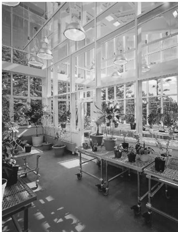
Figure 5-23. This modern greenhouse in a college science building has high pressure sodium lighting in addition to large expanses of glazing that allow for plant growth with daylight.
