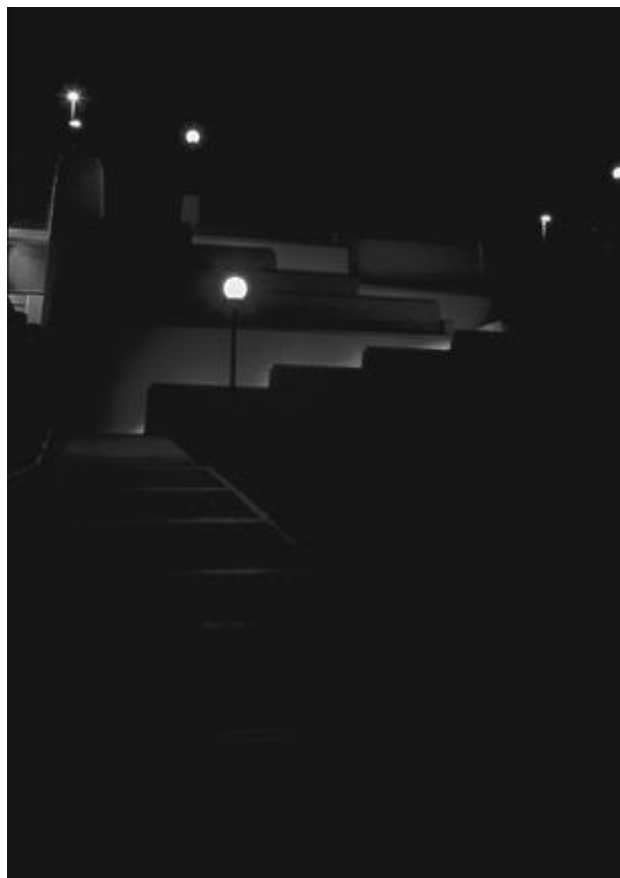
Figure 21-8. Layered lighting emphasizing the stair hazard with silhouette outlining.
