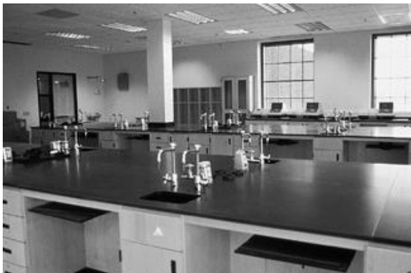
Figure 12-4. Fluorescent lighting is used to provide high illuminance in a chemistry laboratory. The parabolic louvers help control glare from equipment used in a laboratory including bench tops, glassware, and VDT screens.
