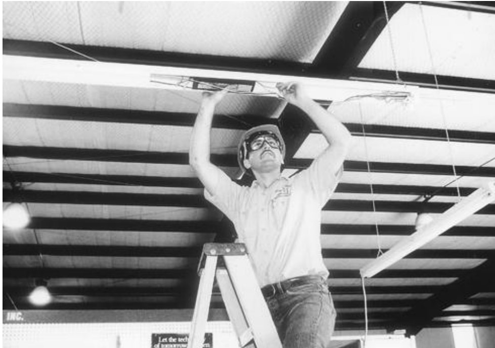
Figure 28-3. A ladder is used to change a ballast.
