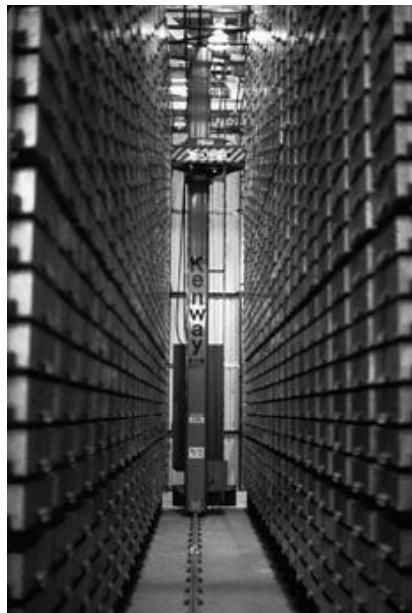
Figure 19-30. Even in automated storage areas, proper lighting is required to allow for necessary movement in the area, for required maintenance operations, and to facilitate closed circuit TV (CCTV) where it is included in the system.
