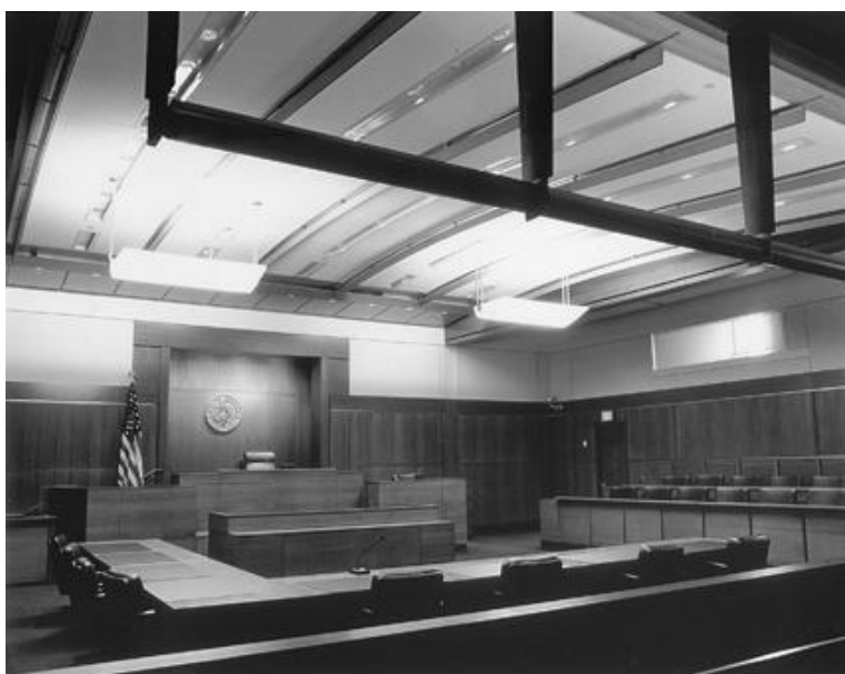
Figure 14-23. The 15 courtrooms in the Mark O. Hatfield U.S. Courthouse are lighted with a combination of 32-watt T-8 fluorescent lamps with electronic ballasts plus 50-, 60- and 100-watt halogen lamps. The lighting is controlled by a system on the judge's bench.
