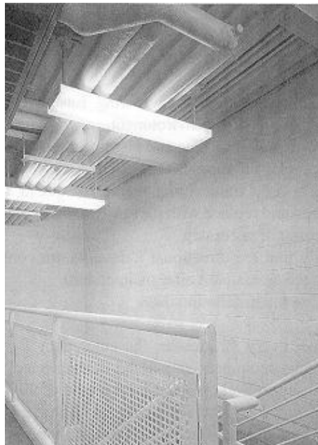
Figure 29-16. Adequate safety lighting must be used in spaces with obstructions or changes in direction or level, such as stairwells.
