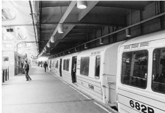
Figure 23-17. Downlights illuminate the platform and car door area. Horizontal illuminance is important since the viewing task is at the platform and entrance tread. Color should be selected to properly render the color of painted hazard markings.
