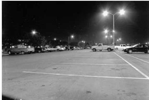
Figure 17-17. High-glare parking lot illumination.
