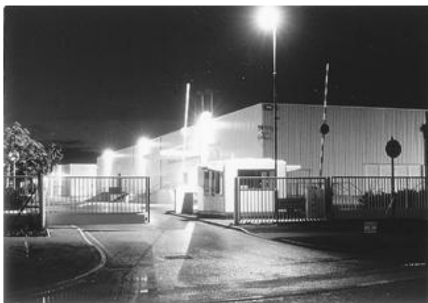
Figure 29-21. Secure entrances must be sufficiently illuminated to enable inspection of visitors or automobiles.
