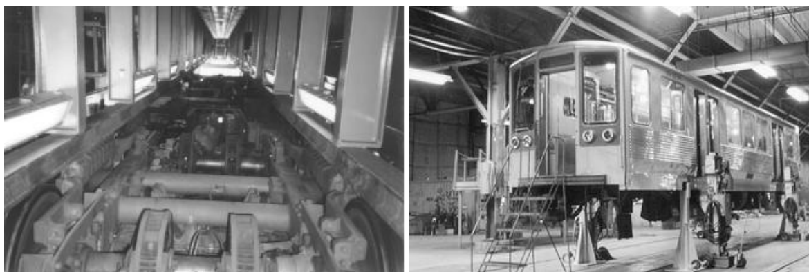
Figure 23-16. Car shop lighting. (a) Linear fluorescent luminaires in suitable environmental housings provide light to the underside of rail cars to allow maintenance work to be done with speed and accuracy. (b) Wide-distribution fluorescent luminaires provide good general lighting and vertical illuminance to facilitate cleaning
