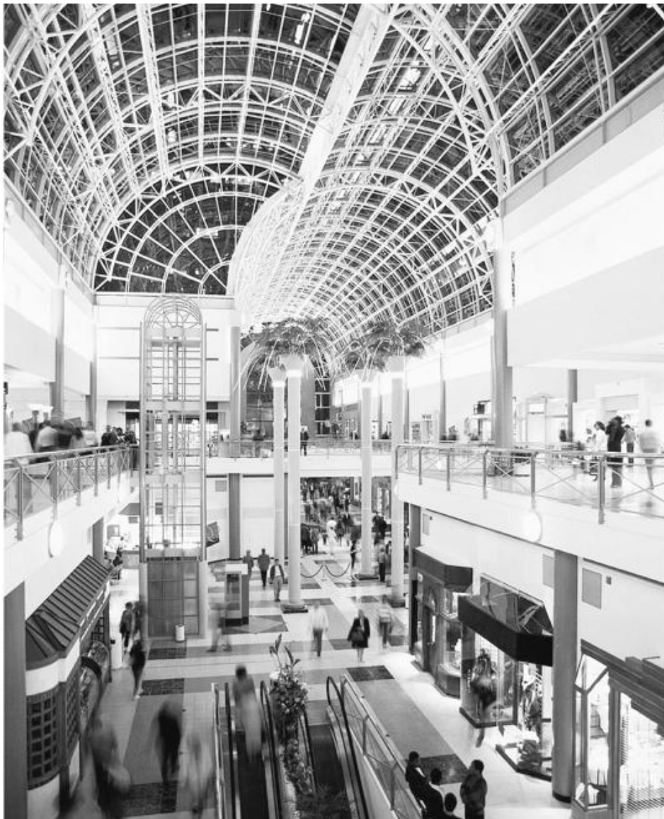
Figure 17-22. A mall's glazing should look appealing both day and night. In this atrium, exposed light sources are mounted to the structural framing system, resulting in luminous effects that are reflected and
