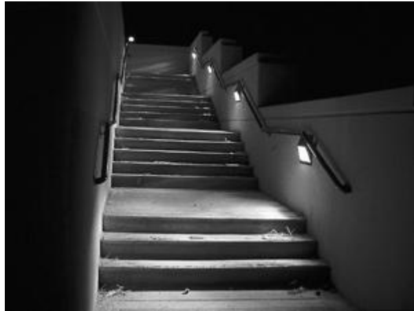
Figure 21-7. Effective hazard lighting on stairs. This lighting is unidirectional, emphasizing stair treads.
