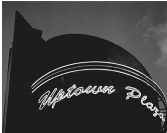
Figure 17-32. The signage for a mall illuminated with fiber optics. The individual bands above the script lettering are each sourced by separate illuminators. Side-emitting fiber tubing was mounted in sections of mounting track to follow the contour of the bands. The script words were formed from fiber tubing that was penetrated in an out of the channel letter and mounted with silicone adhesive and sourced by illuminators.
