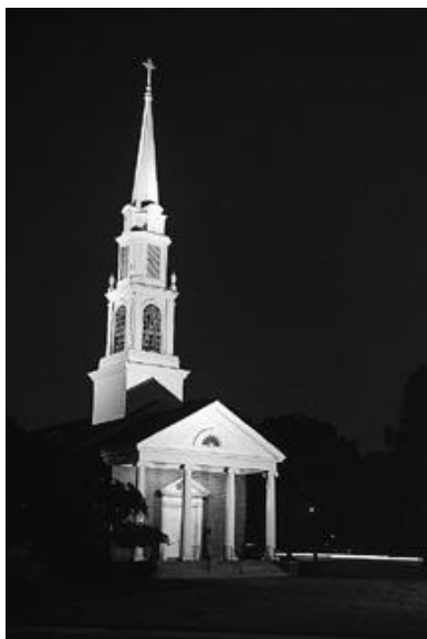
Figure 14-22. Steeple uplighted with narrow-beam floodlights.
