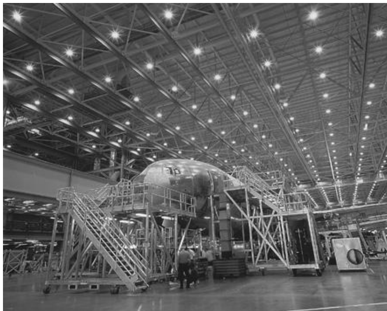
Figure 19-27. Widespread high-bay HID luminaires with uplight provide proper horizontal and vertical illuminance for large parts assembly while lighting the ceiling and walls to improve environmental surroundings.
