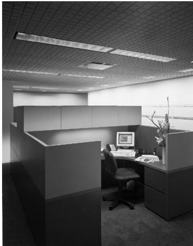
Figure 11-7. A workstation with built-in task lighting illuminating the desk top below. The low-brightness ceiling luminaire with parabolic louvers cuts down on reflections on the VDT screen.
