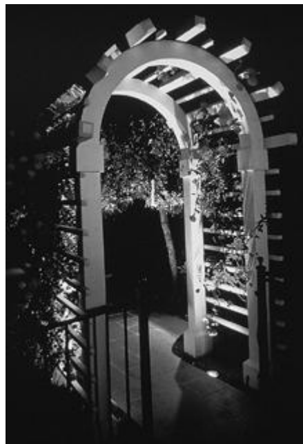
Figure 18-29. Low-voltage luminaires, mounted on stakes, uplight the structure (trellis) and the roses. MR-16 lamps are used as the light source.
