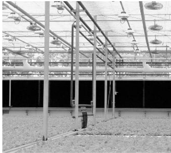
Figure 5-27. After the lettuce plants have germinated, they are brought to the pond area of the greenhouse where they are given constant light (through conventional 600-W high pressure sodium lamps), irrigation, and nutrients, until they reach full size at approximately 21 days. For the production of 1000 heads of lettuce per day, a 660 m 2 (6342 ft 2 ) growing area is required. This greenhouse serves as a "controlled environment agriculture" demonstration site for hydroponic leaf lettuce. Research methods employed here will be applied to commercial greenhouses.
