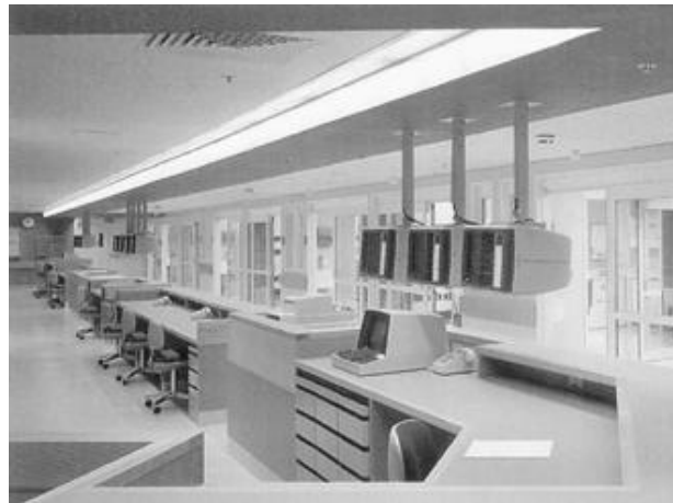
Figure 16-2. Lighting at a nurses' station is multilevel, to allow for a higher illumination during the day and a lower level at night. The lighting is designed for the critical task of reading patient information from the computer screen. Undercounter task lights also function as night lights.
