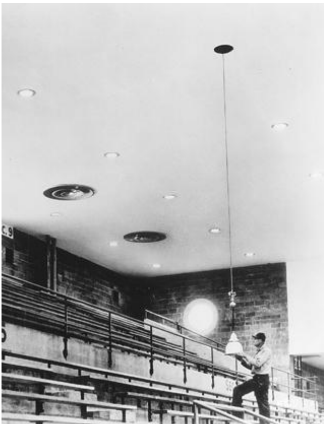
Figure 28-8. Disconnecting and lowering hangers.
