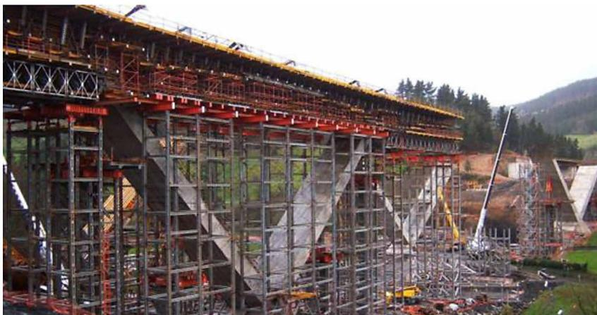
couplers, braced by diagonal members and placed under the entire formwork. These structural solutions are the same as the ones described for scaffolds.
