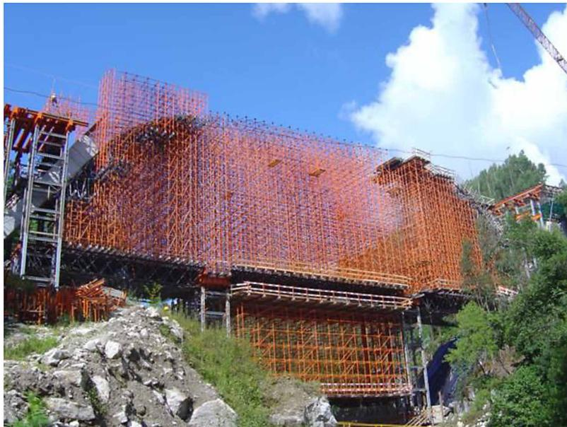
*Figure 9. Shoring example. ©2016 RMD Kwikform. Used with permission*
