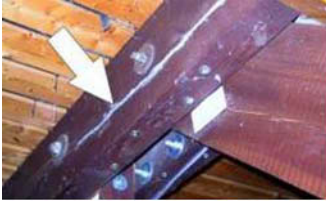
FIGURE 2. Truss of square-shaped timber
