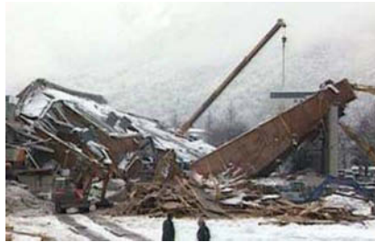
FIGURE 1. Collapse of the German ice-skating rink in Bad Reichenhall (Photo: ZDF)
