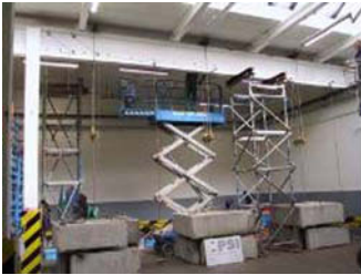
FIGURE 4. Prestressed precast girders made of high-alumina cement
