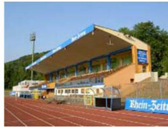
FIGURE 5. Roof of a football stadium, Koblenz.
