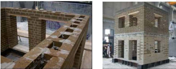
FIGURE 1. View of the three-leaf (“a sacco”) walls during construction and as-built prototype
