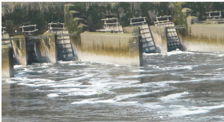
Fig. 10.6 Sewage passes through the sluice gates of the canal into the Bidyadhari River
