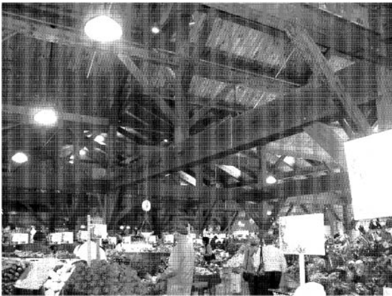
Figure 2.5-1. Market constructed using salvaged wood timbers (Photo copyright Mark D. Webster, used with permission)
