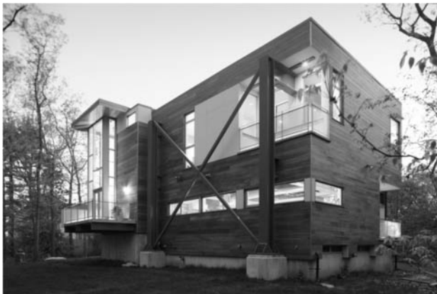
Figure 2.5-3. House constructed with salvaged steel, designed by SsD (Photo copyright SsD, used with permission)
