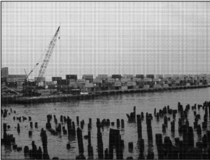
Figure 5.4-2. The Nomadic Museum under construction (Photo copyright Buro Happold)
