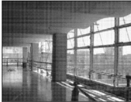
Figure 1.2-5. A construction photo taken in an office space shows the raised soffit of the wing slab, which highlights the form of the wave slab and allows additional daylight to enter the space. (Photo courtesy of Chuan Do)
