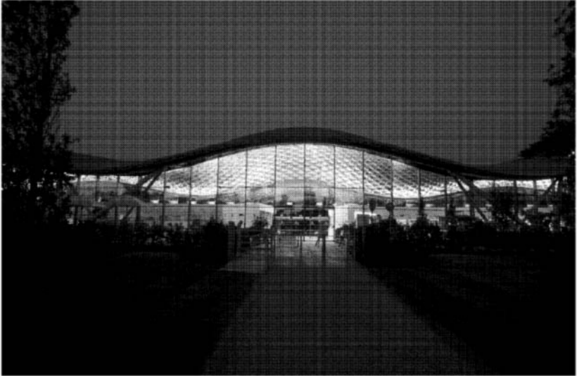
Figure 5.10-1. This site-sensitive project reflects the surroundings. (Photo copyright Warwick Sweeney)
