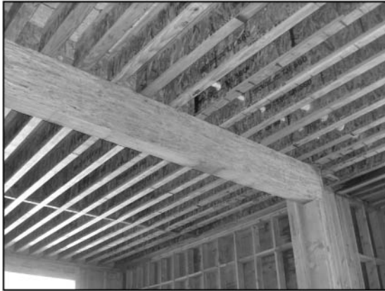
Figure 3.5-6. Engineered wood products utilize wood efficiently. (Photo by DeStefano & Chamberlain, used with permission)
