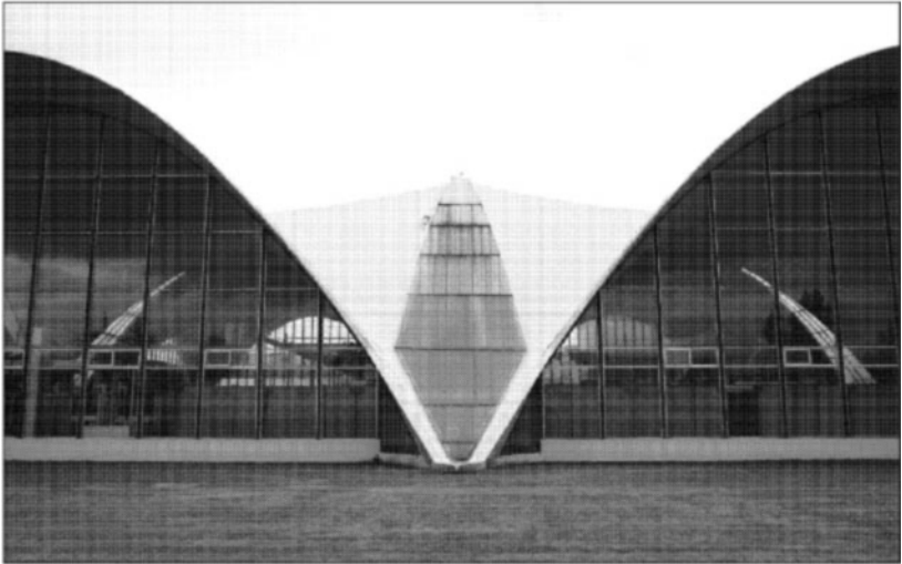
Figure 5.1-1. Bacardi y Cia Warehouse, exterior view of groined vaults. (Photo by Bruce M. White)
