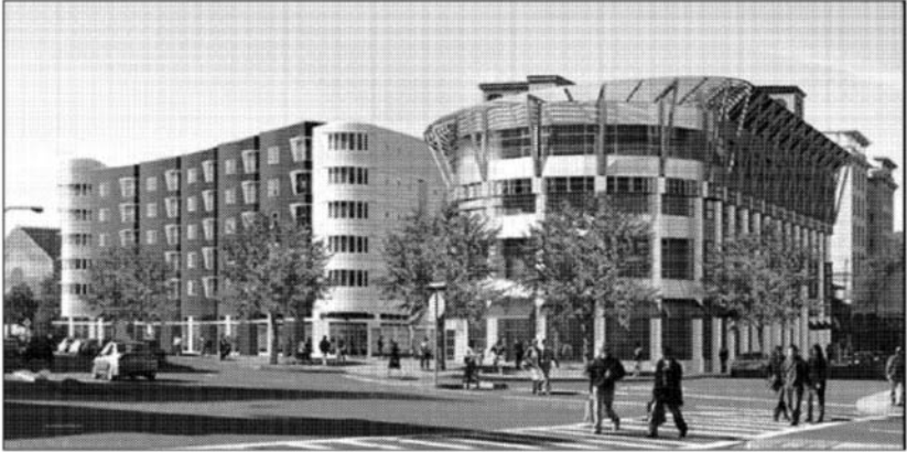
Figure 5.7-1. Designed to achieve a LEED rating, the project’s ultimate goal was to remain functional after an earthquake. (Photo copyright WRT/Solomon E.T.C.)
