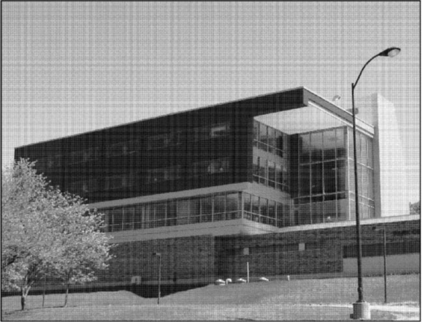
Figure 5.6-1. Ithaca College Business School obtained a LEED-platinum rating. (Photo copyright Graham Steward, used with permission.)
