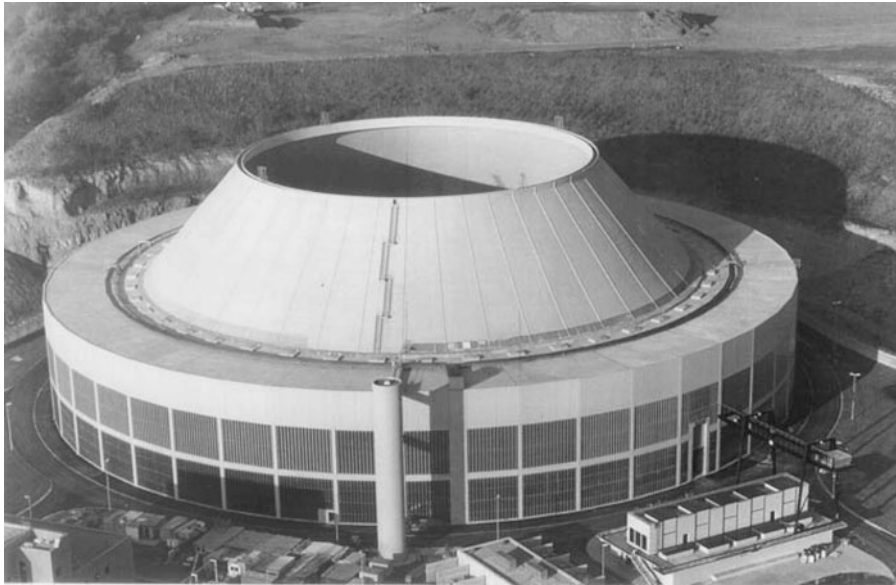
Fig. 11.1 Cooling tower of power plant equipped with parallel baffle silencers (Source: BBM-Gerb Akustik)
