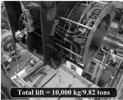
Figure 6.27 The lift in progress. Reproduced with permission of Quartzelec, Aberdeen Scotland.
