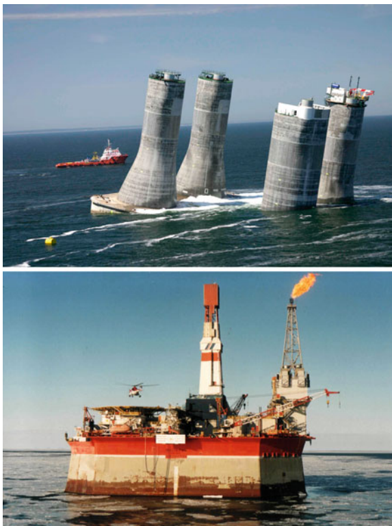
Photo 5.9 Base of drilling platform ( top ) is set (submersed) first on-site of future well, at which then the “roof” is attached ( bottom ) (Photo by V.Pishchalnik)
