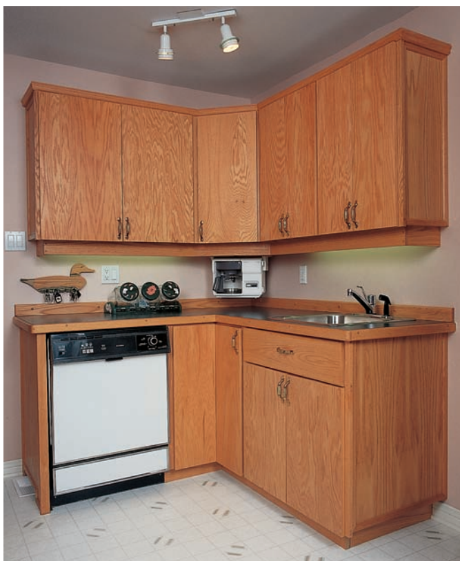
The doors for this kitchen were made using \frac{3}{4} "-thick oak-veneer particleboard with taped wood-veneer edges.
