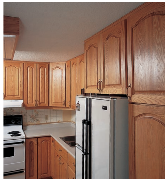
Five-piece wood cabinet doors with solid raised panels are the most expensive door style. Substituting the solid-wood core for a \frac{1}{4} "-thick veneer plywood center panel can reduce the price.
