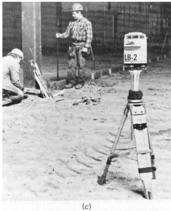
FIGURE 11-26. (a, b) The construction surveyor must accurately locate the footing and column positions for a proposed structure. (c) Laser instruments are often used to establish construction elevations. (Courtesy of Laser Alignment, Inc.)
