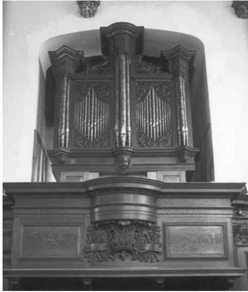
Figure 19.1 General view of the organ, showing the wooden case which contains the pipes, and below, the organ loft where the player sits.
