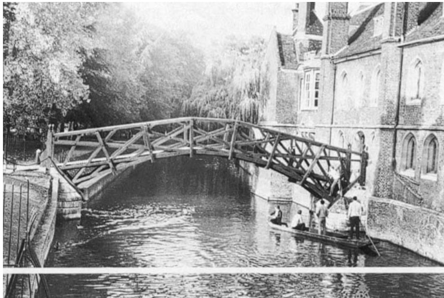
Figure 1.6 The wooden bridge at Queens' College, Cambridge, a 1902 reconstruction of the original bridge built in 1749 to William Etheridge's design.
