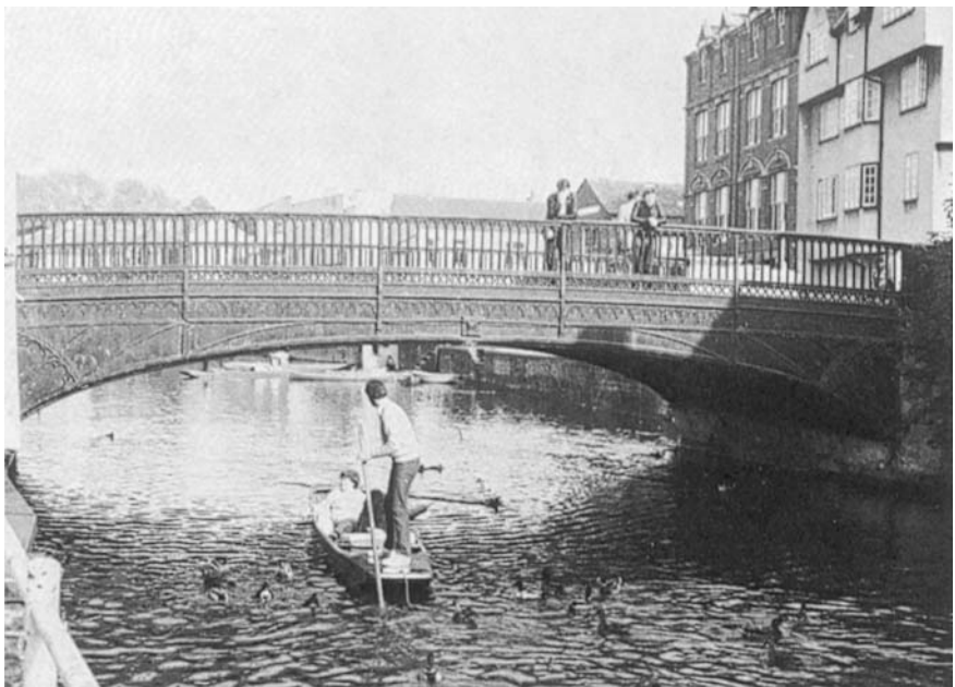
Figure 1.8 Magdalene Bridge built in 1823 on the site of the ancient Saxon bridge over the Cam. The present cast-iron arches carried, until recently, loads far in excess of those envisaged by the designers. Fortunately, the bridge has now undergone a well-earned restoration.
