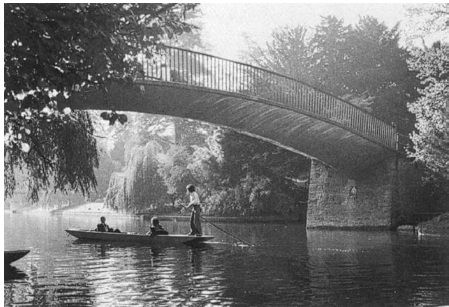
Figure I.10 The reinforced concrete footbridge in Garret Hostel Lane. An inscription carved nearby reads: "This bridge was given in 1960 by the Trusted family members of Trinity Hall. It was designed by Timothy Guy Morgan an undergraduate of Jesus College who died in that year."
