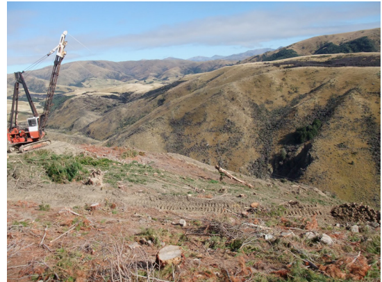
Figure 3. Cable hauler bringing up a log
