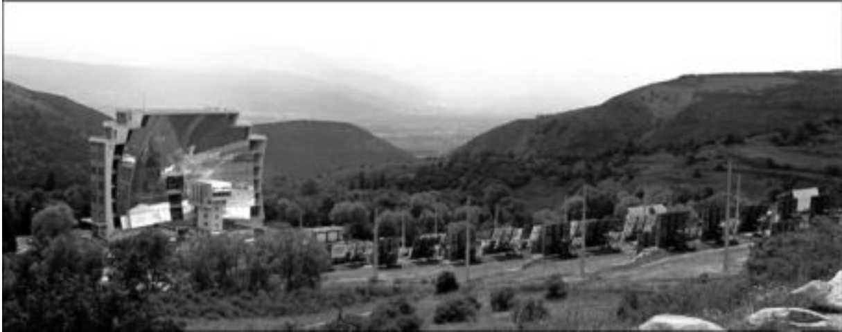
FIG. 5.8 SOLAR FURNACE IN FRANCE [12]
