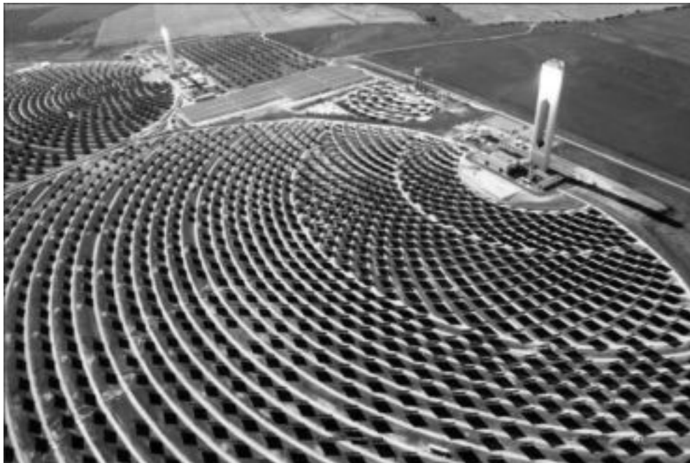
FIG. 3.13 AERIAL VIEW OF THE FIRST COMMERCIAL SOLAR TOWERS IN THE WORLD. PS20 WITH 20 MW AT THE FRONT AND THE PS10 WITH 11 MW AT UPPER LEFT. HELIOSTAT FIELD LAYOUT IS FORMED BY HUNDREDS OF TRACKING MIRRORS FOCUSING CONCENTRATED LIGHT ONTO THE RECEIVER APERTURE. PS20 AND PS10 HAVE BEEN DEVELOPED AND THE TECHNOLOGY IS OWNED BY ABENGOA SOLAR S.A. AND ARE LOCATED IN SANLUCAR LA MAYOR, SEVILLE, SPAIN (Source: Abengoa Solar, S.A.) (All rights reserved on Figure 3.13 to Abengoa Solar, S.A. © 2010)
