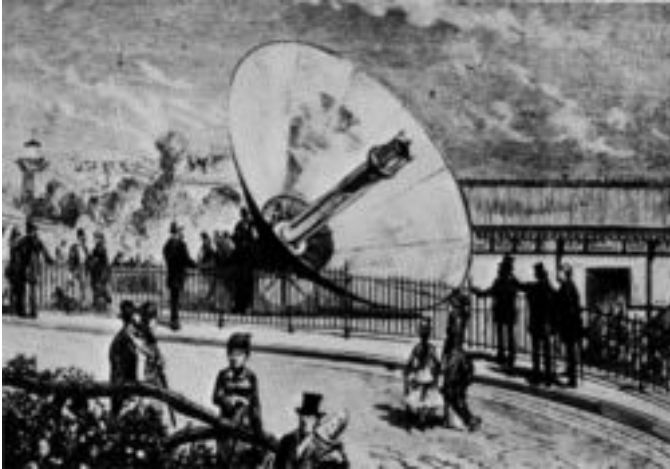
FIG. 5.1 SOLAR STEAM ENGINE [4]
