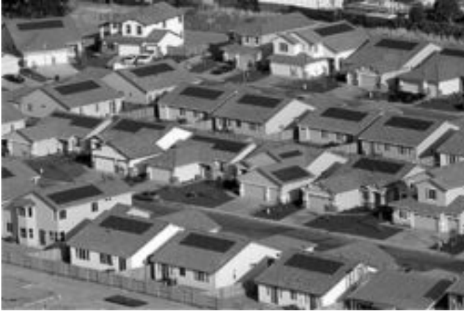
FIG. 5.11 PV RESIDENTIAL SOLAR ARRAY (Courtesy of DOE/NREL)
