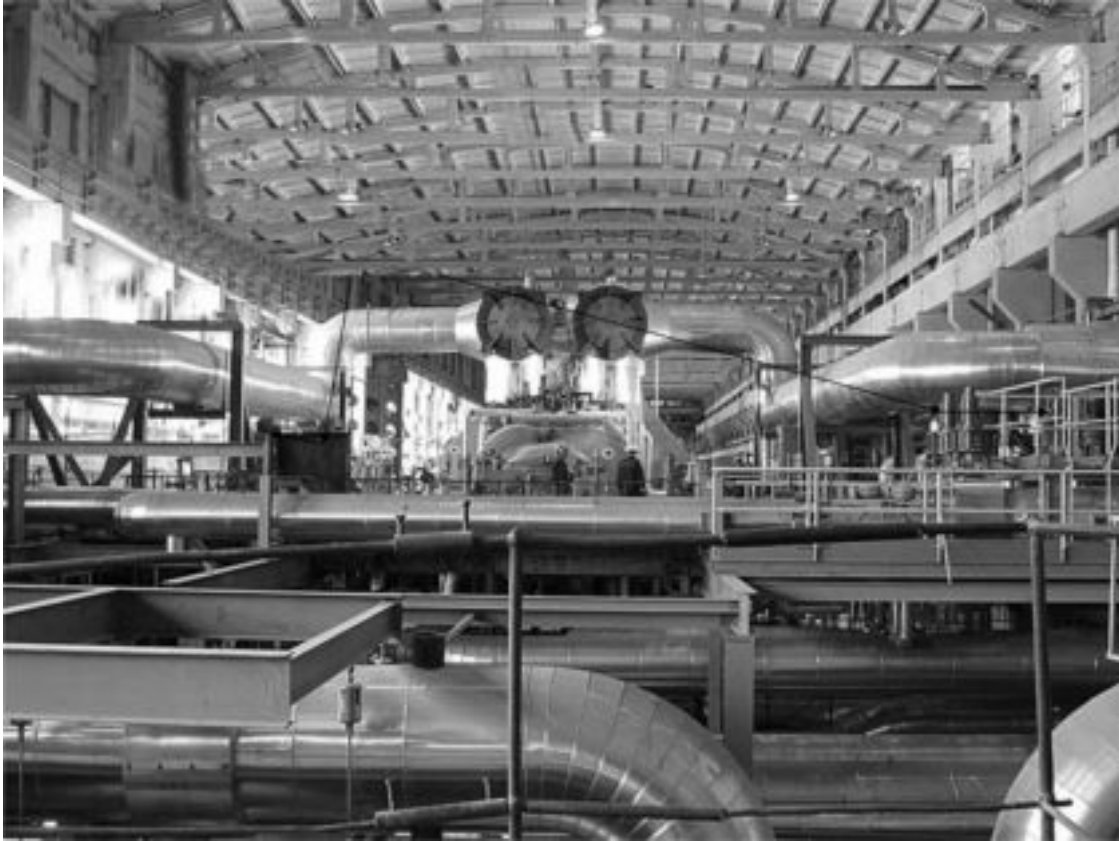
FIG. 27.4 STEAM BLED AFTER IP STAGE OF STEAM TURBINE FOR TOWN CENTER HEATING PURPOSES
