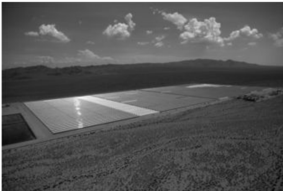
FIG. 1.4 NEVADA SOLAR ONE, A 64 MWE (75 MWE MAXIMUM) PLANT BUILT BY ACCIONA SOLAR POWER BEGAN ELECTRICAL PRODUCTION NEAR LAS VEGAS DURING 2007 (Courtesy Acciona Solar Power)
