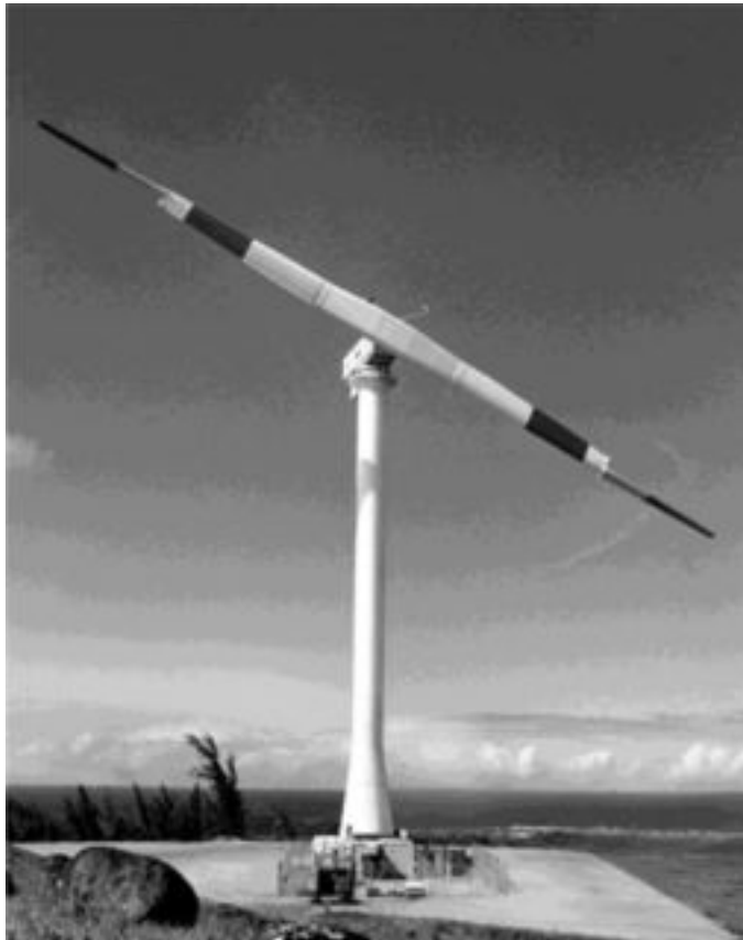
FIG. 6.28 THE NASA/DOE/BOEING MOD-5 IN HAWAII PIONEERED VARIABLE SPEED GENERATORS AND WAS THE WORLD'S LARGEST OPERATING WIND TURBINE INTO THE 1990S
