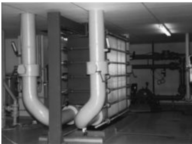
FIG. 16.23 THIS IS A “PLATE TYPE” HEAT EXCHANGER, WHICH PASSES HOT GEOTHERMAL WATER PAST MANY LAYERS OF METAL PLATES, TRANSFERRING THE HEAT TO OTHER WATER PASSING THROUGH THE OTHER SIDE OF EACH PLATE WHERE THE HEATED FLUID IS USED FOR SPACE HEATING (Source: [59])
