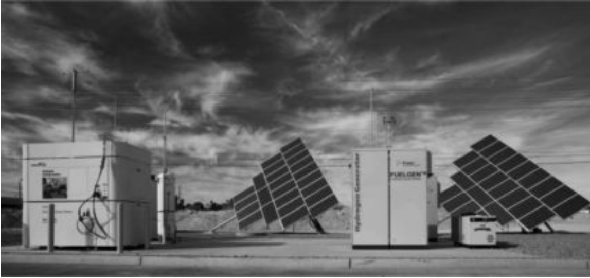
FIG. 1.15 THE UNLV/LAS VEGAS VALLEY WATER DISTRICT SOLAR POWERED HYDROGEN GENERATION AND FILLING STATION IS SHOWN. TO THE RIGHT IN THE FIGURE IS THE ELECTROLYZER SYSTEM, TO THE LEFT ARE THE COMPRESSOR, STORAGE AND DISPENSING STATION, AND IN THE REAR TWO OF THE FOUR PV PANELS ARE SHOWN THAT POWER THE SYSTEM
