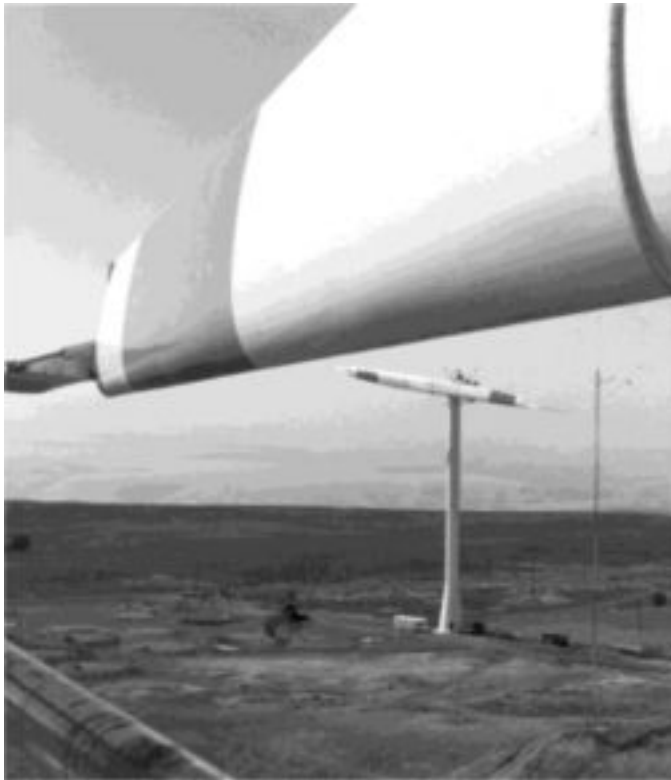
FIG. 6.26 THE NASA / DOE/ BOEING MOD-2 (2.5 MEGAWATT) WIND TURBINE WAS A SECOND GENERATION DESIGN THAT PIONEERED THE LOWER COST “SOFT” STEEL TUBE TOWERS USED IN THE INDUSTRY TODAY
