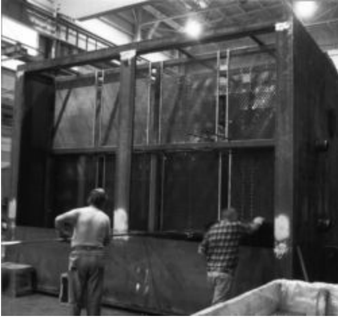
PHOTOGRAPH C: RECTANGULAR CONDENSER WITH NON-SEGMENTAL BAFFLES DURING FABRICATION (Courtesy Holtec International)
