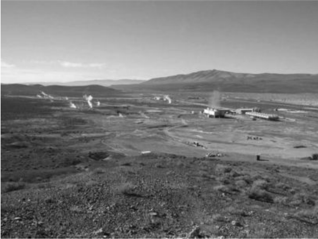
FIG. 16.8 VIEW OF BRADYS POWER PLANT AND FUMAROLES FROM A DISTANCE. BRADYS GEOTHERMAL PLANT IS OPERATED BY ORMAT, NV, AND HAS BOTH FLASH AND BINARY UNITS PRODUCING POWER (Source: [43], Photo by Mark Coolbaugh. Nov. 2, 2002)
