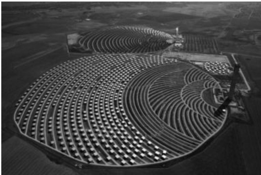
FIG. 1.7 THIS PHOTO SHOWS PS10 IN OPERATION IN THE BACKGROUND AND PS20 UNDER CONSTRUCTION IN THE FOREGROUND. PS20 STARTED POWER PRODUCTION IN 2009 (From ABENGOA SOLAR)
