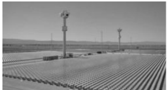
FIG. 3.17 FIRST EXPERIMENTAL EXAMPLE IN THE WORLD OF A MULTITOWER SOLAR ARRAY CORRESPONDING TO ESOLAR'S SIERRA SOLAR GENERATING STATION WITH TWO FULL-SIZED HELIOSTAT FIELDS IN LANCASTER, CALIFORNIA (Source: eSolar)
