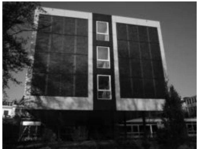
FIG. 5.10 BUILDING INTEGRATED PV (Courtesy of DOE/NREL, Credit-BP Solarex)
