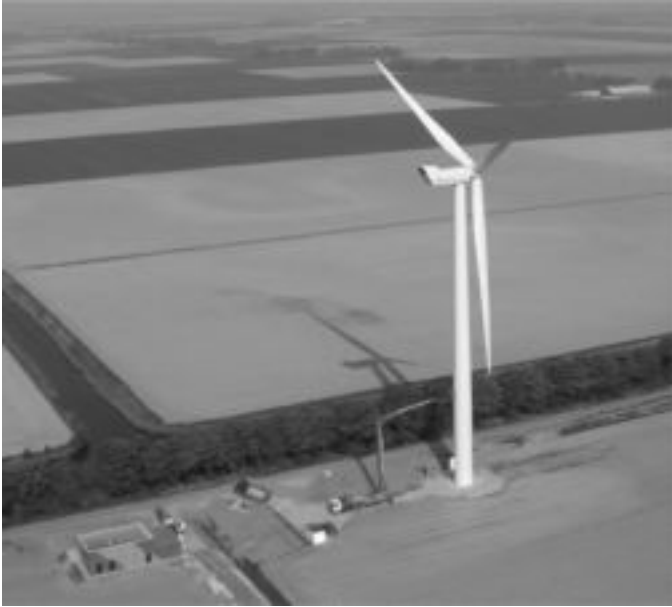
FIG. 9.1 THE NM90 2.75 MW WIND TURBINE (ALSO KNOWN AS DOWEC TURBINE) AT THE ECN TEST SITE IN THE WIERINGERMEER AS SEEN FROM THE MEASUREMENT MAST (109 M) (Source: [ECN, taken by R. Nijdam])
