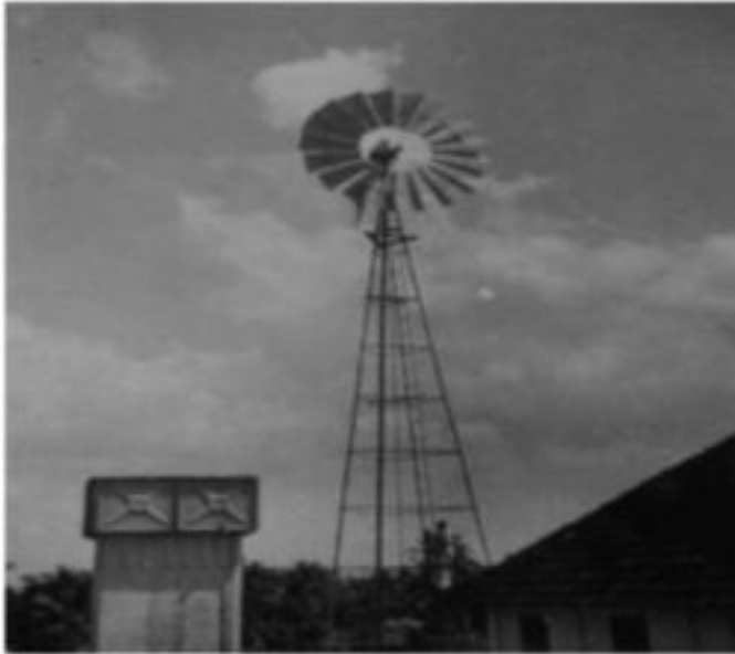
FIG. 10.1 ONE OF THE 70 WINDMILLS (MODEL WP 2) INSTALLED IN RURAL INDIA DURING EARLY 1960S
