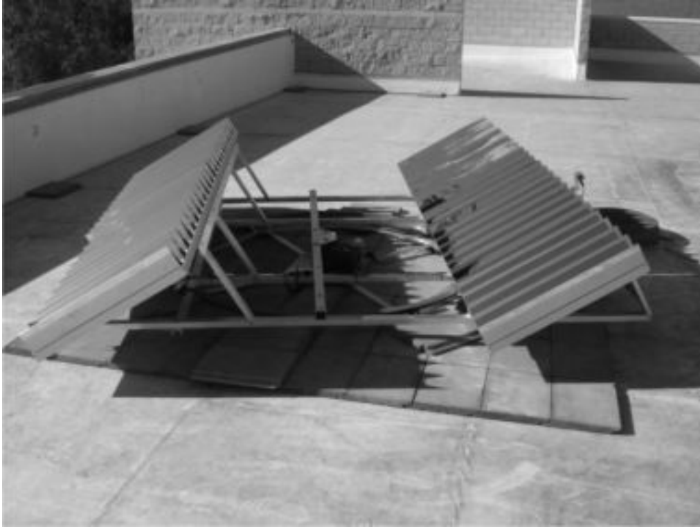
FIG. 1.14 THE JX CRYSTALS ONE-AXIS TRACKING 3X CONCENTRATION PV SYSTEM IS SHOWN (Courtesy UNLV)
