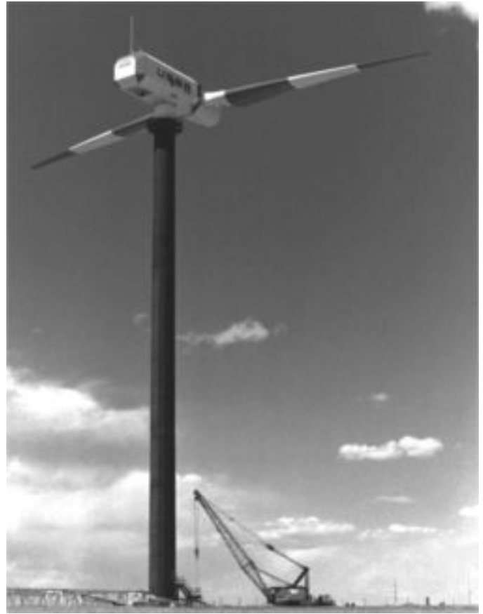
FIG. 6.27 THE NASA / DOI / HAMILTON STANDARD WTS-4 (4 MEGAWATT) WIND TURBINE IN WYOMING TYPIFIED THE “COMPLIANT” DESIGN APPROACH AND HELD THE WORLD RECORD FOR POWER OUTPUT FOR OVER 20 YEARS
