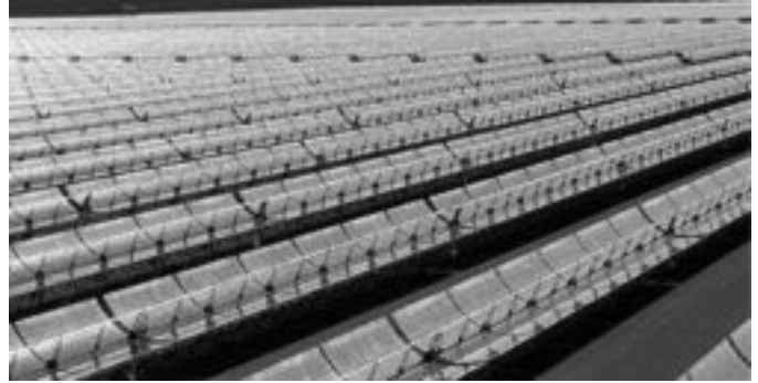
FIG. 5.13 CONCENTRATING SOLAR TROUGH (Courtesy of DOE/NREL)
