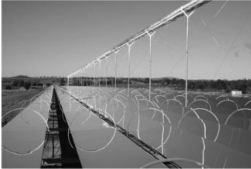
FIG. 5.14 LINEAR FRESNEL REFLECTORS (Courtesy of DOE/NREL)
