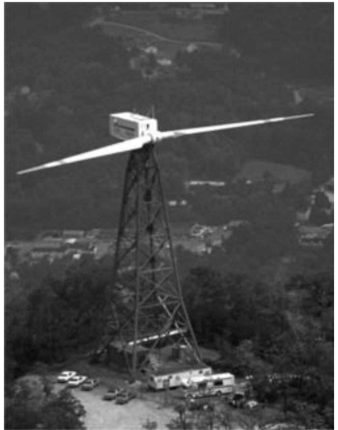
FIG. 6.25 THE NASA/GENERAL ELECTRIC MOD-1 WIND TURBINE WAS THE WORLD'S FIRST MULTI-MEGAWATT COMMERCIAL PROTOTYPE WIND TURBINE (Derived from the Mod-0 in Sandusky, Ohio)
