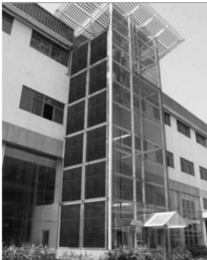
FIG. 1.22 BUILDING INTEGRATED PHOTOVOLTAICS (BIPV) ARE INCORPORATED IN A NUMBER OF THE FACADES OF THIS BUILDING [24]
