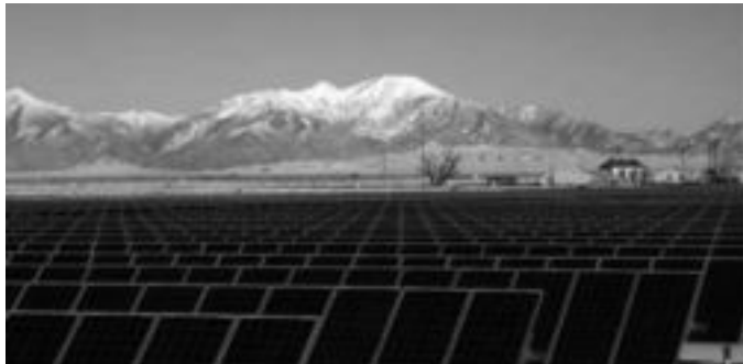
FIG. 5.9 PV PLANT (courtesy of DOE/NREL, Credit — Steve Wilcox)
