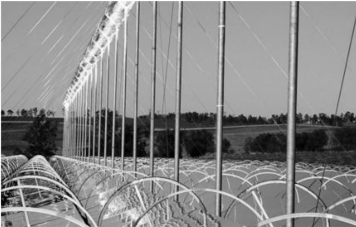
FIG. 1.5 A CONCEPT OF A FRESNEL (LINE FOCUS) SOLAR THERMAL PLANT HAS BEEN PUT FORTH BY AREVA. IN THIS APPROACH, LONG AND TRANSVERSELY NEARLY FLAT FACETS EACH ROTATE ON THE GROUND TO FOCUS THE DIRECT BEAM RADIATION ONTO A FIXED RECEIVER OVERHEAD (Courtesy of AREVA)
