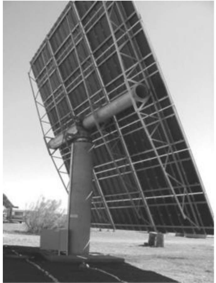
FIG. 3.14 LATERAL VIEW OF A TYPICAL GLASS-METAL HELIOSTAT WITH T-SHAPE SUPPORTING STRUCTURE FORMED BY PEDESTAL, TORQUE TUBE AND TRUSSES. REFLECTIVE SURFACE IS MADE OF FACETS WITH A METALLIC FRAME AND GLASS MIRROR. LOCAL CONTROL BOX IS LOCATED AT THE BOTTOM OF THE PEDESTAL (Source: Abengoa Solar, S.A.) (All rights reserved on Figure 3.14 to Abengoa Solar, S.A. © 2010)
