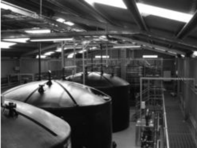
FIG. 28.8 VRB LAYOUT (Source: Hydro Tasmania)
