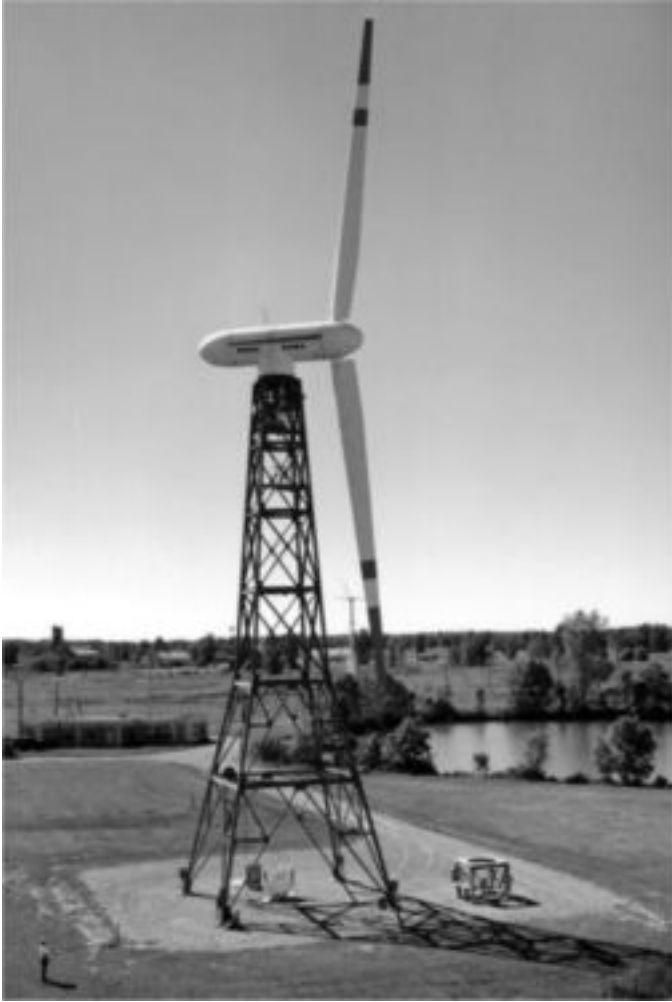
FIG. 6.24 NASA MOD-0 WIND TURBINE, INSTALLED IN SANDUSKY, OHIO IN 1975 BECAME THE TEST BED FOR DEVELOPING NEW TECHNOLOGIES FOR LARGE HORIZONTAL AXIS WIND TURBINES
