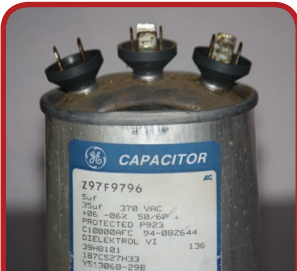
Bad run capacitor (Extruding outside normal shade). (Delmar/Cengage Learning) FIGURE 9.27
