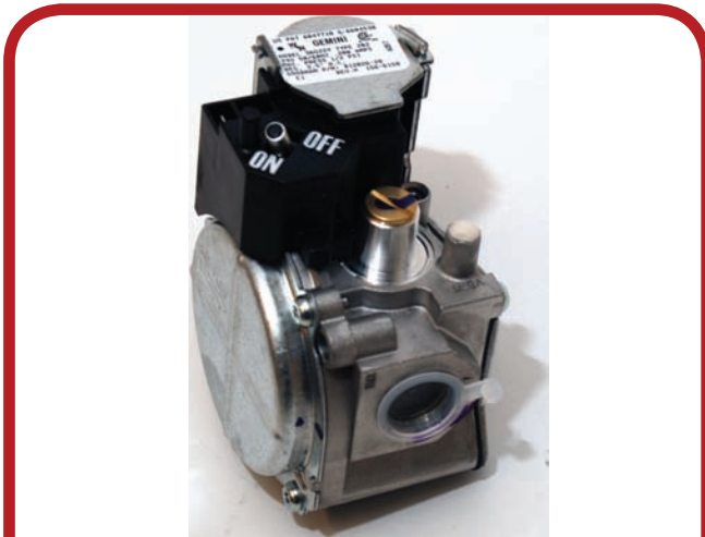
Photograph of redundant gas valve. (Delmar/Cengage Learning)
