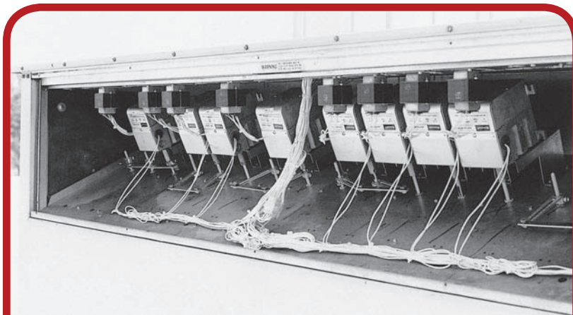
Zone damper section of multi-zone roof top packaged unit. (Delmar/Cengage Learning) FIGURE 17.18
