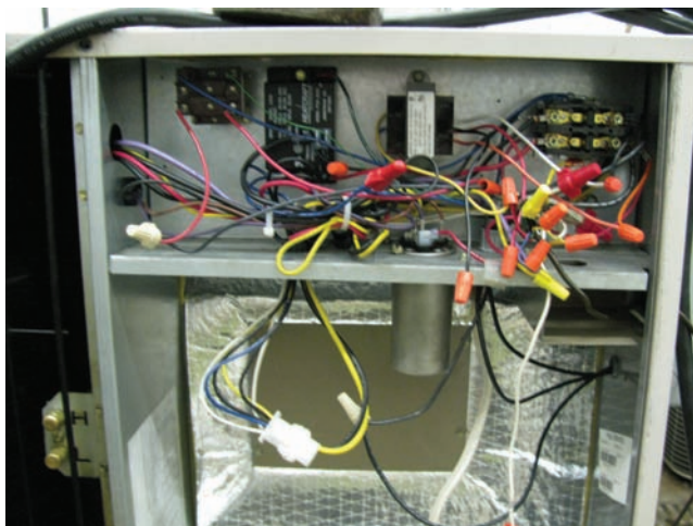
Control panel of small cooling-only packaged air-conditioning unit. (Delmar/Cengage Learning)
