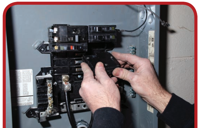
Breaker being installed in a breaker panel. (Delmar/Cengage Learning)
