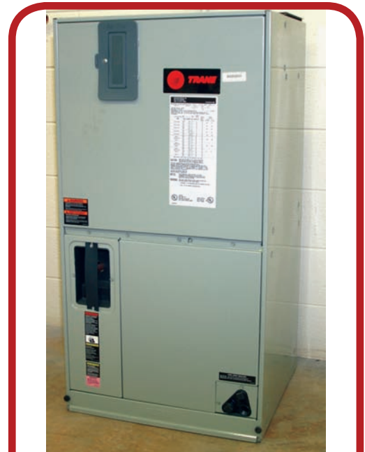
Fan-coil unit. (Photo by Bill Johnson)
