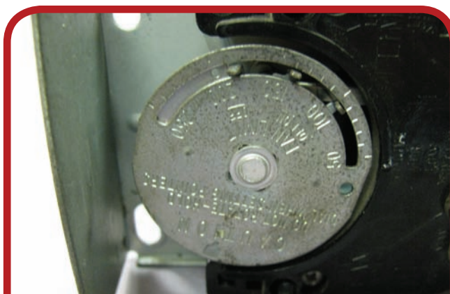
Dial of a combination fan and limit switch. (Delmar/Cengage Learning)
