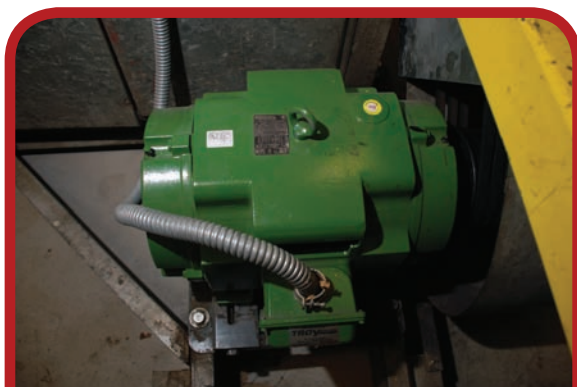
Three-phase induction motor. (Delmar/Cengage Learning) FIGURE 9.40
