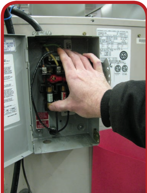
Technician becoming part of an electrical circuit by coming in contact with L1 and neutral. (Delmar/Cengage Learning) FIGURE 1.1
