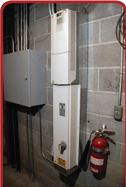
Multifunction electronic three-phase motor monitor. (Delmar/Cengage Learning)
