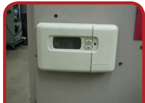
Electronic programmable thermostat. (Delmar/Cengage Learning)
