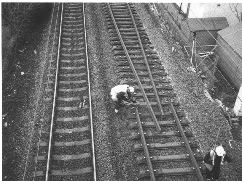
Figure 13.3 Example of Track Maintenance Activities (RSSB)
