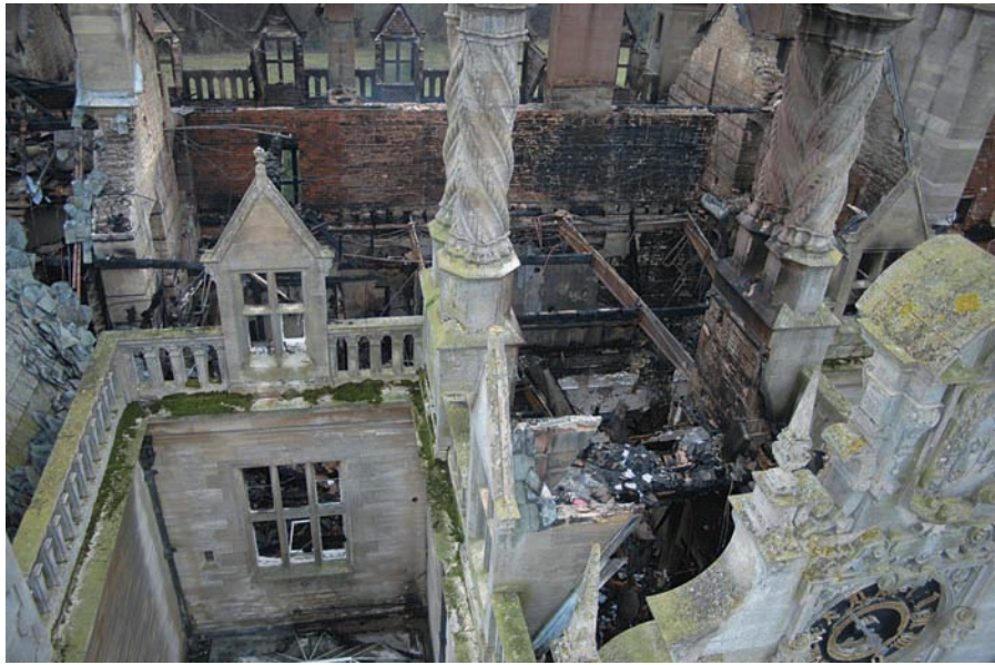
Figure 12.2 Grade I-listed Stoke Rochford Hall, now a residential conference centre, near Grantham, Lincolnshire, was partially destroyed by fire in January 2005. Good access is vital to effective firefighting to limit damage.
