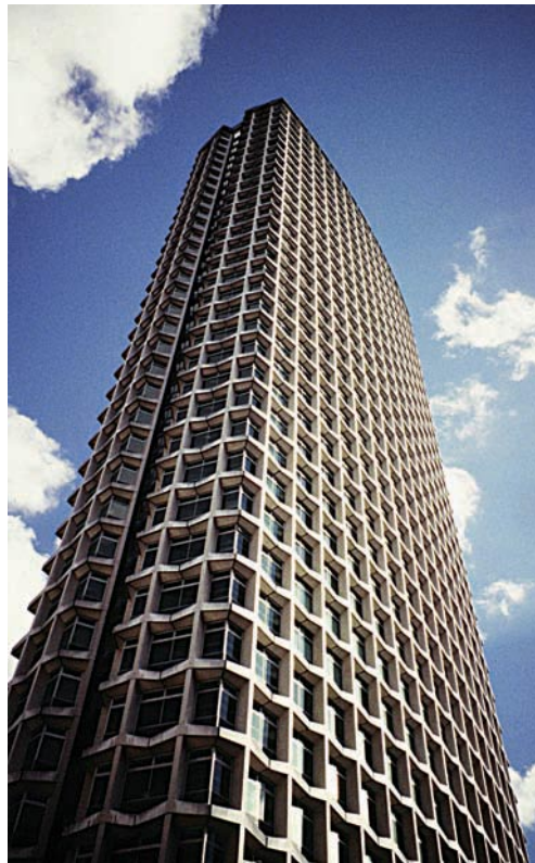
Figure 11.3 One of the more conspicuous additions to the skyline in the twentieth century was Centrepoint, London, 1962–67, by Richard Seifert.
