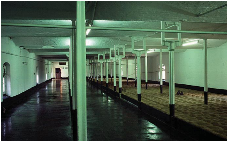
Figure 10.2 Ditherington Mill, Shrewsbury, Shropshire of 1797, the world's first iron-framed multi-storey building, using cast iron for both beams and its cruciform-section columns.
