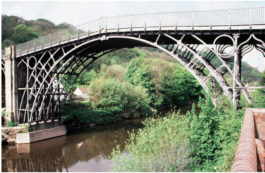
Figure 10.1 Iron Bridge, Shropshire across the River Sever, cast at the nearby Coalbrookdale Works in 1779.
