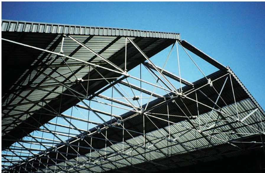
Figure 10.4 Roof over platforms at Huddersfield Station, West Yorkshire, completed in 1850.
