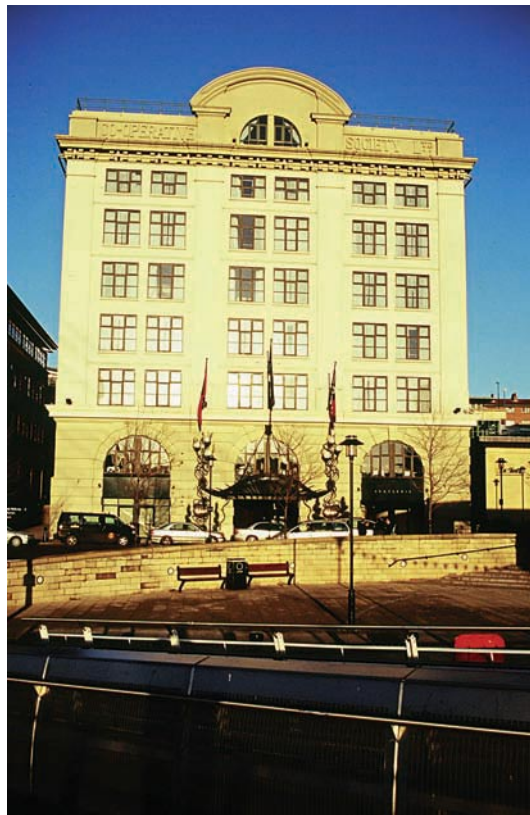
Figure 11.2 The Malmaison Hotel, Newcastle upon Tyne, built in 1901 as a warehouse for the Co-operative Wholesale Society, converted by Terry Farrell & Partners.
