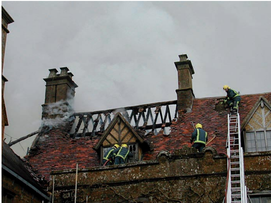
Figure 12.3 A devastating fire at the seventeenth century Wardington Manor, near Banbury, Oxfordshire, in 2004. The Manor contained Britain's greatest private collection of atlases, which was saved by villagers forming a human chain to pass the books to safety.
