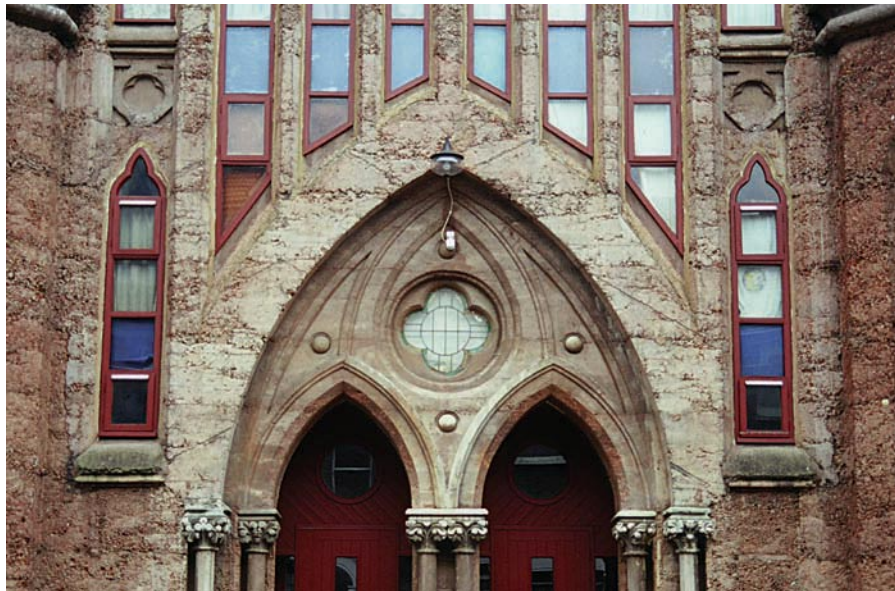
Figure 11.1 The neo-Gothic, unreinforced mass concrete Swedenborg Church, Waldegrave Road, south London, 1883, by W.J.E. Henley.
