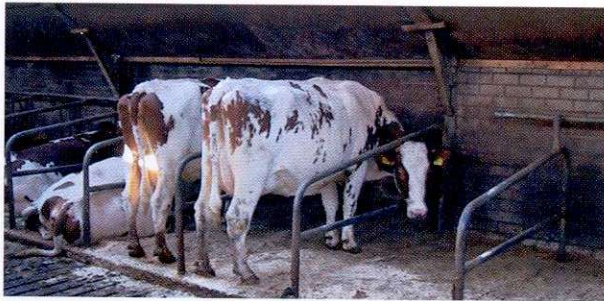
These cows have no headroom when lying down or standing up. There is a mark where the cows have hit the wall. Solution: lengthen the cubicle by demolishing the wall, leaving the front open to provide fresh air and better lighting, while taking measures to protect the bedding from driving rain.
