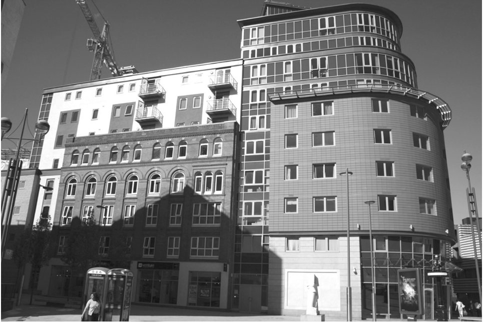
Figure 6.3 Postmodern architecture often borrows from past styles, but in this case, part of Birmingham's Orion Building, a section of terracotta Victoriana has been literally built into the new development. There has, however, been relatively little attempt made to integrate the old façade into the design of the new building.
