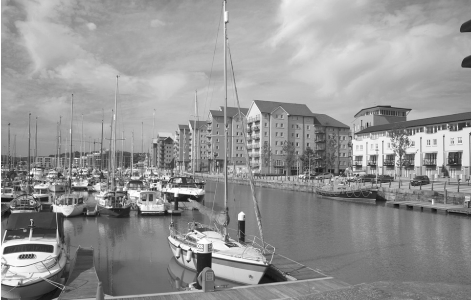
Figure 7.1 Though a large-scale development, Port Marine has created a very attractive and varied new waterfront for Portishead. This brownfield development is anchored by a Waitrose supermarket, giving some indication of the wealthier social demographic being targeted.
