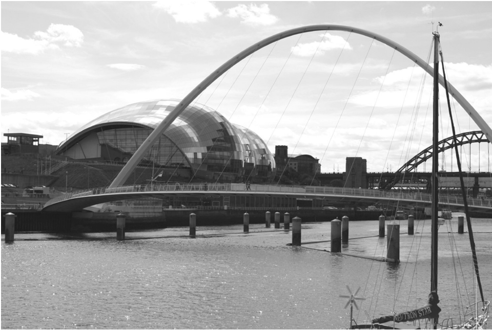
Figure 6.6 The Sage, Gateshead, designed by Foster and Partners, provides a striking outlook to those sitting in the riverside cafés on the Newcastle side of the Tyne.
