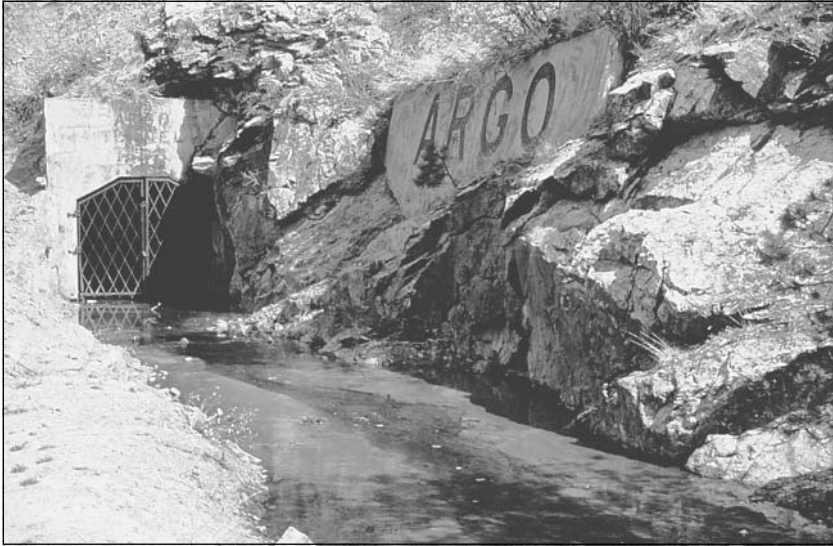
Contaminated water caused by mining in Idaho Springs, Colorado, in the early 1980's. (U.S. Geological Survey)
