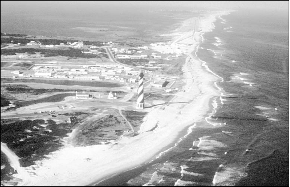
A groin built to protect the coastline of Cape Hatteras, North Carolina, traps sand that normally moves along the shoreline. (U.S. Geological Survey)
