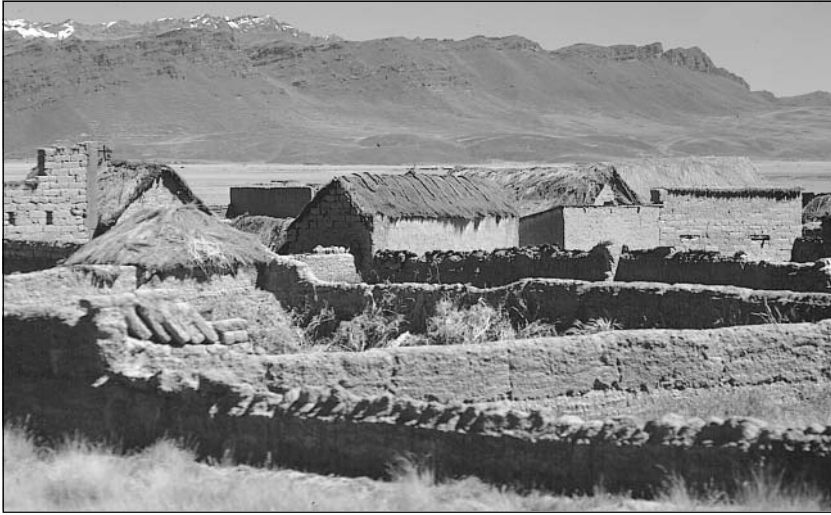
Buildings and walls made almost entirely from mud bricks in the South American Andes. (Clyde L. Rasmussen)
