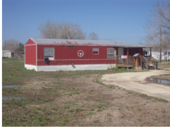
Fig. 15.5 Typical manufactured home (trailer) with “skirt”. Rancho Vista. (Note also the self constructed porch and steps rather than a ramp)
