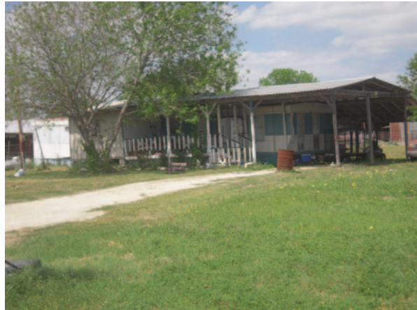
Fig. 15.6 Older—style manufactured (trailer) with self-built extensions, porch and false roof for shade, Rancho Vista
