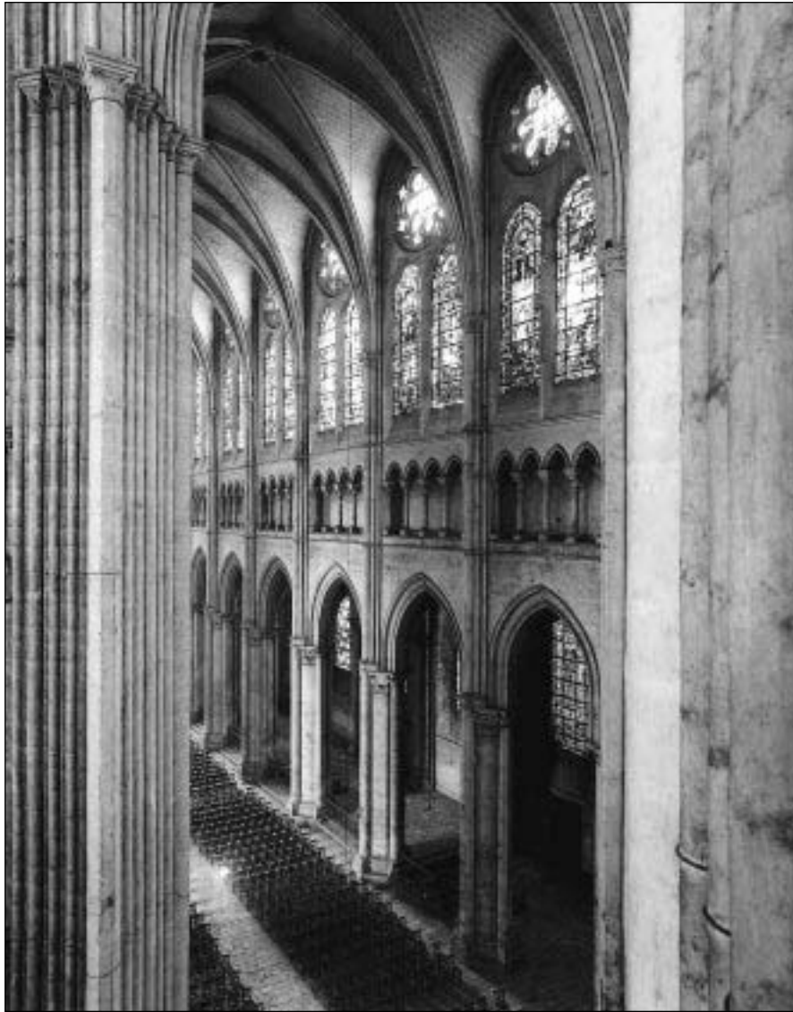
Fig. 3.1 Chartres Cathedral, France, twelfth and thirteenth centuries. The Gothic church incorporates most of the various forms for which masonry is suitable. Columns, walls and compressive form-active arches and vaults are all visible here. (Photo: Courtauld Institute)
