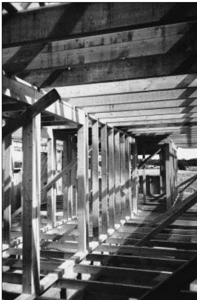
Fig. 3.6 The all-timber house is a loadbearing wall form of construction in which all of the structural elements in the walls, floors and roof are of timber. An internal wall of closely spaced sawn-timber elements is here shown supporting the upper floor of a two-storey building. Note temporary bracing which is necessary for stability until cross-walls are inserted. (Photo: A. Macdonald)
