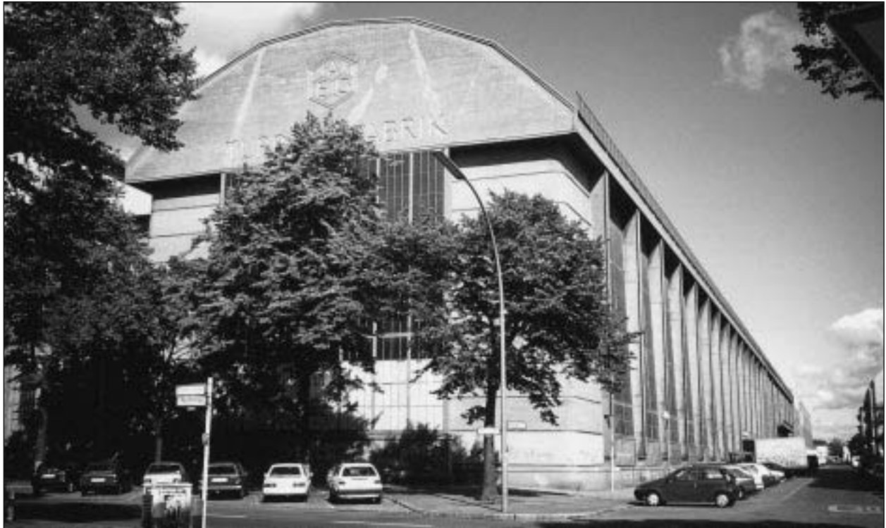
Fig. 7.3 AEG Turbine Hall, Berlin, 1908; Peter Behrens, architect. Glass and structure alternate on the side walls of this building and the rhythm of the steel structure forms a significant component of the visual vocabulary. Unlike in many later buildings of the Modern Movement the structure was used 'honestly'; it was not modified significantly for purely visual effect. With the exception of the hinges at the bases of the columns it was also protected within the external weathertight skin of the building. (Photo: A. Macdonald)
