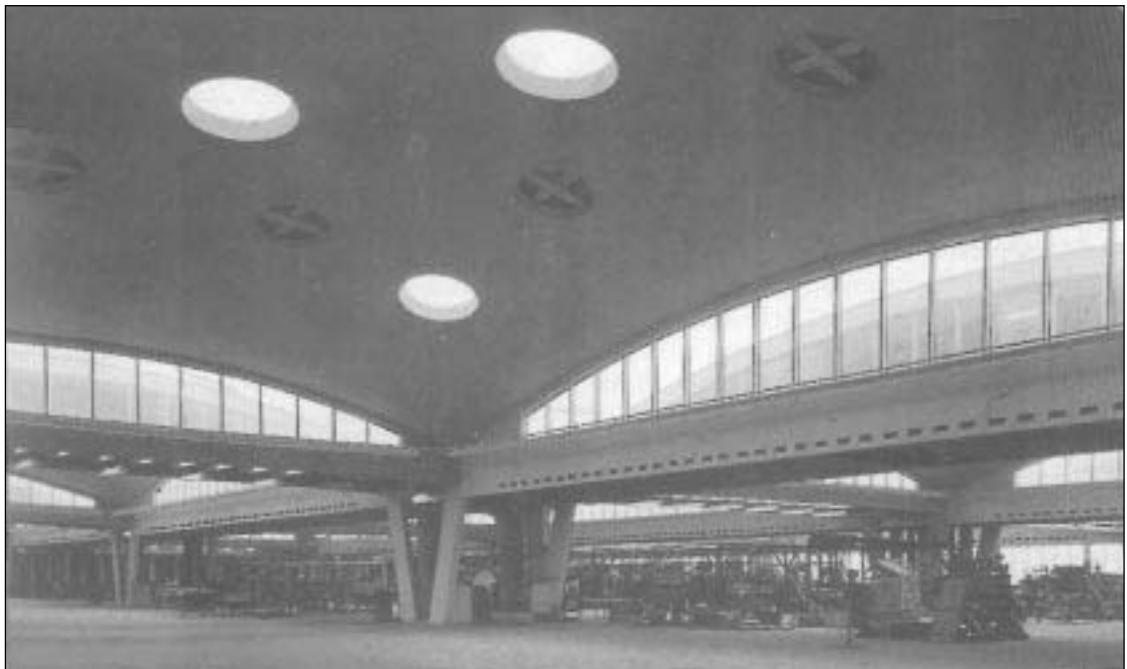
Fig. 5.25 Brynmawr Rubber Factory, Brynmawr, UK, 1952; Architects Co-Partnership, architects; Ove Arup & Partners, structural engineers. The principal enclosing elements here are compressive form-active, elliptical paraboloid shell roofs. (Photo: Architectural Review )
