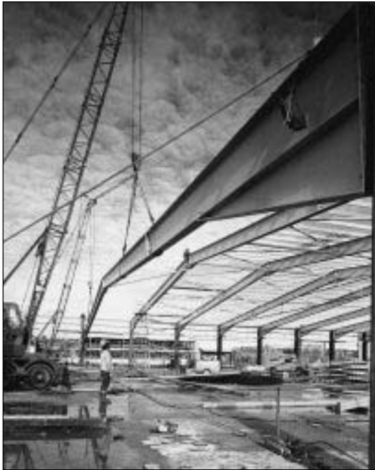
Fig. 5.20 The ubiquitous portal frame is a semi-form-active structure. The main elements in this example have 'improved' I-shaped cross-sections. (Photo: Conder)
