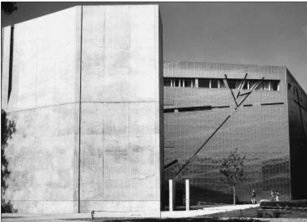
Fig. 7.42 Jewish Museum, Berlin, 1999; Daniel Libeskind Architekturburo, architects. The use of a reinforced concrete structural framework has allowed both a highly sculptured overall form to be created and a high degree of freedom to be achieved in the treatment of the non-structural cladding of the exterior.
