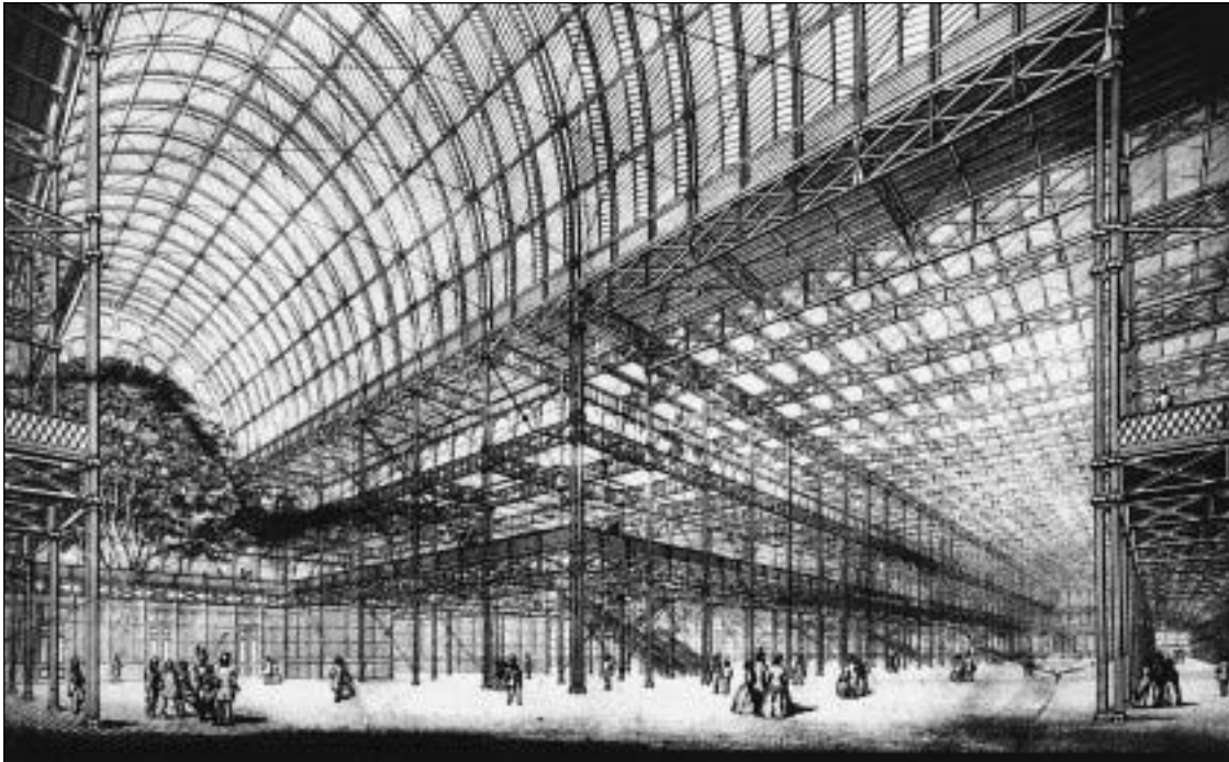
Fig. 7.25 Crystal Palace, London, UK, 1851; Joseph Paxton, architect/engineer. The Crystal Palace was a truly high-tech building and an inspiration to generations of modern architects. Unlike many twentieth-century buildings to which the label High Tech has been applied, it was at the forefront of what was technically possible at the time. The major decisions affecting the form of the building were taken for technical reasons and were not compromised for visual or stylistic effect. The building has technical shortcomings, such as the poor durability of the many joints in the external skin, but in the context of a temporary building it was appropriate that these were given a low priority.
