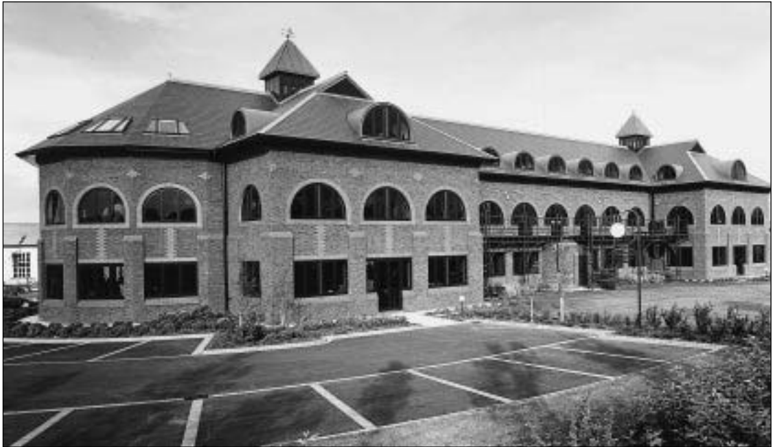
Fig. 5.6 Corinthian Court, Abingdon, UK; the Baron Willmore Partnership, architects; Glanville and Associates, structural engineers. The vertical structure of this three-storey office building, which measures 55 m by 20 m on plan and has few internal walls, is of loadbearing masonry. The floors are of reinforced concrete.
