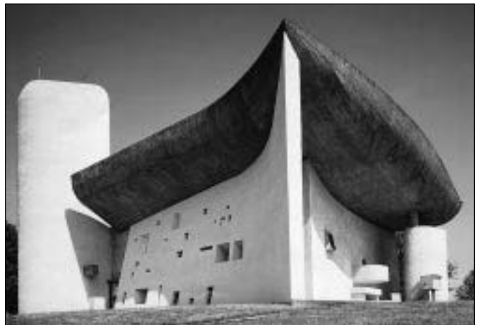
Fig. 7.40 Notre-Dame-du-Haut, Ronchamp, France, 1954; Le Corbusier, architect. Structural considerations have played very little part in the determination of the form of this building. Its small scale together with the excellent structural properties of reinforced concrete, which was used for the roof, meant that it could be constructed without difficulty. (Photo: P. Macdonald)
