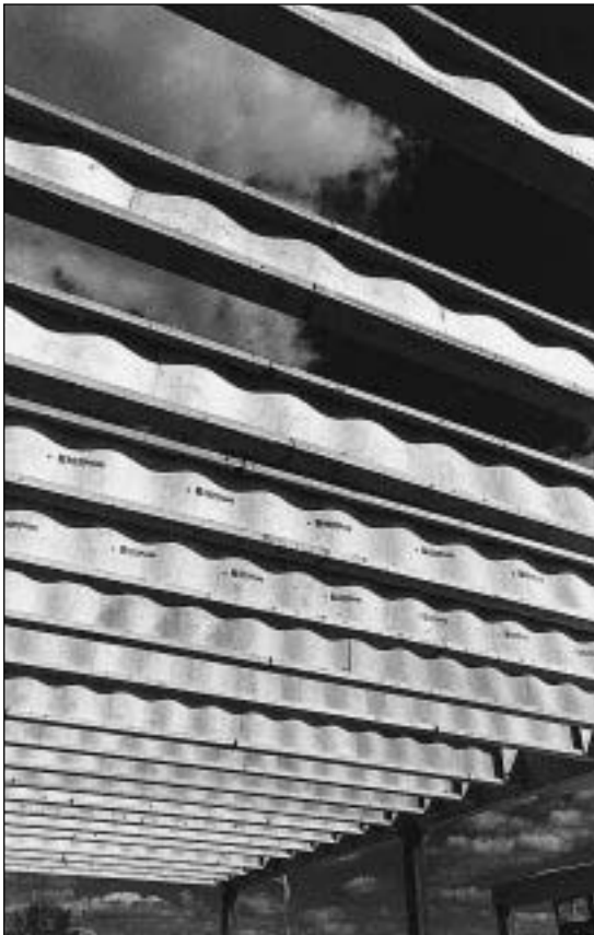
Fig. 3.11 Built-up-beams with I-shaped cross-sections consisting of sawn timber flanges connected by a plywood web. The latter is corrugated which allows the necessary compressive stability to be achieved with a very thin cross-section. (Photo: Finnish Plywood International)
