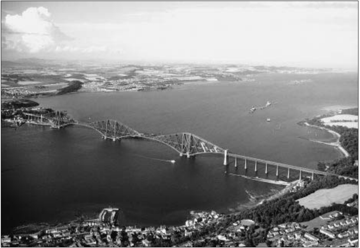
Fig. 6.6 Basic structural arrangement of the Forth Railway Bridge, Firth of Forth, UK. This structure is a post-and-beam framework but, as with the Renault Headquarters (Figs 3.19 & 6.8), it has been 'improved' at various levels. There is more justification for the complexity in this case due to the large span involved. (Photo: A. & P. Macdonald)
