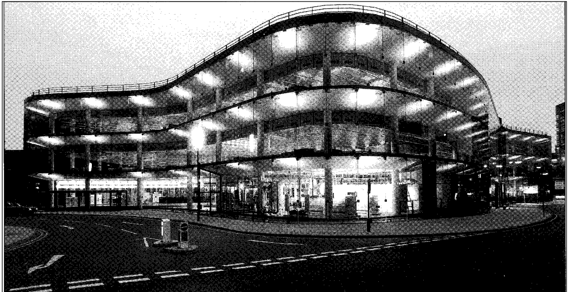
Fig. 7.37 Willis, Faber and Dumas Office, Ipswich, UK, 1974; Foster Associates, architects; Anthony Hunt Associates, structural engineers. This building may be considered to be a late Modern equivalent of the Villa Savoye (Fig. 7.34). The relationship between structure, space planning and visual treatment is similar in both buildings. (Photo: John Donat)
