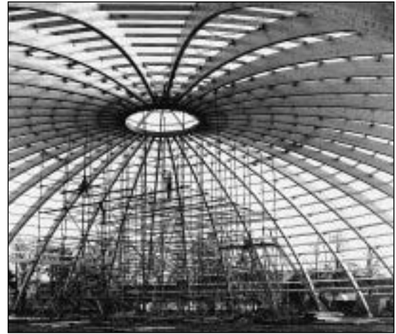
Fig. 3.9 Sports Dome, Perth, Scotland, UK. Laminated timber built-up sections can be produced in a variety of configurations in addition to straight beams. Here a series of arch elements is used to produce the framework of a dome.
