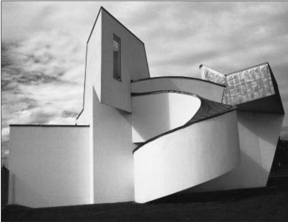
Fig. 7.41 Vitra Design Museum, Basel, Switzerland, 1989; Frank Gehry, architect. From a technical point of view forms such as this present a challenge. Their construction is made possible by the excellent structural properties of present-day materials such as reinforced concrete and steel. The scale of such a project must be small however. (Photo: E. & F. Mclachlan)
