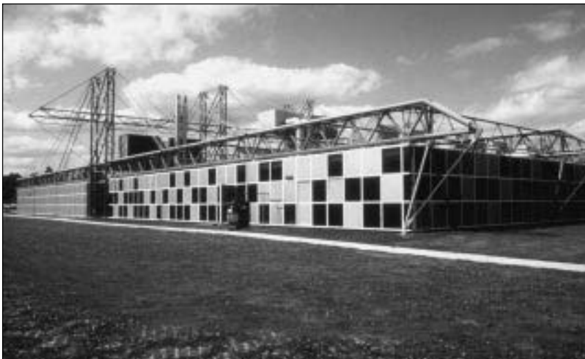
Fig. iv Inmos Microprocessor Factory, Newport, South Wales, 1982; Richard Rogers Partnership, architects; Anthony Hunt Associates, structural engineers. The general arrangement and appearance of this building were strongly influenced by the requirements of the exposed structure. The form of the latter was determined by space-planning requirements. (Photo: Anthony Hunt Associates)
