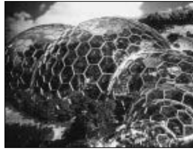
Fig. 7.54 The Eden Project, Cornwall, UK, 1999; Nicholas Grimshaw and Partners, architects; Anthony Hunt Associates, structural engineers. The complexity of form made possible by computer-aided design has brought into being a new generation of metal and glass structure.
