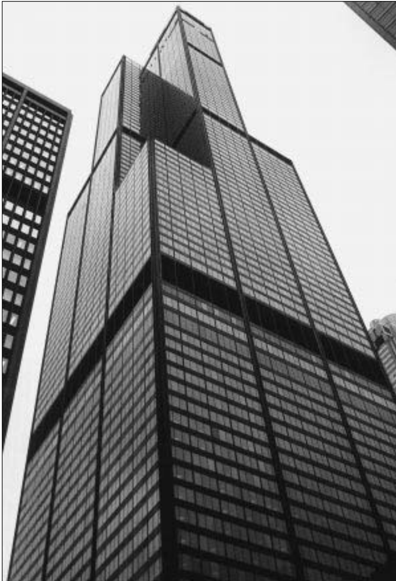
Fig. 7.22 Sears Tower, Chicago, USA, 1974; Skidmore, Owings and Merrill, architects and structural engineers. This building, which is currently the tallest in the world, is subdivided internally by a cruciform arrangement of 'walls' of closely spaced columns which enhance its resistance to wind loading. This structural layout is expressed in the exterior form.
