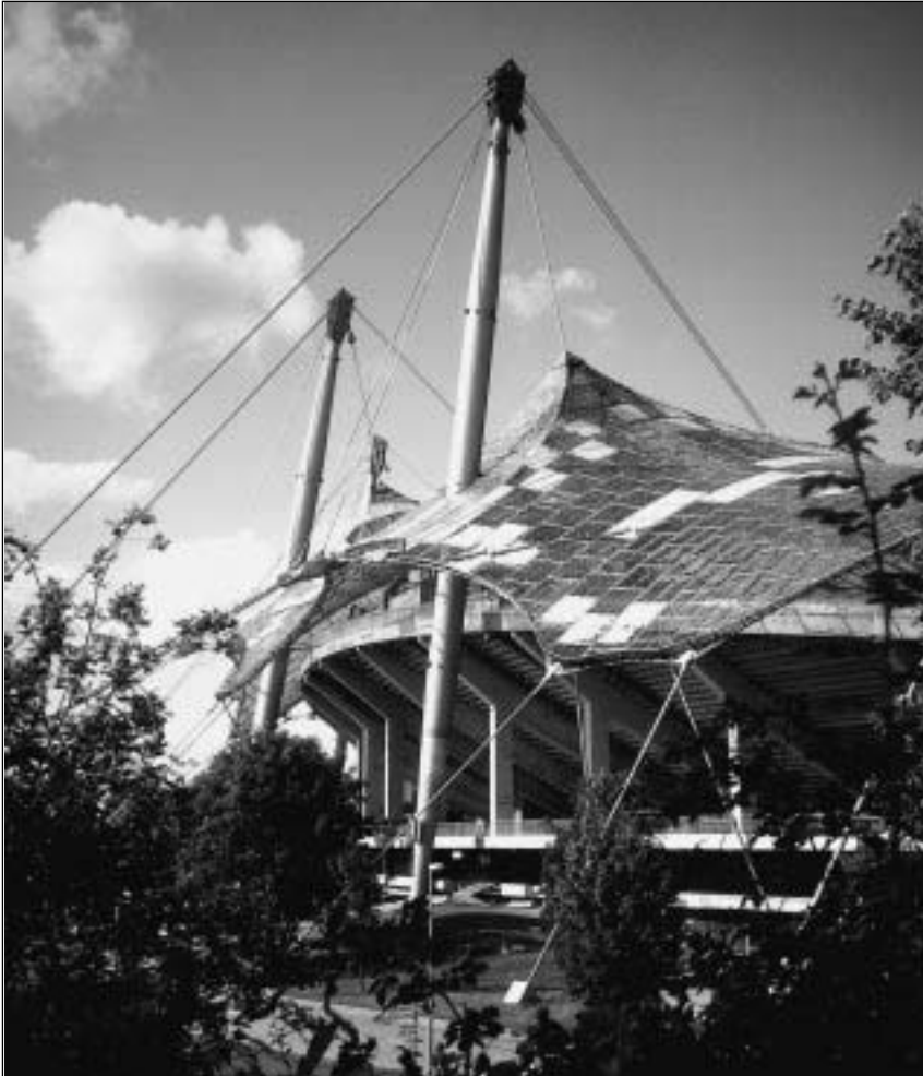
Fig. i Olympic Stadium, Munich, Germany, 1968–72; Behnisch & Partner, architects, with Frei Otto. In both the canopy and the raked seating most of what is seen is structural. (Photo: A. Macdonald)
