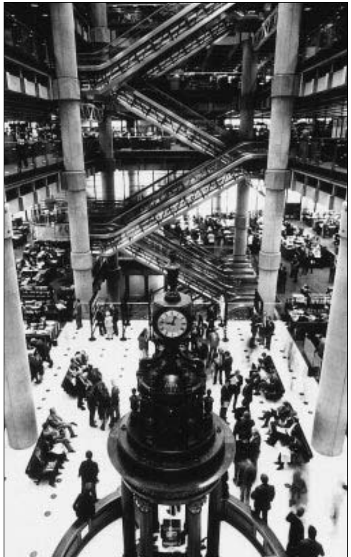
Fig. 7.12 Atrium, Lloyds headquarters building, London, UK, 1986; Richard Rogers and Partners, architects; Ove Arup & Partners, structural engineers. The columns are set outside the perimeter of the floor decks and connected to them through visually prominent pre-cast concrete brackets. The arrangement allows the structure to be easily 'read' but is far from ideal structurally. It introduces bending into the columns, which causes high concentrations of stress at the junctions.
