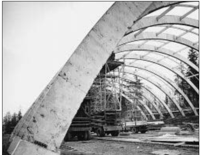
Fig. 3.12 Sports Stadium at Lähderanta, Sweden. The primary structural elements are plywood timber arches with rectangular box cross-sections. (Photo: Finnish Plywood International)
