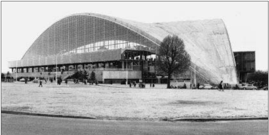
Fig. 1.4 Exhibition Hall of the CNIT, Paris, France; Nicolas Esquillan, architect. The principal element is a self-supporting reinforced concrete shell.
