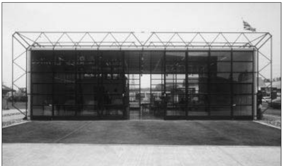
Fig. 7.26 Patera Building; Michael Hopkins, architect; Anthony Hunt Associates, structural engineers. The building consists of a lightweight steel framework which supports an insulated cladding system and fully glazed end walls. The principal structural elements are external and the purlins and cladding rails are located within the cladding zone to give a very clean interior. (Photo: Anthony Hunt Associates)
