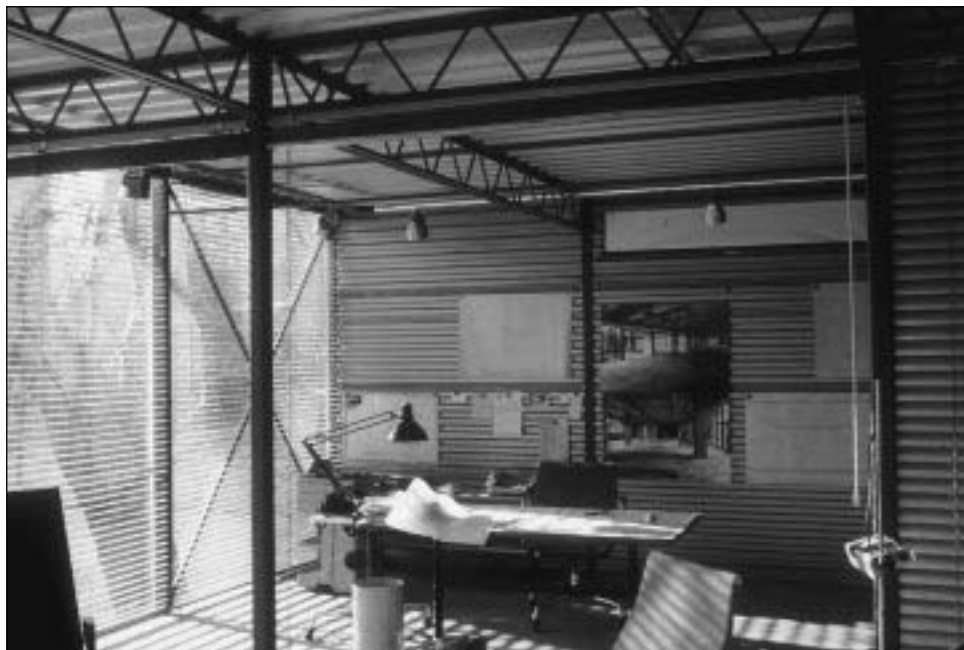
Fig. 6.5 Hopkins House, London, UK, 1977; Michael Hopkins, architect; Anthony Hunt Associates, structural engineers. The very short spans involved here would not normally justify the use of complex triangulated elements for the horizontal structure. Ease and speed of erection were the main technical reasons for their selection. The visual excitement which they produce was, nevertheless, the principal reason for their adoption. (Photo: Anthony Hunt Associates)
