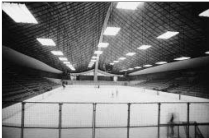
Fig. 7.18 David S. Ingalls ice hockey rink, Yale, USA, 1959; Eero Saarinen, architect; Fred Severud, structural engineer. A combination of compressive form-active arches and a tensile form-active cable network was used in this long-span building. The architecture is totally dominated by the structural form.
