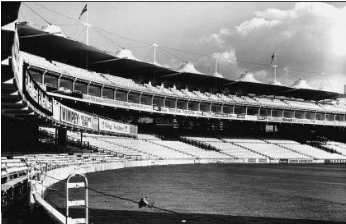
Fig. 5.23 Grandstand at Lord's Cricket Ground, London, UK, 1987; Michael Hopkins & Partners, architects; Ove Arup & Partners, structural engineers. The canopies which form the roof of this building are form-active tensile membranes.
