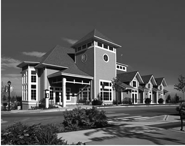
Figure 2.4 Blakely Hall is a Community Center and town hall for Issaquah Highlands, a planned community near Seattle, Washington. It consists of 7000 sq. ft. and built to a budget of US $1,500,000. It is used mainly as a meeting place for numerous clubs and groups at Issaquah Highlands. Blakely Hall is the first building in the United States to earn a Green Globes Certification (earned two Globes out of four possible) as well as a LEED Silver award.
