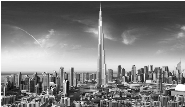
Figure 1.7 Illustration of Burj Khalifa, Dubai which was inaugurated on January 4, 2010. Burj Khalifa is currently the tallest skyscraper in the world in all three categories recognized by the Council on Tall Buildings and Urban Habitat (CTBUH), the world leading authority which compiles and ranks the world's tallest buildings. CTBUH ranks buildings on the basis of height to architectural top, highest occupied floor and height to tip. Burj Khalifa, was designed by the Chicago office of Skidmore, Owings & Merrill LLP (SOM) and constructed by Samsung/BESIX/Arabtec Corporation for Emaar properties, UAE. Turner Construction International was the project and construction manager. The height of the completed tower is 2717 feet (828 m) and built at a cost of about $1.5 billion. It reportedly contains 160 habitable floors, 57 elevators, apartments, shops, swimming pools, spas, corporate suites, Italian fashion designer Giorgio Armani's 160 room hotel, and an observation platform on the 124th floor. Source: Skidmore, Owings & Merrill.
