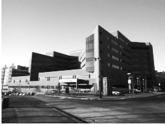
Figure 11.5 Photo of the Cee hospital, a nine-story, 600,000 square feet acute care facility in Minneapolis, MN which recently underwent recommissioning (ReCx). The first floor was built in 1981, and the rest of the floors were added in 1982. The owner's objective in recommissioning the building was to reduce operating costs while maintaining or improving IAQ and comfort. For this project, CEE partnered with the Energy Systems Lab at Texas A&M University, which is considered to be the most experienced and effective healthcare recommissioning provider in the US. Source: Center for Energy and Environment.
