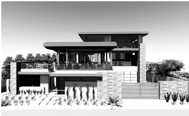
Figure 2.14 Photo showing NAHB documenting the New American Home 2016 as it goes through each stage of the construction process. This image reflects America’s premier show home!
