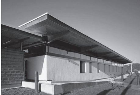
Figure 2.3 (a) The Santa Clarita Transit Maintenance is one of the first LEED Gold-certified straw-bale buildings in the world. The resource- and energy-efficient transit facility was designed by HOK and exceeds California Energy Efficiency Standards by more than 40%, securing a new standard for straw-bale in high-performance building design. (b) Diagram shows section taken through exterior wall of transit facility. The designers reportedly opted for a solar photovoltaic canopy to shade buses and provide nearly half of the building's annual energy needs. An electronic monitoring system is in place to track thermal comfort, energy efficiency, and moisture levels. Source: HOK Architects.
