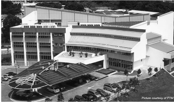
Figure 2.12 The PTM Green Energy Office Building (GEO Building) is Malaysia's first GBI-certified green building and is designed as an administration-cum-research office for Pusat Tenaga Malaysia (Malaysia Energy Centre). The GEO building is built on a 5-acre site in Seksyen 9, Bandar Baru Bangi, Selangor, Malaysia. It is among the first Malaysian Government office buildings whose design is based on green concepts and is environmentally friendly. Source: PTM-GreenBuildingIndex.
