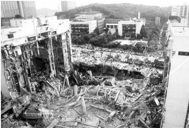
Figure 16.3b View of the Sampoong Department store building after its collapse. The building is located in the Seocho-gu district of Seoul, South Korea. There were more than 1500 people in this luxury department store in Seoul, South Korea, when a section of the five-story building collapsed in which more than 500 people were killed. The collapse of the building, which was constructed using steel-reinforced concrete pillars, was blamed on faulty construction.
