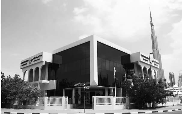
Figure 2.13 Photo depicting the Dubai Electricity and Water Authority (DEWA) Headquarters in the UAE which received a LEED Platinum certification. DEWA's green features help the building reduce consumption of energy by 66% and water by 48%. Additionally, 36% of construction material used was recycled content. DEWA was founded on January 01, 1992 by Sheikh Maktoum bin Rashid Al Maktoum. After using conventional gas-fired power plants since it was founded, DEWA recently added solar power to its energy mix.
