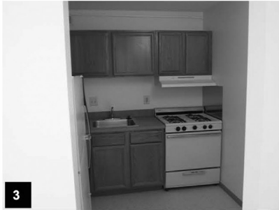
3 Interior – View of Kitchen of Unit 1120 on the eleventh floor of the ABC Apartments. Apartment unit is complete and ready for hand over.
