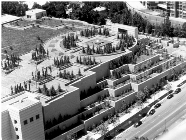
Figure 6.6 Example of a 70,000-square-foot vegetated roof on the LDS Assembly Hall building, Salt Lake City, UT. Source: American Hydrotech, Inc.
