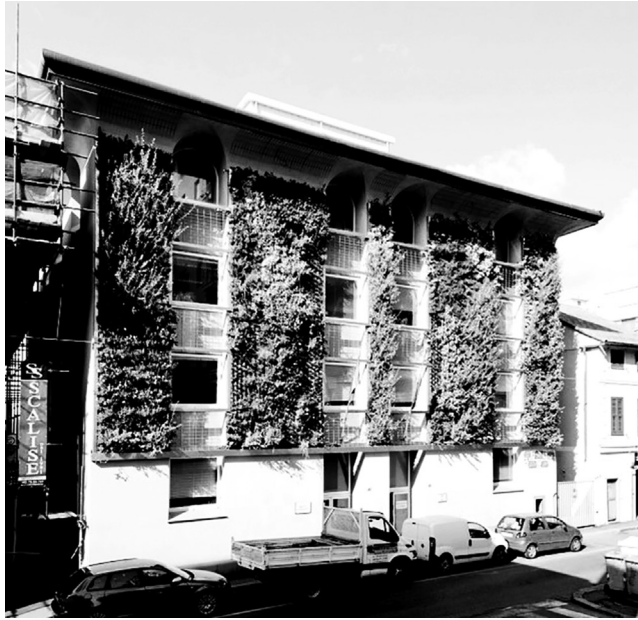
Figure 10.5 Photo of building in Italy with “green façade” showing the benefits of vertical vegetation on exterior walls. There are two types of green facades: (1) that utilize climbing plants or plants secured by a trellis and contain enough soil to support the plants; and (2) living wall systems constructed of thin panels on an artificial growing medium such as felt or mineral wool, that need nutrients and water. Photo: Anna Positano.
