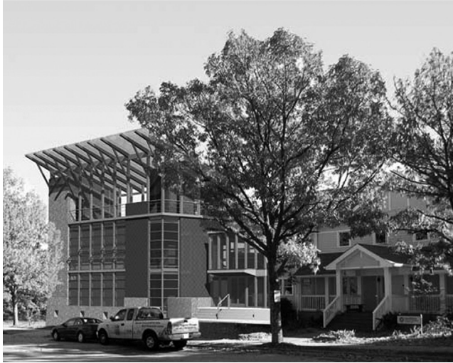
Figure 8.1 The new Eco Office in Atlanta, Georgia is a 10,000 square feet. facility seeking LEED-Platinum rating, which was designed as a model for environmentally responsible commercial construction that is achievable utilizing existing off-the-shelf materials and technology. The new Eco Office provides a showcase of state-of-the-art energy, water, and waste-reducing features.
