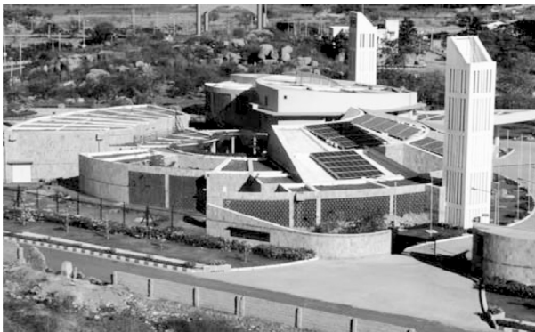
Figure 2.10 The Sohrabji Godrej Green Business Centre in Hyderabad, India. This was the first Platinum-rated green building under the LEED rating system, outside the United States, boasting Energy Savings of 63%. Source: Confederation of Indian Industry.
