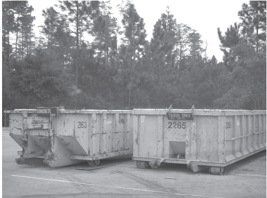
Figure 7.7 Separating waste on-site is one method to comply with the construction waste management strategies to avoid using landfills and incineration facilities.
