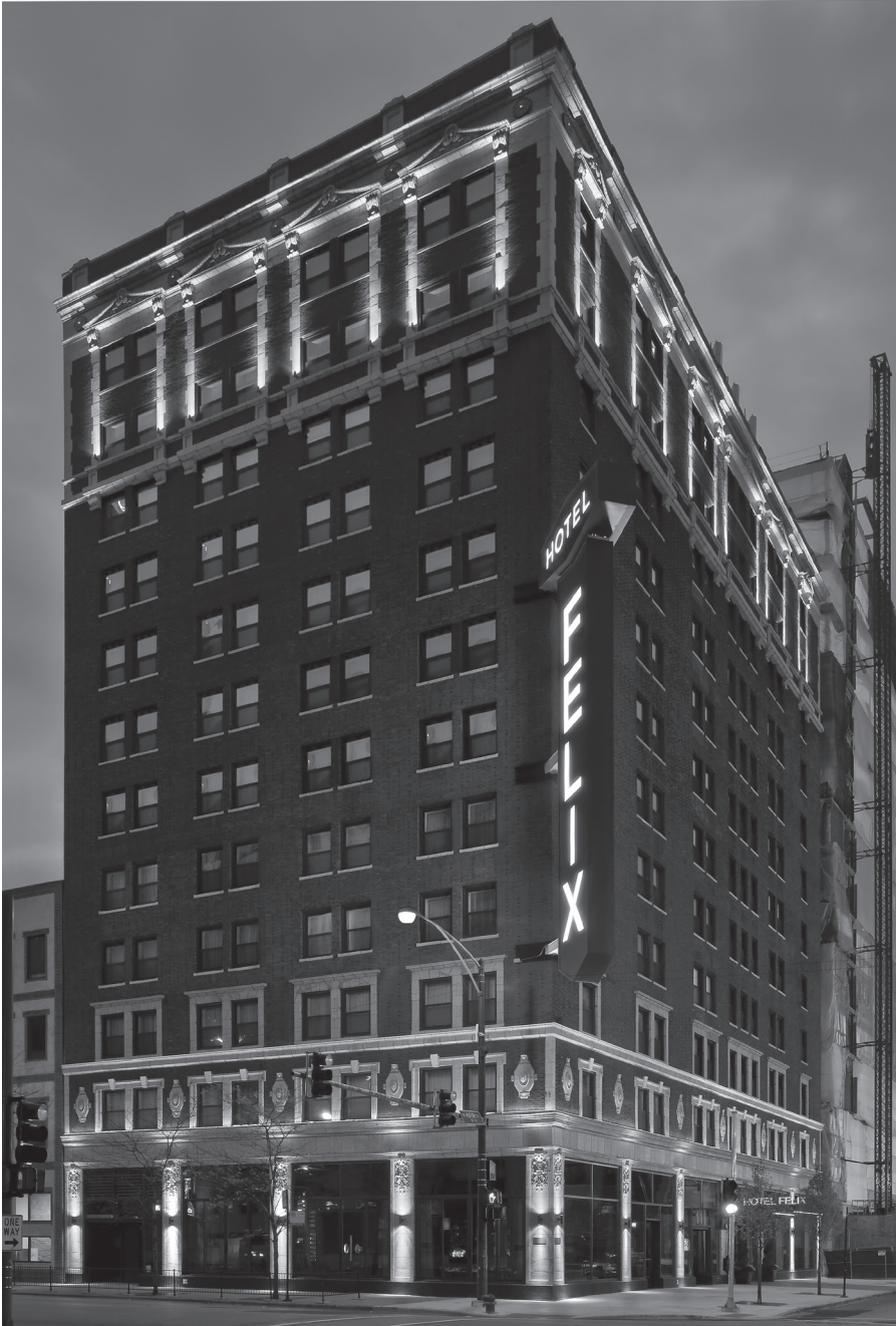
Figure 4.20 Gettys Hotel Felix in Chicago, designed by Gettys, successfully earned LEED CI Silver certification; its urban location helped earn the project SS Credits 2 and 3. Photo courtesy of Gettys
