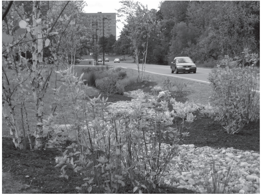
Figure 4.5 Bioswales, an on-site filtration strategy, can help to recharge the groundwater and reduce stormwater runoff. Photo courtesy of Thomas M. Robinson, EDR
