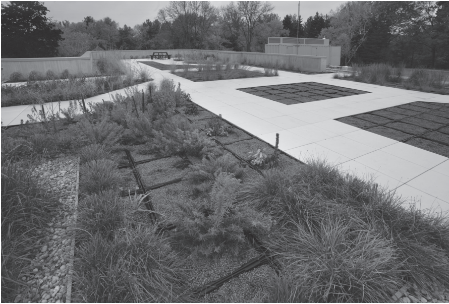
Figure I.1 Holy Wisdom Monastery project in Madison, Wisconsin, by Hoffman, LLC, reduces the amount of stormwater runoff from the site, increases the amount of open space, promotes biodiversity, reduces cooling loads, and reduces the impacts of the urban heat-island effect by implementing a vegetated roof.
