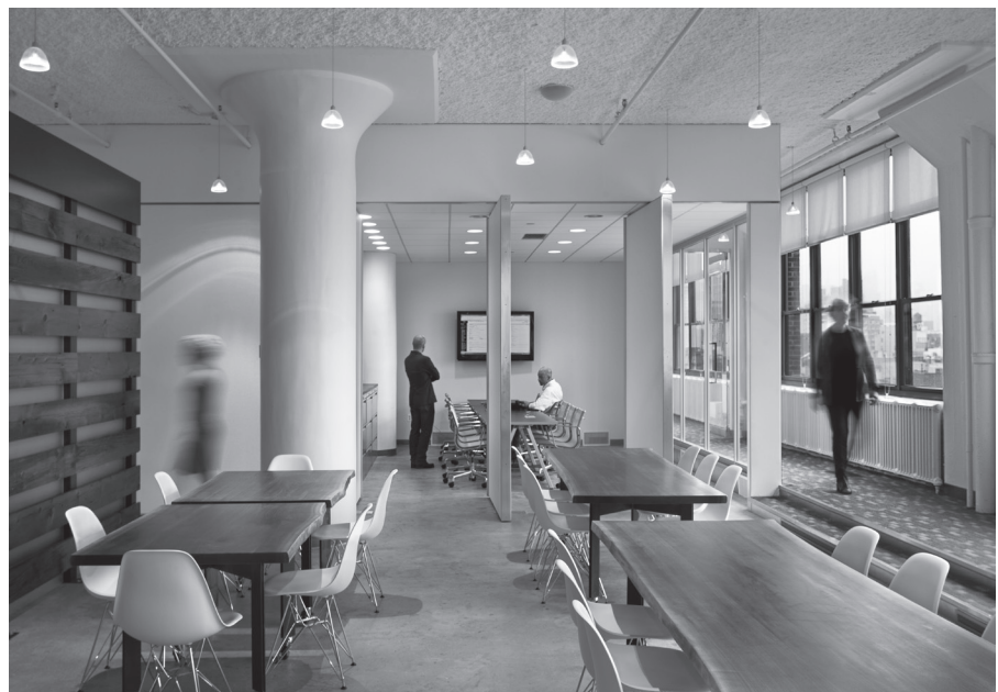
Figure 8.13 The lighting design at The National Audubon Society project in New York designed by Illumination Arts and FXFOWLE Architects includes simple downlights and wallwashers in the conference rooms where both were separately controlled by dimmers, thus allowing the occupants to adjust the lighting to fit their needs and the task at hand. Notice too the glare control strategy at the window. These types of strategies helped to earn the project its LEED CI Platinum level certification. Photo courtesy of FXFOWLE Architects and David Sundberg/Esto
