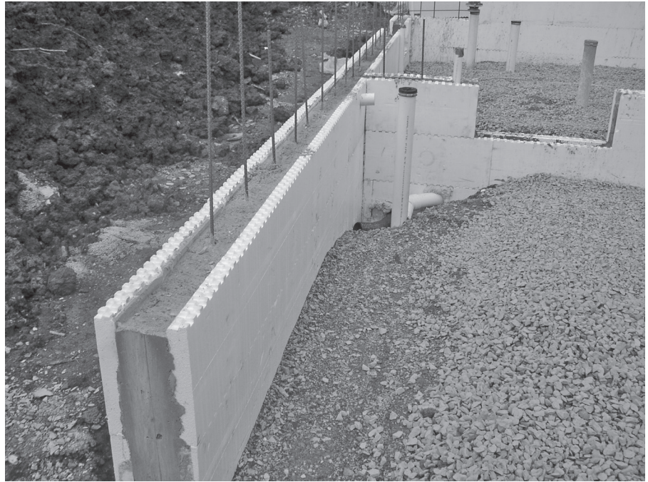
Figure 6.7 Selecting insulated concrete forms (ICFs) as a building envelope material can increase the performance of a building. Photo courtesy of Moshier Studio
