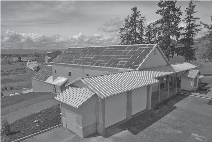
Figure 4.18 Stoller Vineyards in Dayton, Oregon, generates electricity on site by the means of photovoltaic panels mounted on the roof. Photo courtesy of Mike Haverkate, Stoller Vineyards
