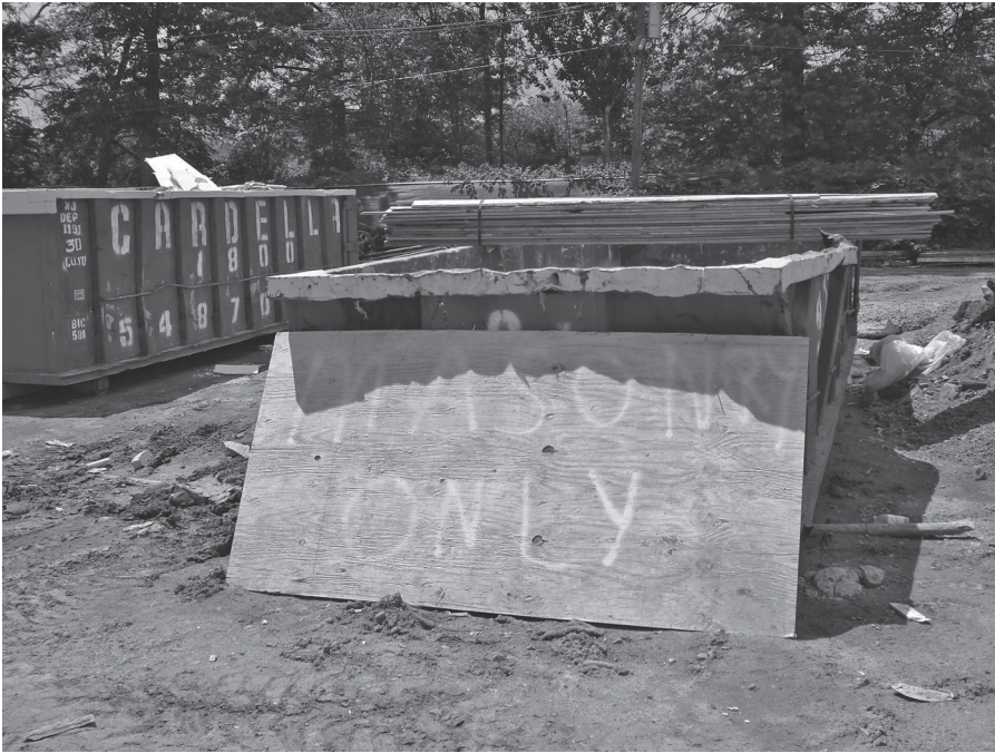
Figure 7.8 Dedicated waste container for masonry to be collected for recycling.
