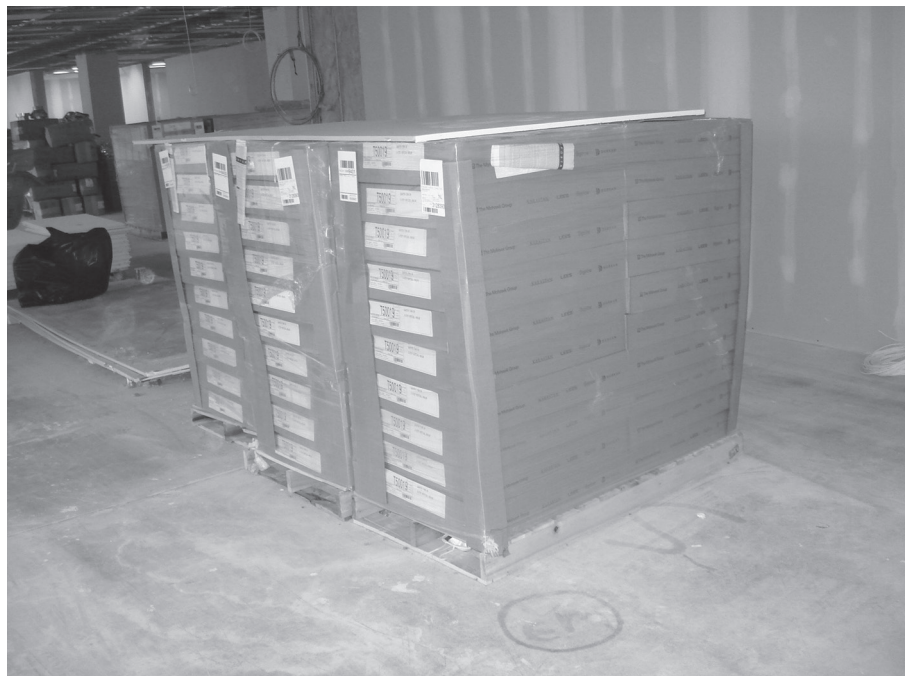
Figure 8.6 Elevating product storage protects against damage as suggested by SMACNA guidelines.
