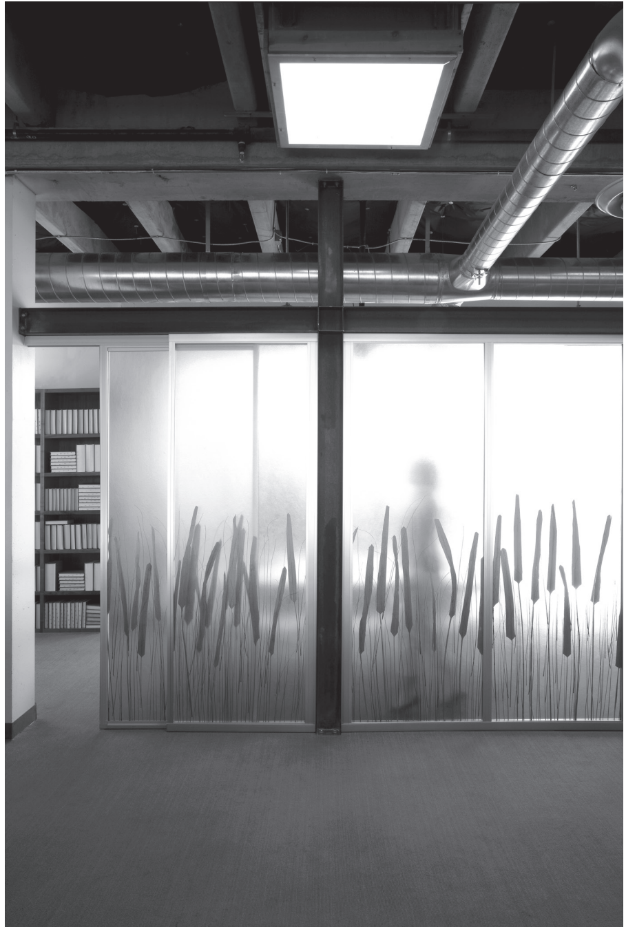
Figure 7.1 Specifying green materials, such as these 3Form® panels with recycled content, is a strategy to reduce the detrimental impacts of construction and the need for virgin materials. Photo courtesy of Skylar Nielson, 3Form
