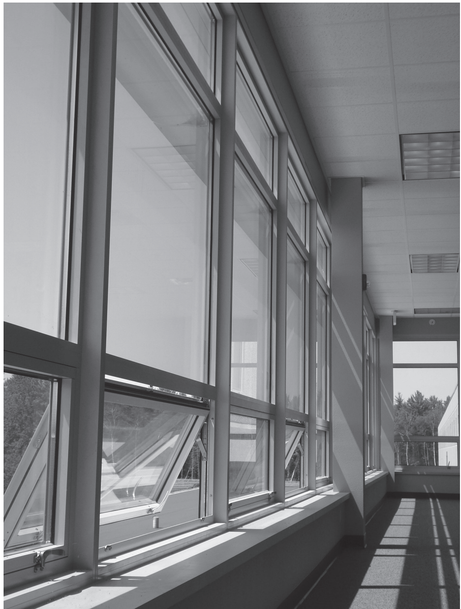
Figure 8.9 Wausau's LEED Silver facility in Wausau, Wisconsin, employs operable windows to give their employees access to fresh air. Photo courtesy of Wausau Windows and Wall Systems
