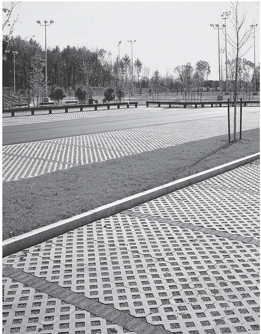
Figure 4.9 Turfstone™ Open-Grid Pavers allow stormwater to pass through and encourage vegetation growth between each open cell, in order to recharge groundwater and reduce runoff. Photo courtesy of Ideal
