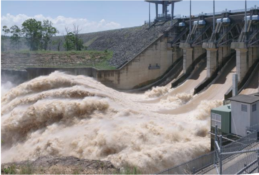
Figure 7.1. Air bubble entrainment on the Wivenhoe Dam spillway (Qld, Australia) on 17 January 2011.
