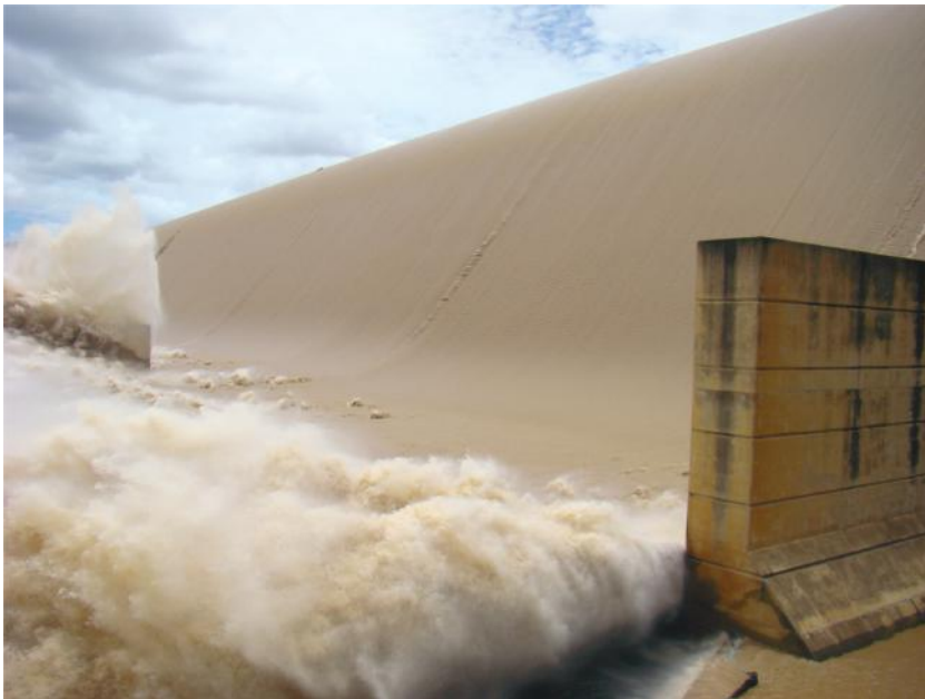
Figure 7.2. Air bubble entrainment downstream of Burdekin Falls Dam (Qld, Australia) in February 2009 (Courtesy of Queensland Department of Environment and Mineral Resources (DERM, Dam Safety) and David Li) – Looking upstream at the chute flow and aerated jet formation at spillway toe – Note the “brownish” dark colour of the flow caused by the suspended load and the “white” waters downstream of the spillway toe highlighting the air bubble entrainment.
