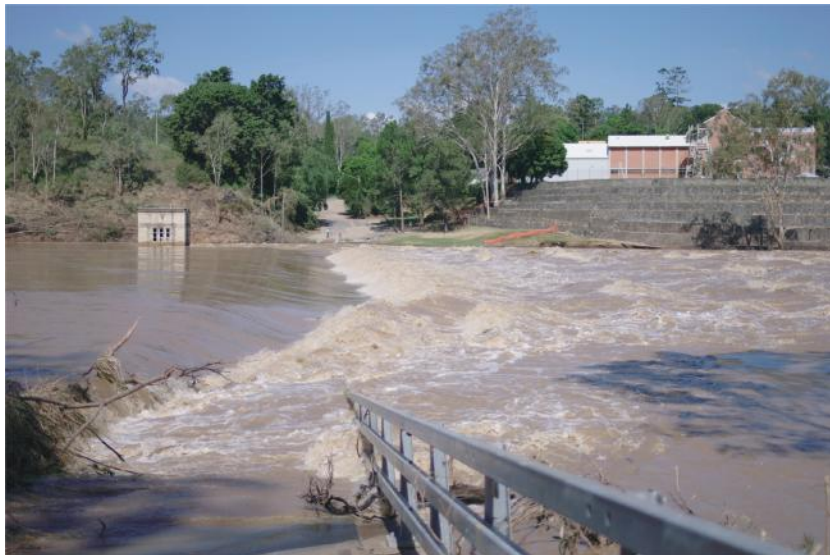
Figure 7.3. Free-surface aeration during the overtopping of Mount Crosby weir and bridge (Qld, Australia) on 17 Jan. 2011 – Flow direction from left to right.
