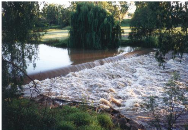
(C) Hydraulic jump downstream of Moree weir (NSW, Australia) on 16 December 1997 during some runoff – Flow from top left to bottom right.
