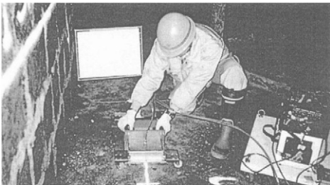
Photograph 2. Antenna and control unit
