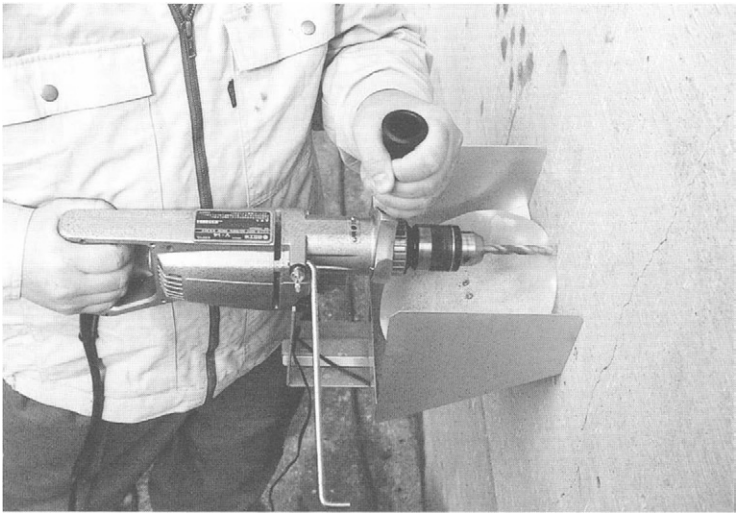
Photo 4 The neutralization depth test using drilled powder for only one engineer
