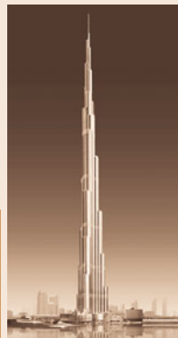
Figure E2.2 (Figure courtesy of Emaar Properties, Dubai, UAE.)
