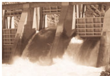
(Photograph courtesy of Pend Oreille Public Utility District.)
