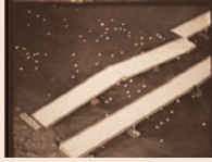
V10.10 Big Sioux River Bridge collapse
