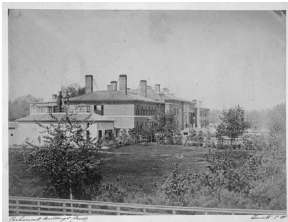
Figure 10.7 Parliament Buildings (front), Toronto, C.W., 1856–57; photograph by Armstrong, Beere & Hime, courtesy of National Archives of Canada, PA-186726.
