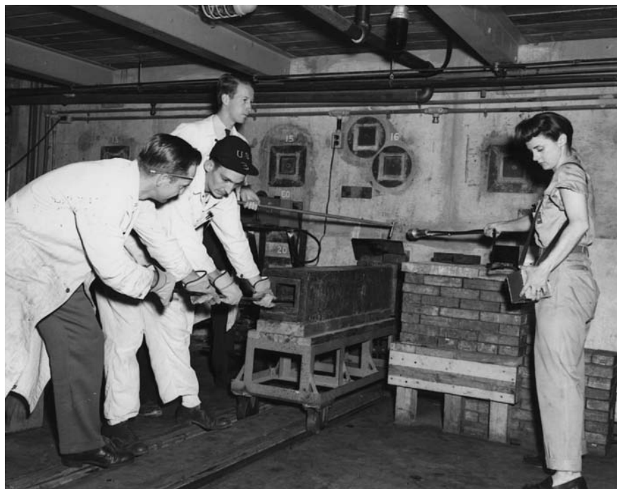
Figure 10.1 Unloading of an irradiated sample from the Oak Ridge reactor. Original caption reads: 'Removal of radioactivated sample from the pile after a neutron bombardment. Here Dr Ralph Overman, with a long holder, removed a bombarded sample from the carrier block which has been pulled from the pile. Mrs Weber measures the sample's radioactive strength to check on the safety of handling it. The carrier block is pulled into a lead shield to protect the workers from the radiation of the other samples in the carrier'. X-10, Clinton Laboratories, 14 June 1946. Source: US Army Photograph. Courtesy National Archives, photograph no. 433-OR-box 22-MED-308.
