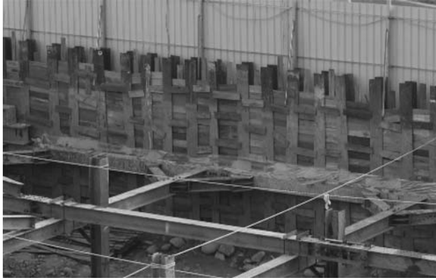
Figure 6.3 Soldier pile wall and its lateral support system. (Courtesy of An-Bin Huang, Hsinchu, Taiwan.)
