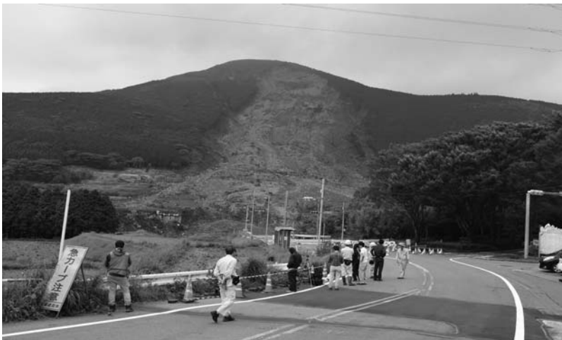
Figure 9.4 Landslide triggered by the 2016 Kumamoto earthquake in Kyushu, Japan. (Courtesy of Prof. Takaji Kokusho, Tokyo, Japan.)
