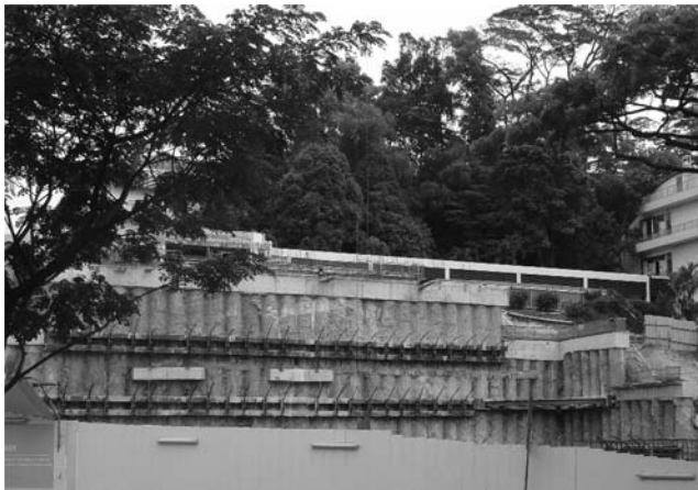
Figure 6.10 Braced excavation at National University of Singapore campus using contiguous-bored concrete piles with tieback support. (Courtesy of An-Bin Huang, Hsinchu, Taiwan.)
