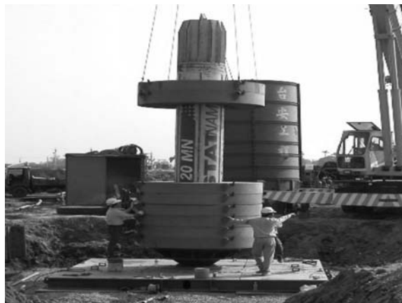
Figure 8.45 Field setup of the Statnamic load test. (Courtesy of DECL, Taipei, Taiwan.)
