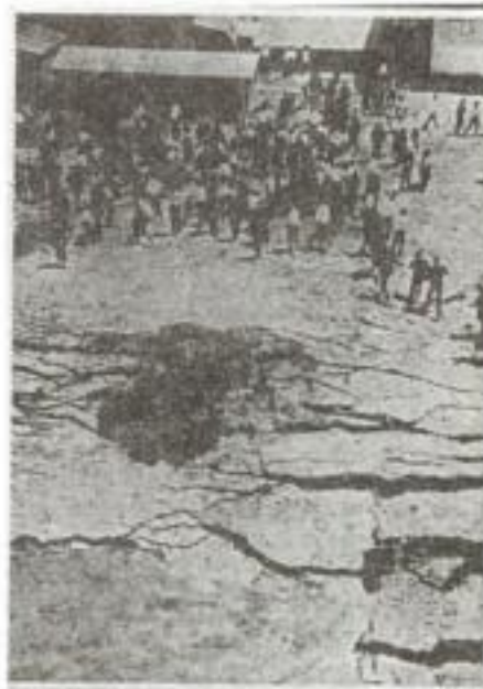
Fig. 13.6 Liquefaction in Niigata earthquake, 1964 (Ohsaki, 1966).
