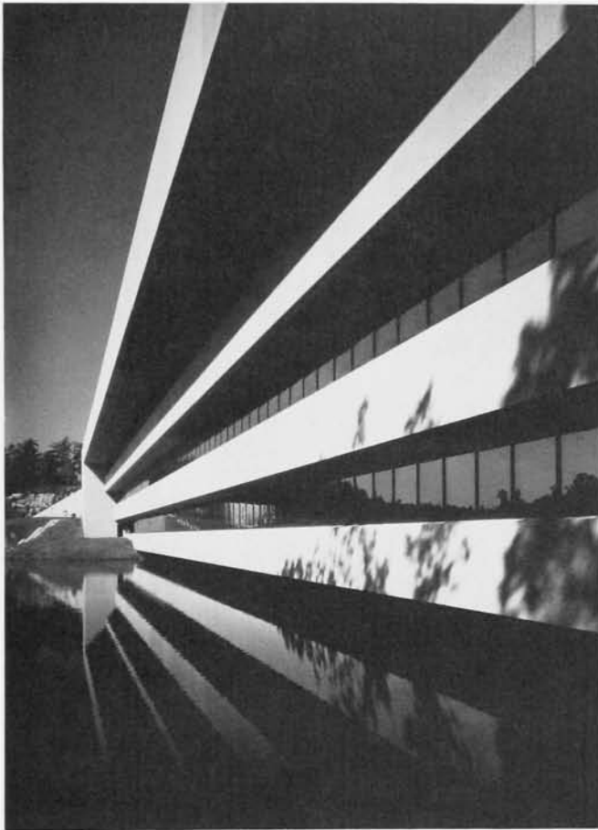
Cantilevered Floors over Pond
