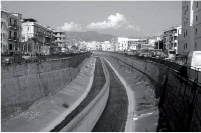
Figure 1. The Calopinace river (Calabria, Italy). An example of full artificialization (photo A. Goltara).
