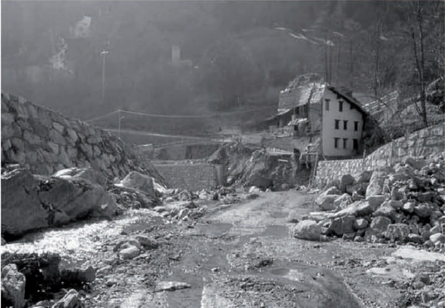
Figure 2. T. Lys (Gressoney, Italy), after the flood of 2002. Huge protection works along the banks are apparent, as is the dangerous proximity of the house to this aggressive water course (photo A. Goltara).
