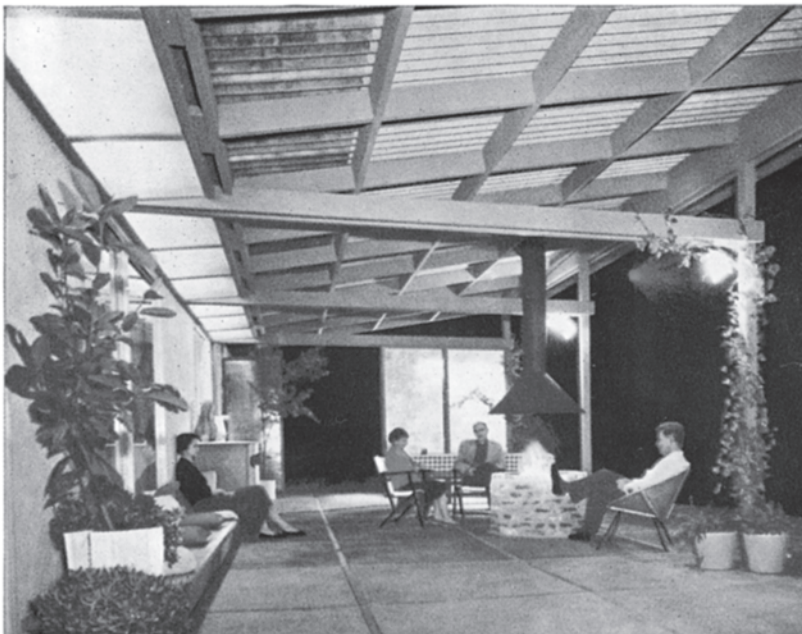
Strategically placed lights glamorize room at night as guests sit around fire in "wishing well" grill
