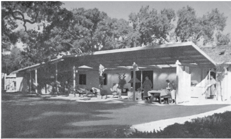
Jaunty roof of the outdoor room was designed to let in more light; it protects grill, tables, even the TV
