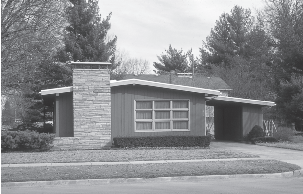
An ordinary postwar house, Urbana, Illinois. Date and architect unknown. Note the picture window and the storage wall that supports the shed roof of the carport. Photograph by the author.
