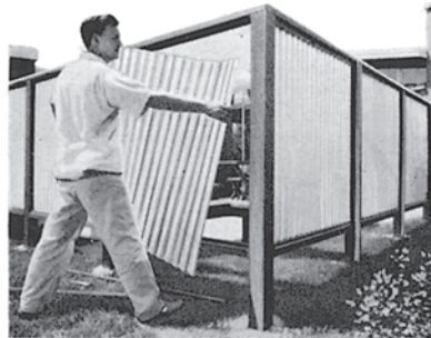
Lightweight inserts of corrugated aluminum make a modern patio enclosure that requires no painting
