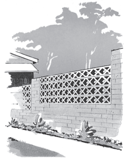
Attractive masonry wall combines regular 4-in. concrete building blocks with ornamental criss-cross ones Courtesy National Concrete Masonry Association
