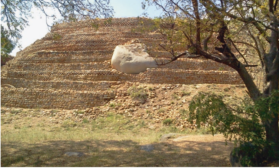
Fig. 9.3 The restored western terraces at the Hill Complex. Photo by S. Makuvaza, April 2016
