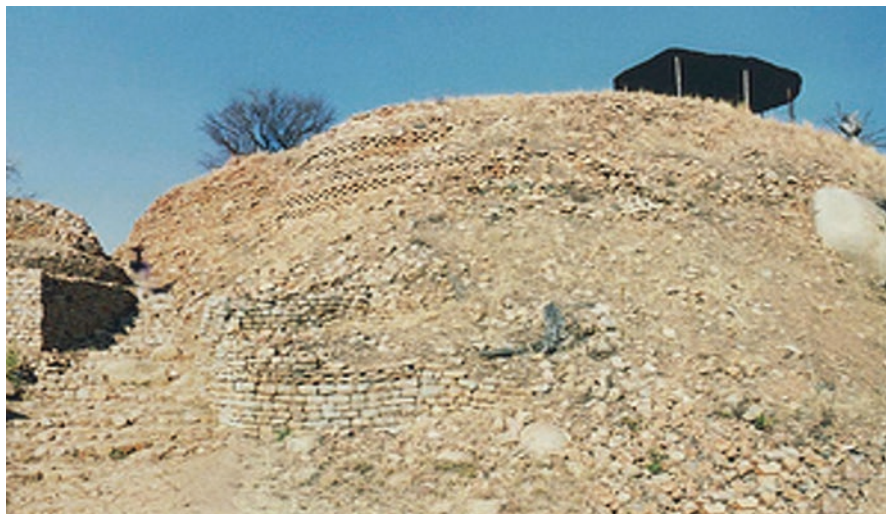
Fig. 9.2 The western terraces of the Khami Hill Complex before restoration in 1999. Photo by S. Makuva
