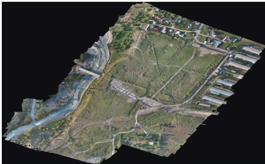
Fig. 6.8 Site of Talgar during the construction of the four-lane road “Birlik-Almalyk-Kazstroy-Ryskulov-Ak-Bulak”. Component part of the Silk Roads: the Routes Network of Chang’an-Tianshan Corridor, World Heritage serial transnational property. Detailed high-resolution aero orthophoto mosaic made with UAV, 2015. Copyright: Archaeological Expertise LLP
