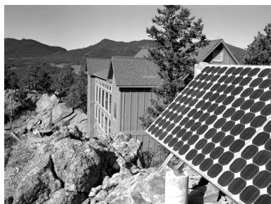
FIGURE 4.1 PV array located adjacent to residential building.
