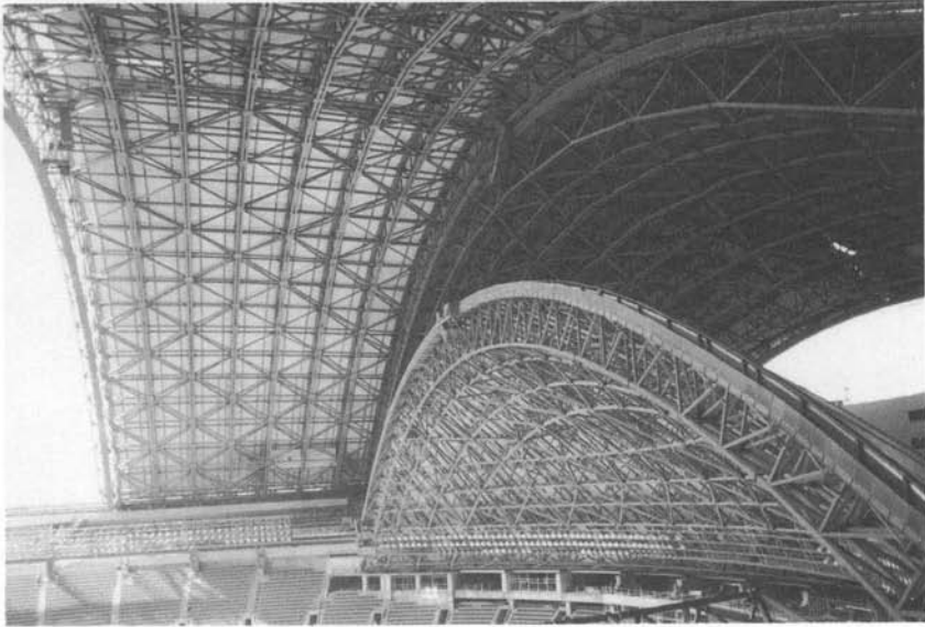
(a) Roof structure of the SkyDome, Toronto, Ontario
