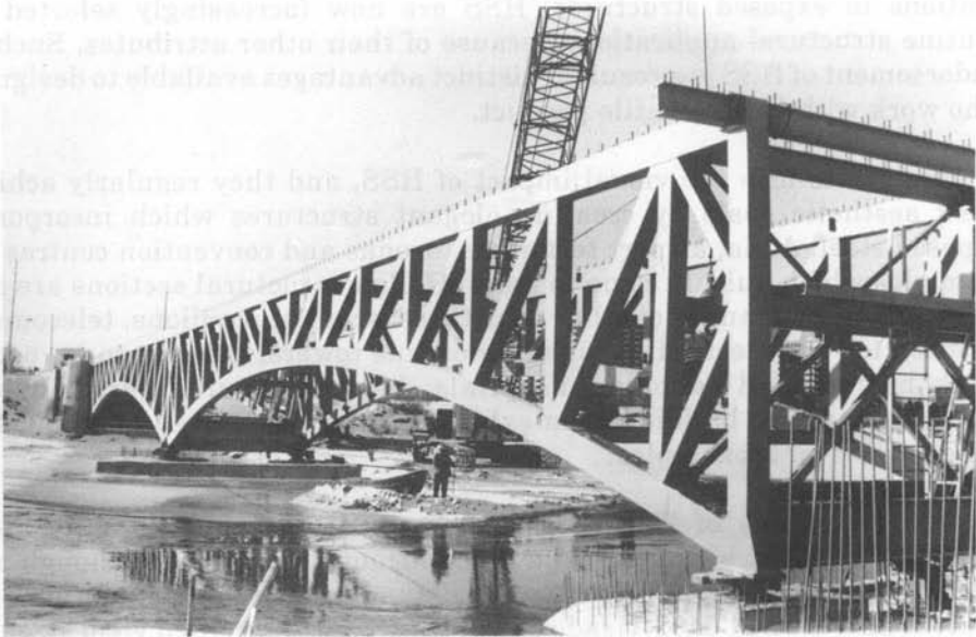
(b) HSS bridge under construction
