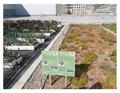
Fig. 34 The biotope-type planters (left side) and the green roof vegetation (Credit: Joe Nasr)
