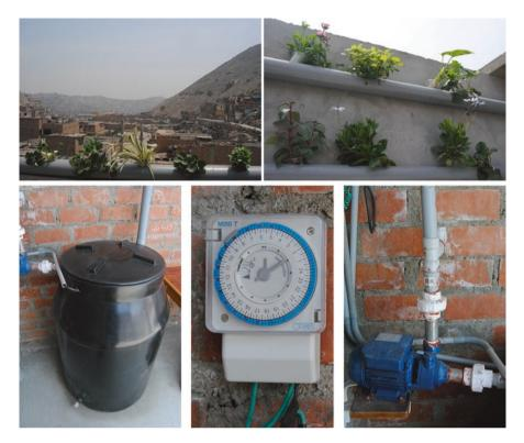
Fig. 2 Modified NFT system that works with a pump in the children playhouse at Monterrey, Lima, Peru (Photo: F. Orsini). *Top*, views of the hydroponic gardens, *bottom*, *left* to *right*, tank for the nutrient solution, electric timer and hydraulic pump
