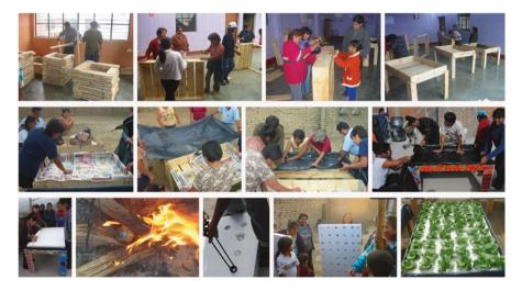
**Fig. 5** Step-by-step procedure for building up a simplified floating system. *Top row*, construction of the growing table. *Middle row*, insulation and waterproofing with a black PE film. *Bottom row*, preparation of the styrofoam trays by making holes with a hot iron rod. Images from Lima and Trujillo, Peru (Photo: F. Orsini)
