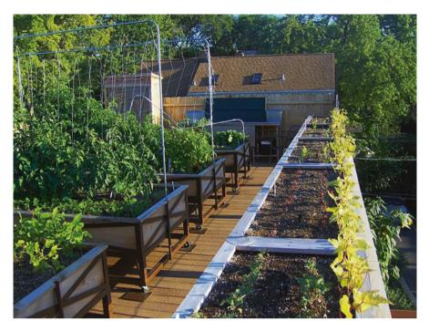
Fig. 2 Planters on the Uncommon Ground roof in Chicago are used as barriers for safety on the roof. (Photo: M. Cameron)
