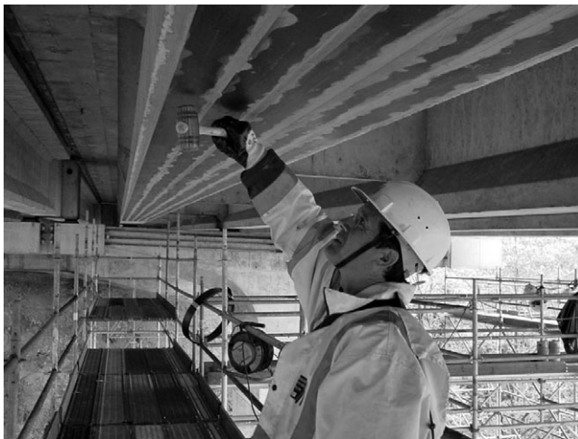
20.1 Inspection with acoustic sounding (hammer tapping).
