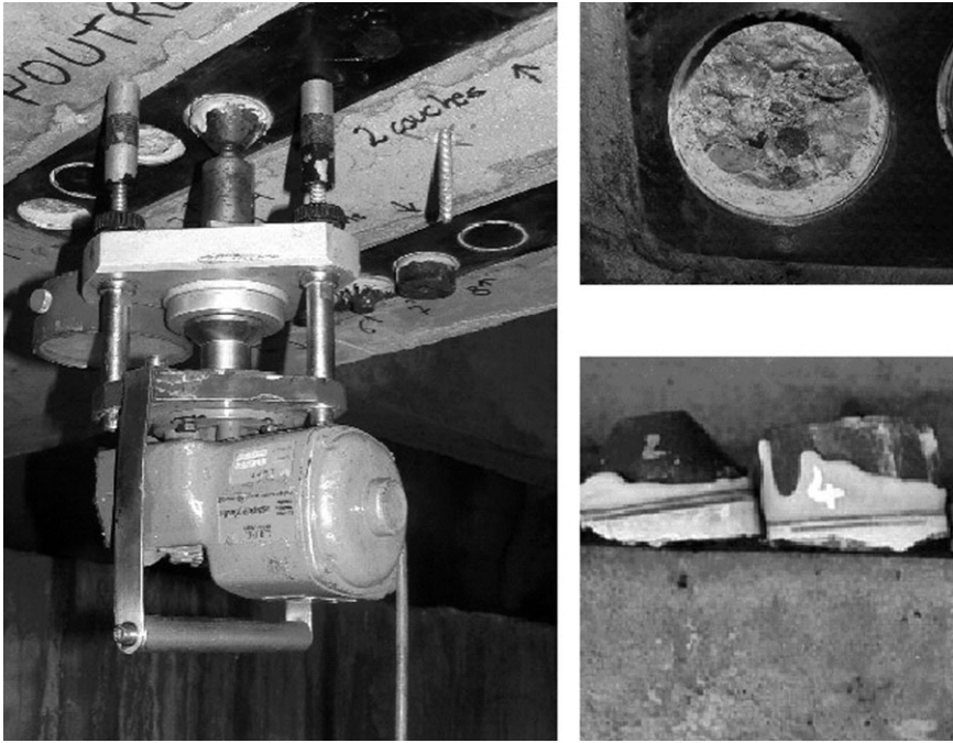
20.2 In-place pull-off method.
