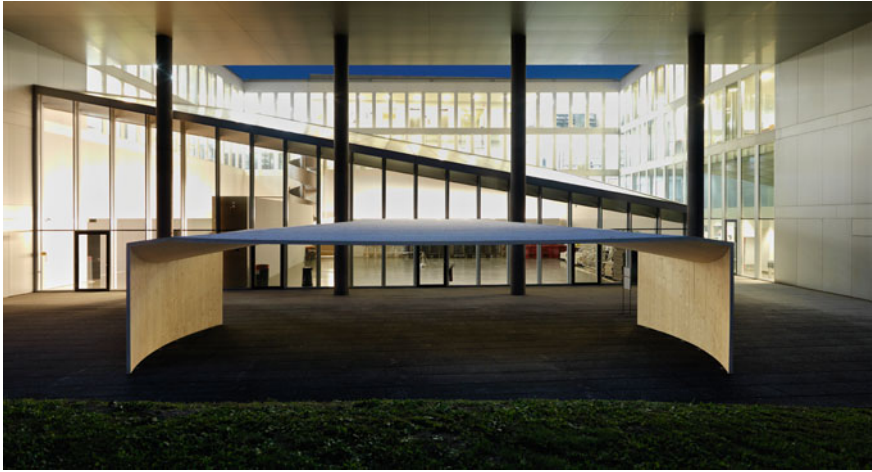
Fig. 1 Full-scale, mono-material prototype structure, spanning 13.5 m at a shell thickness of 77 mm, exhibited at the academy of architecture in Mendrisio, Switzerland
