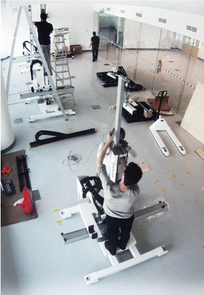
Fig. 4 A simple pulley is used for installation and height adjustments; the vertical axis is modularized into five segments (Gramazio and Kohler, FCL Singapore, 2012)
