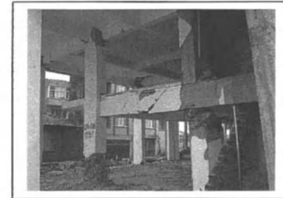
*Photo 6. Compression failure in RC column. irregular Building.*
