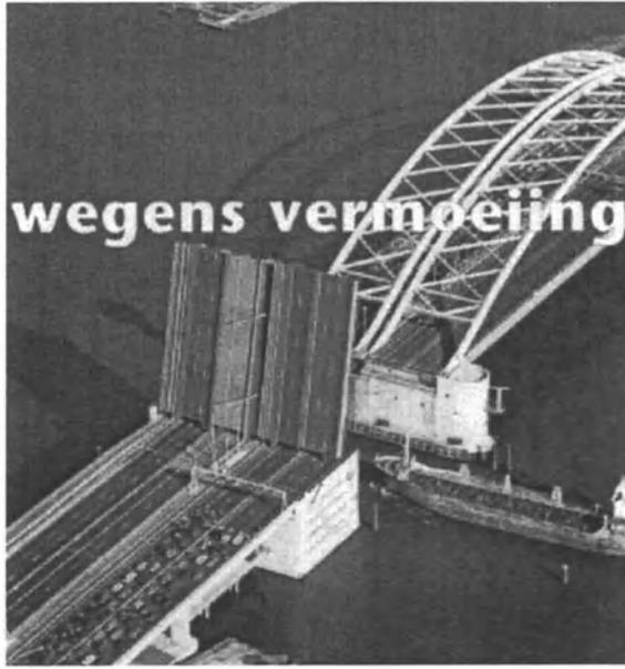
*Figure 1. The two Van Brienenoord Bridges in the main highway North-South near Rotterdam. The wording **wegens vermoeiing** means because of fatigue. The deck of one of the two bridges was replaced because of fatigue damage in the deck structure.*
