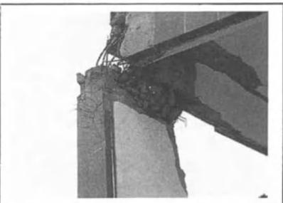
*Photo 5. Beam-to-column joint failure.*
