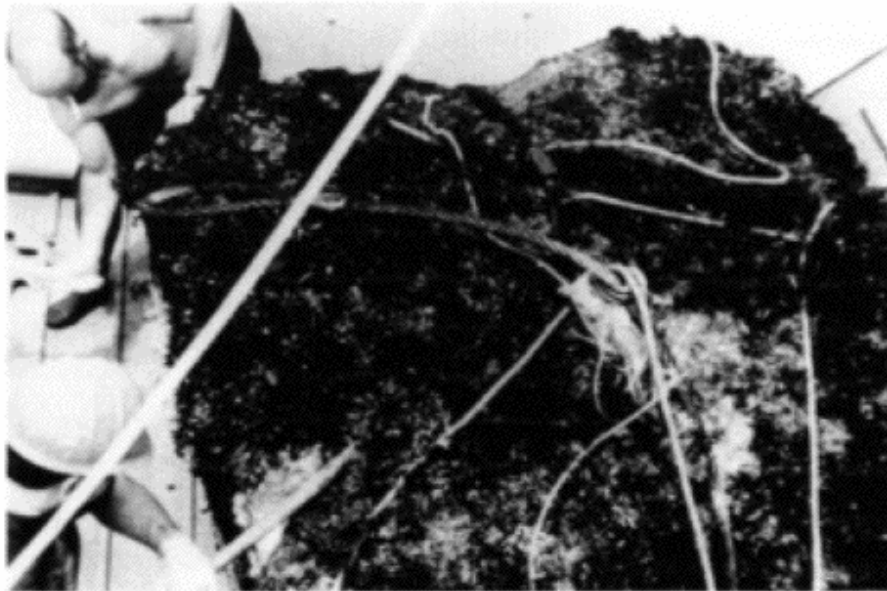
Fig. 4.1. Marine growth on lean concrete block exposed to seawater for 67 years (reproduced, with permission, from Ref. 10).
