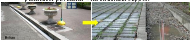
Fig.23: The original side drains different with new swales on the side could conserve water
