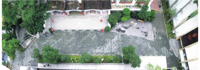
Fig.10:The permeable pavement in front of Design department building panoramic view
