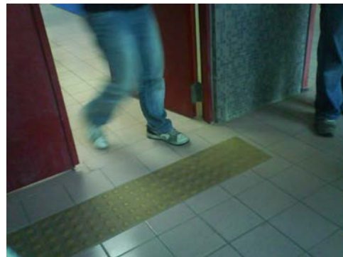
Fig. 1 Tactile paving built by rubber
