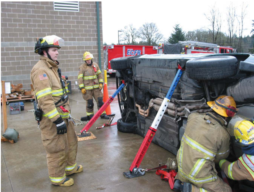
Figure 11-4. Emergency struts are often grouped to provide better rigidity and support.
