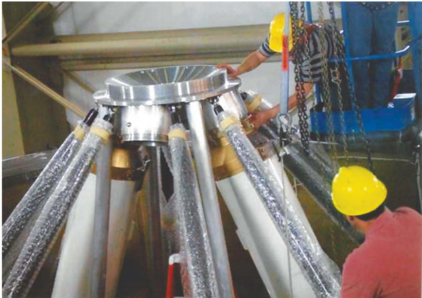
Figure 7-5. Installation, assembly, and alignment of the motors into the motor-mount cage of the MLAS vehicle. (Courtesy NASA)
