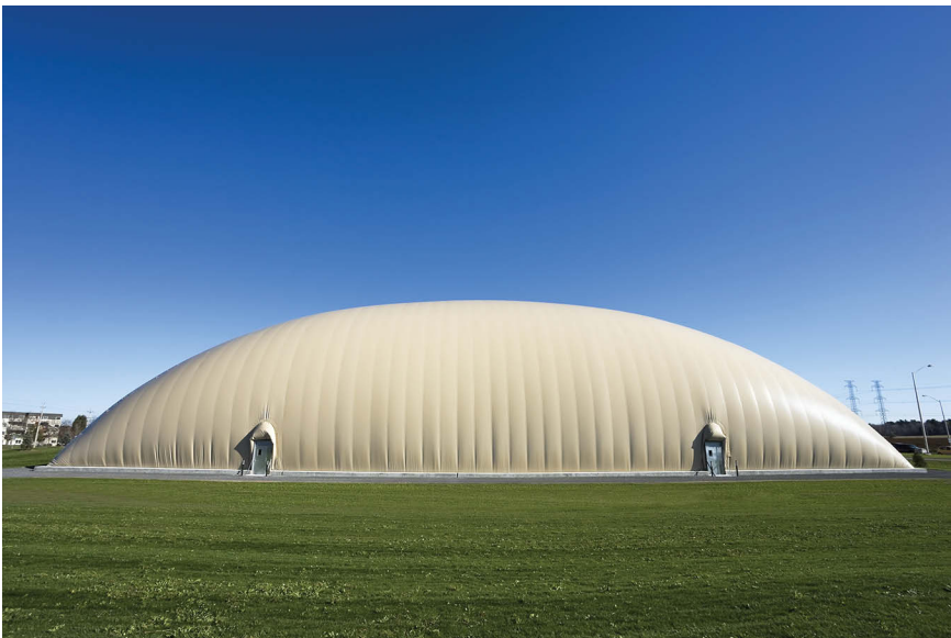
Figure 10-6. A large, inflatable, air-transportable manufacturing facility.
