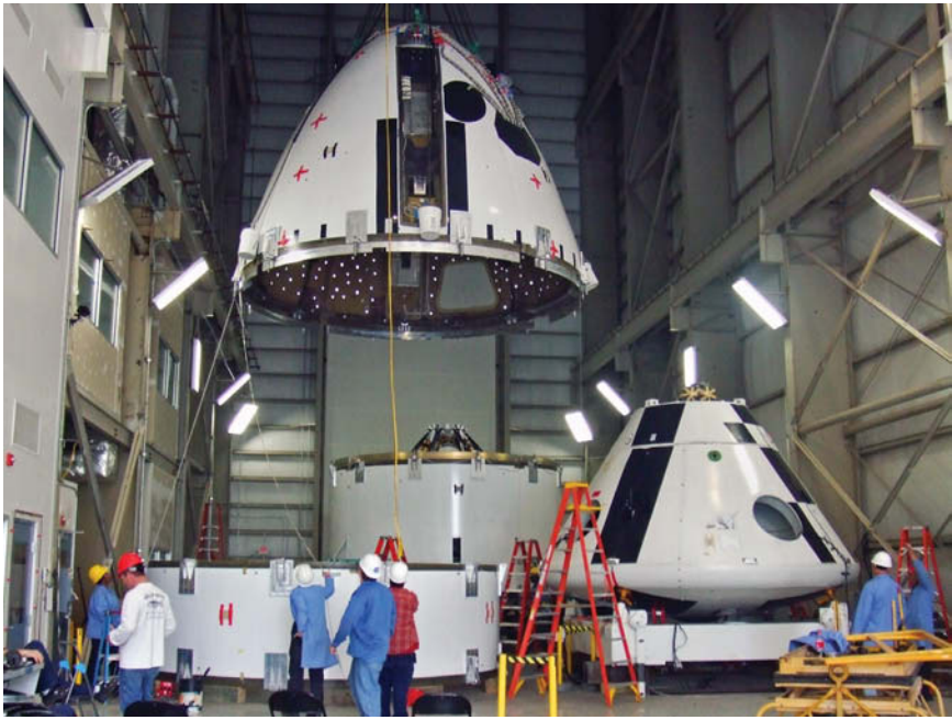
Figure 8-3. Forward fairing assembly using straps and crane to position onto MLAS vehicle. (Courtesy NASA)
