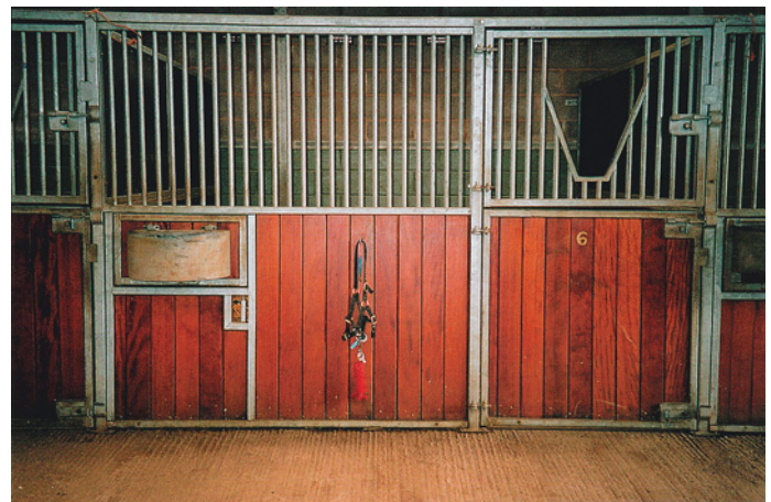
Fig. 8.1 Front of stable. Note the weaving bars, the bolts on the top and bottom of the door and the kick bolt at the bottom. The stable has its own number for identification, an individual head collar for the patient and a removable manger that can be given to the horse without the need to enter the stable.
